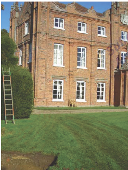
Figure 7. Location of Pump 2, near east range of house
