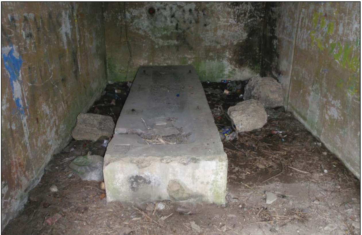
Building 62, interior showing machine bed for the generator (camera facing north)
