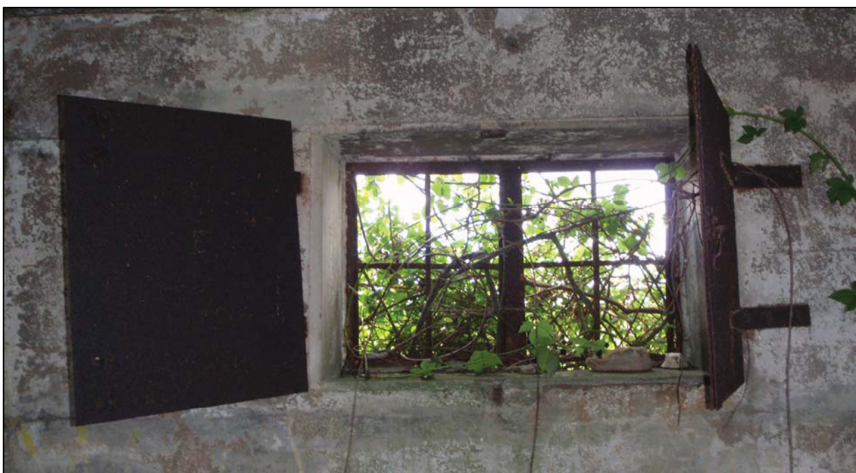
Building 64, window with steel shutters and metal frame (camera facing west)
