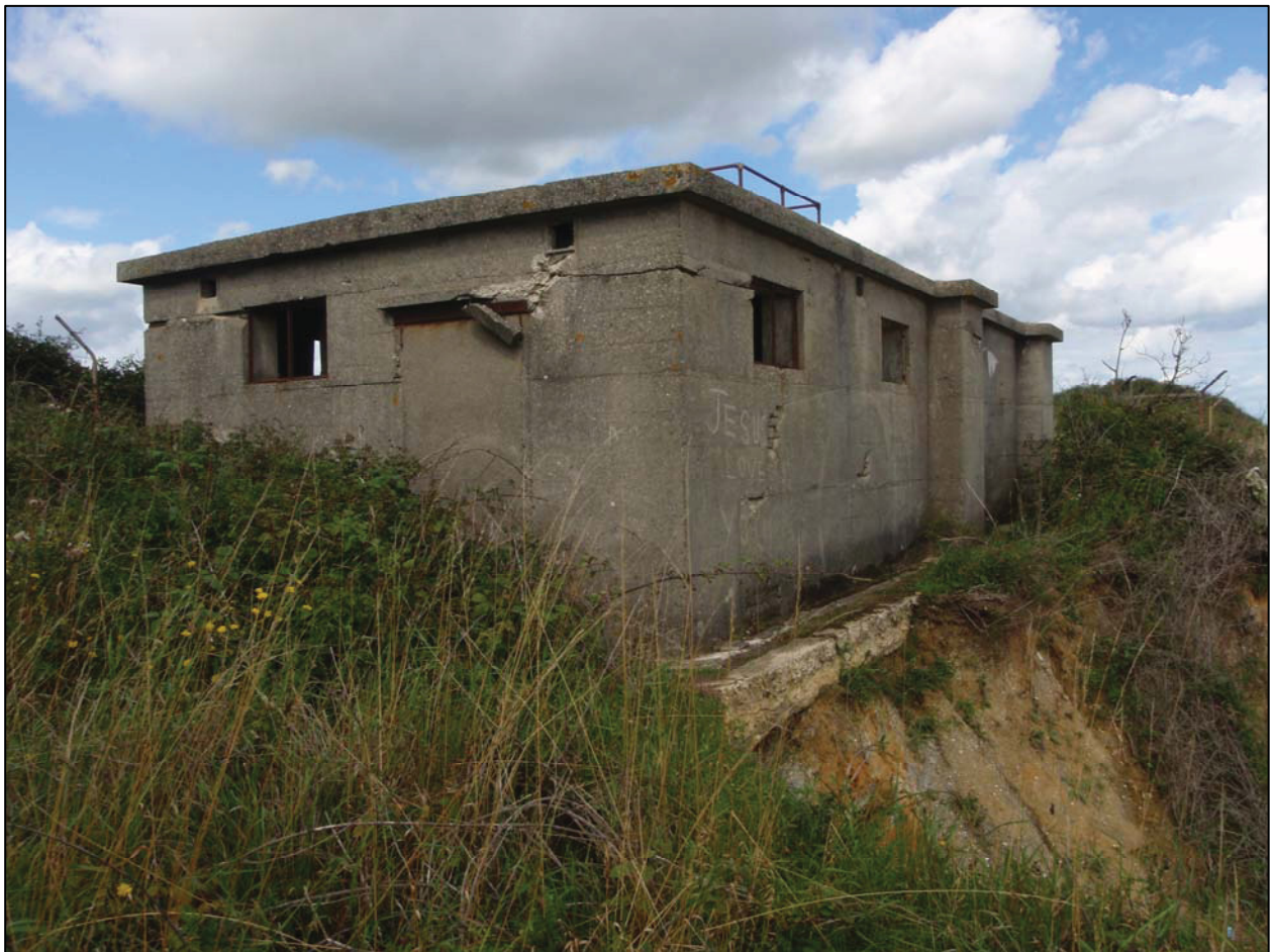
Building 64 showing the blocked southern door and the erosion undermining the southeast corner (camera facing northwest)
