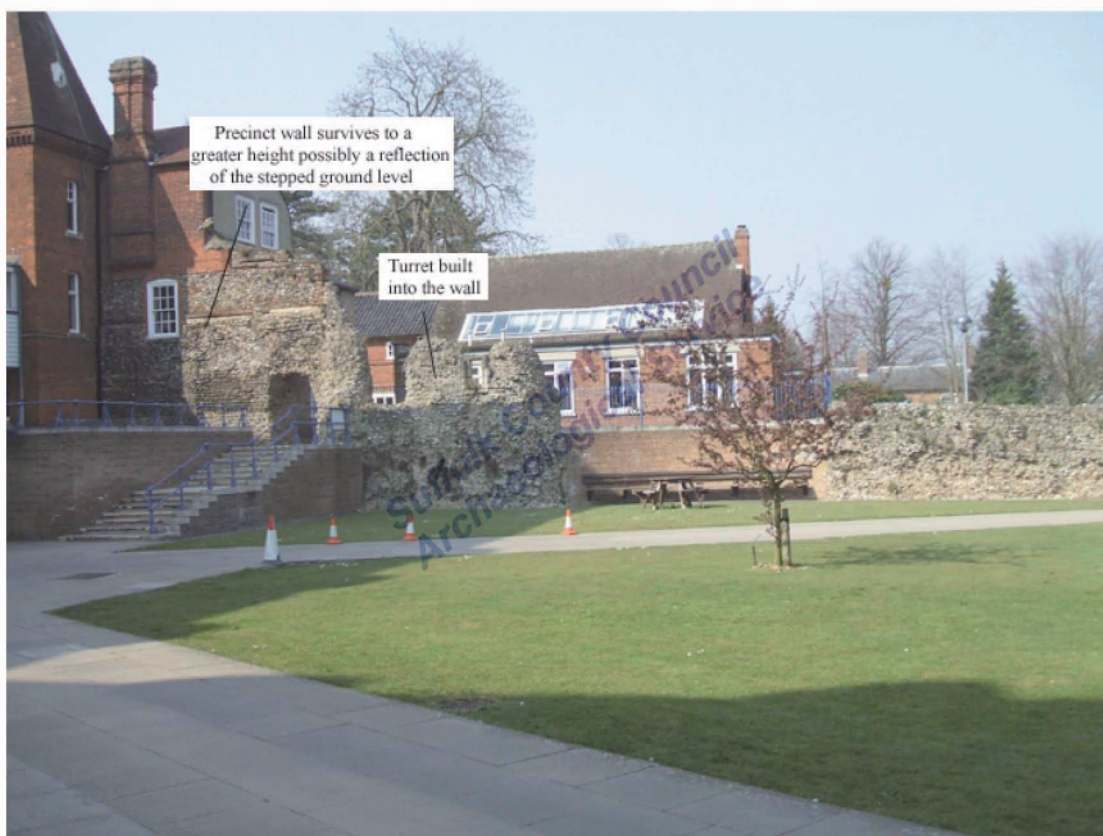
Figure 2. 'B' turret within precinct wall
