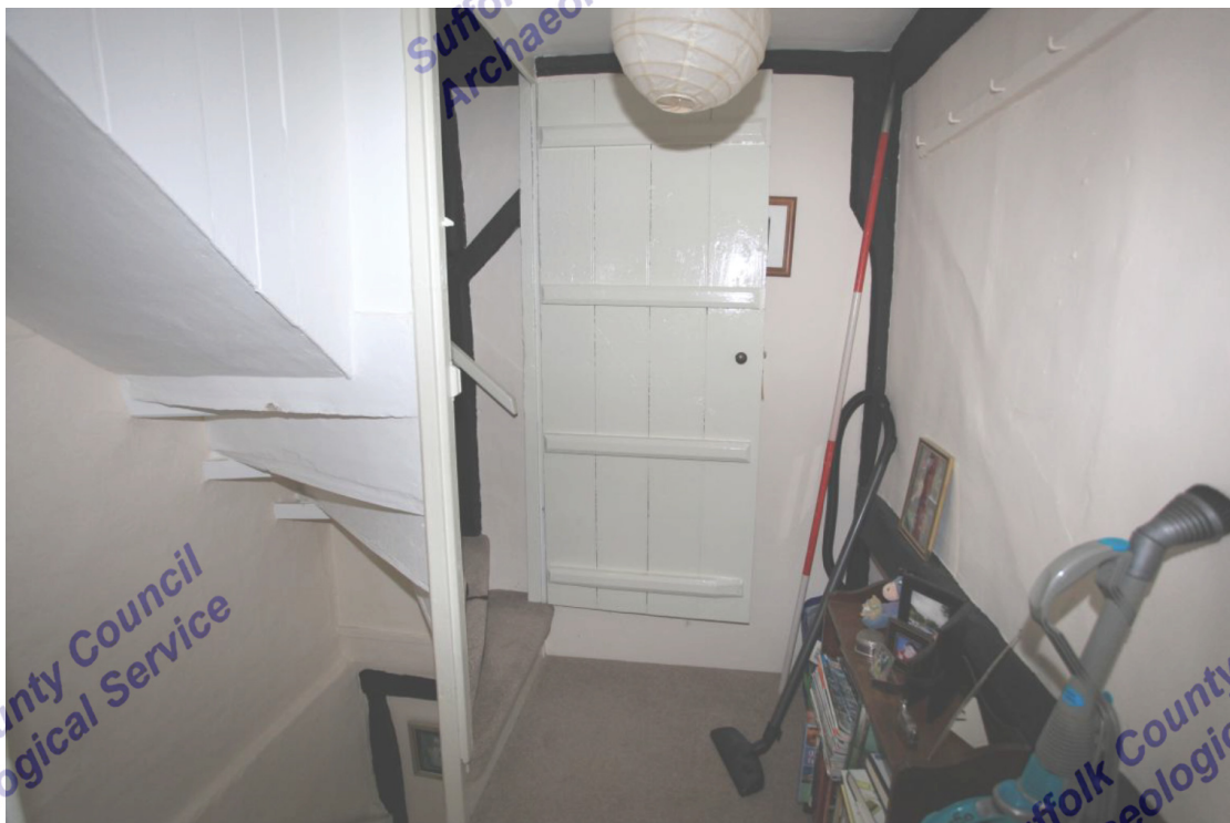
Illus. 8. Stair landing of no. 1 (5) from west showing door to attic stair with blocked access door to no. 2 in centre. The original roof-plate is visible to the right with the contours of the studs and brace of the second-phase wall visible in the render above.
