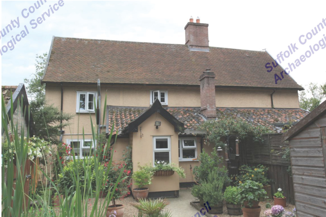
Illus. 3. Northern external rear elevation from garden of no. 2 showing panelled roughcast pargeting with 20 th century lean-to kitchen extensions and detached brick shed dated 1875 to left.
