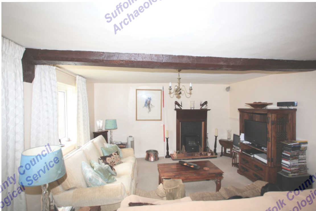
Illus. 4. Living room of no 2 from east showing 20th century fireplace and chamfered binding joist (2) spanning width of 17 th century hall. Much of the 17 th century fabric, including an 'inglenook' fireplace, is hidden behind modern render.
