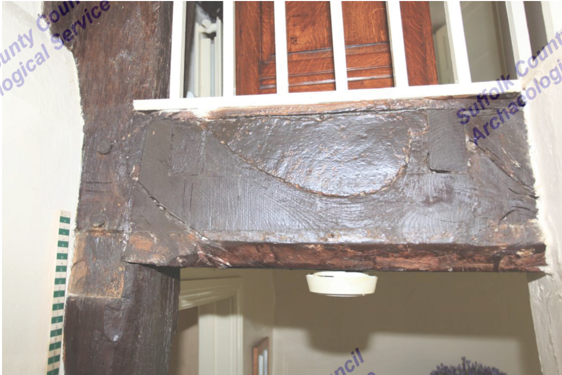
Illus. 5. Detail from west of chamfered binding joist above stair in living room of no. 2 showing carpenters' numerals and the mortises of the tall-sectioned common joists that were removed to accommodate the stair. The original joists probably survive elsewhere but are hidden by render.
