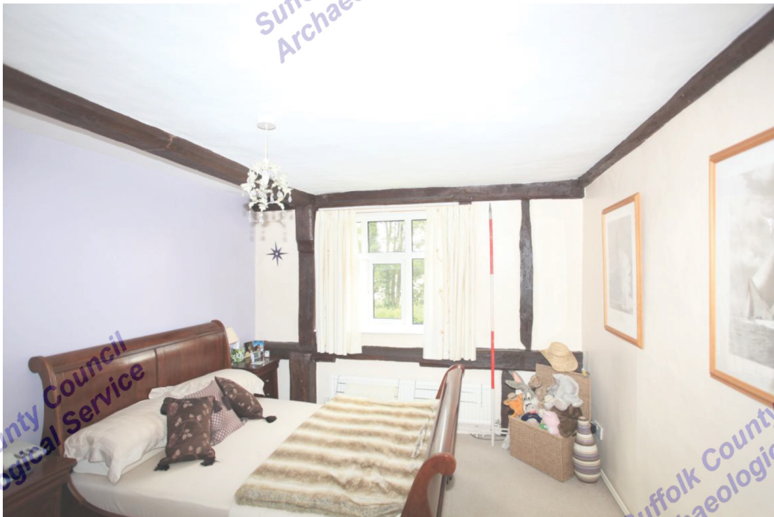
Illus. 6. Southern interior of western bedroom (9) in no. 2 showing the original roof-plate below the window with the mid-17 th century heightening of the wall above.
