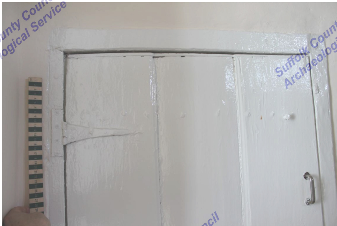
Illus. 9. Detail of 17th century moulded plank door and hinge to under-stair cupboard in lobby entrance of no. 1 (4).
