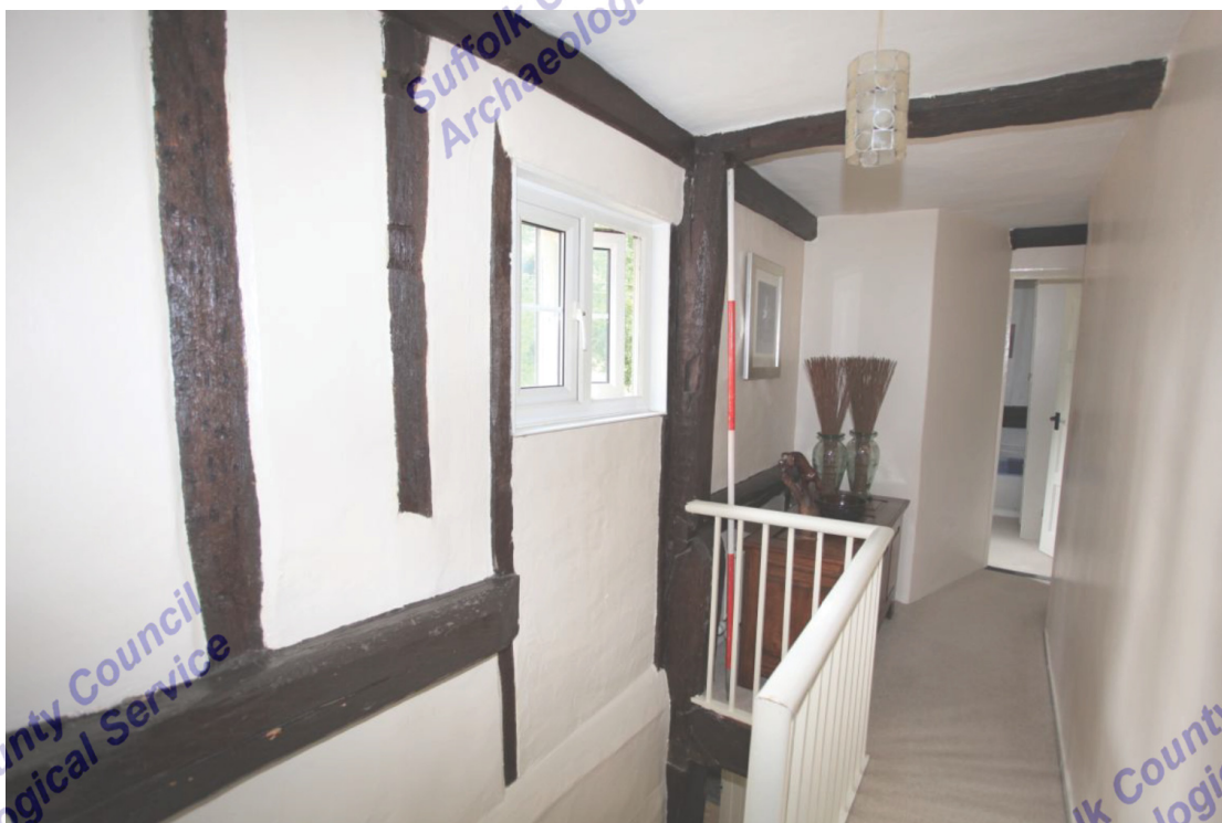
Illus. 10. Stair landing (8) of no. 2 from west showing original rear (northern) roof-plate below with raised wall above. The former has been cut to insert an external loading door of a kind often found in 18 th and 19 th century farmhouses.
