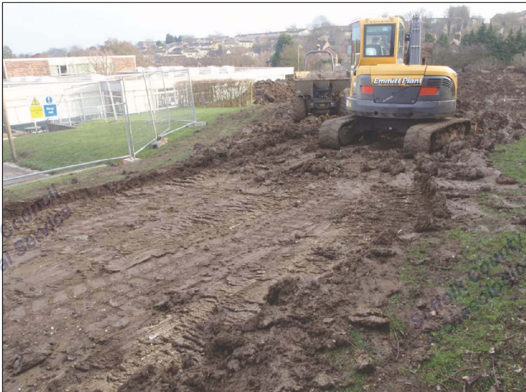
Plate II: Stripping the Haul road, looking SE (photo ref. GEW 30)
