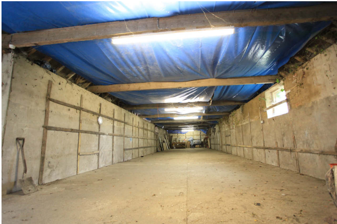
Illus. 6. Interior of linear barn (1) from east showing door to central yard (7) to extreme left and northern window to right. The internal walls have been cement rendered to operate as a loose grain store and the roof structure hidden by a tarpaulin to trap falling dirt and debris.
