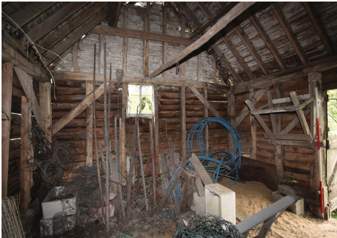
Illus. 10. Interior of unusually diminutive western shed (4) from east showing arch-braced tie-beam and roof-plates with central tenoned post.
