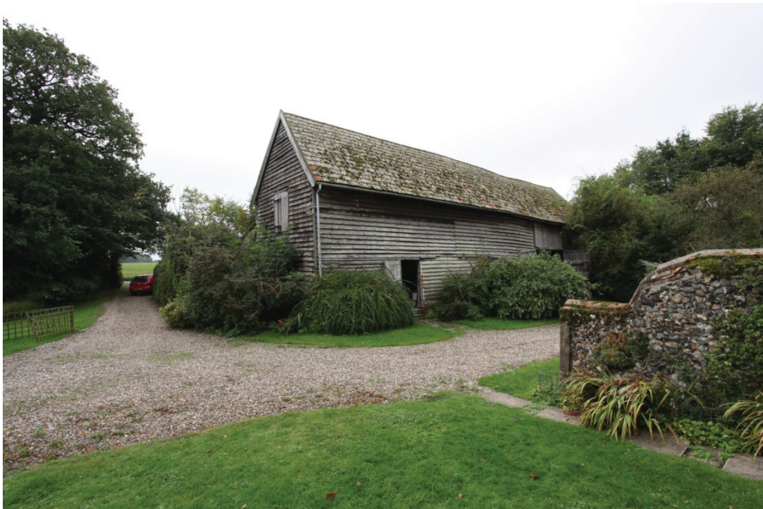
Illus. 2. Northern exterior of barn (3) from north-east showing yard wall adjoining shelter-shed (1) to right. This elevation of the barn was originally open-arcaded and may have formed a rare hay-house
