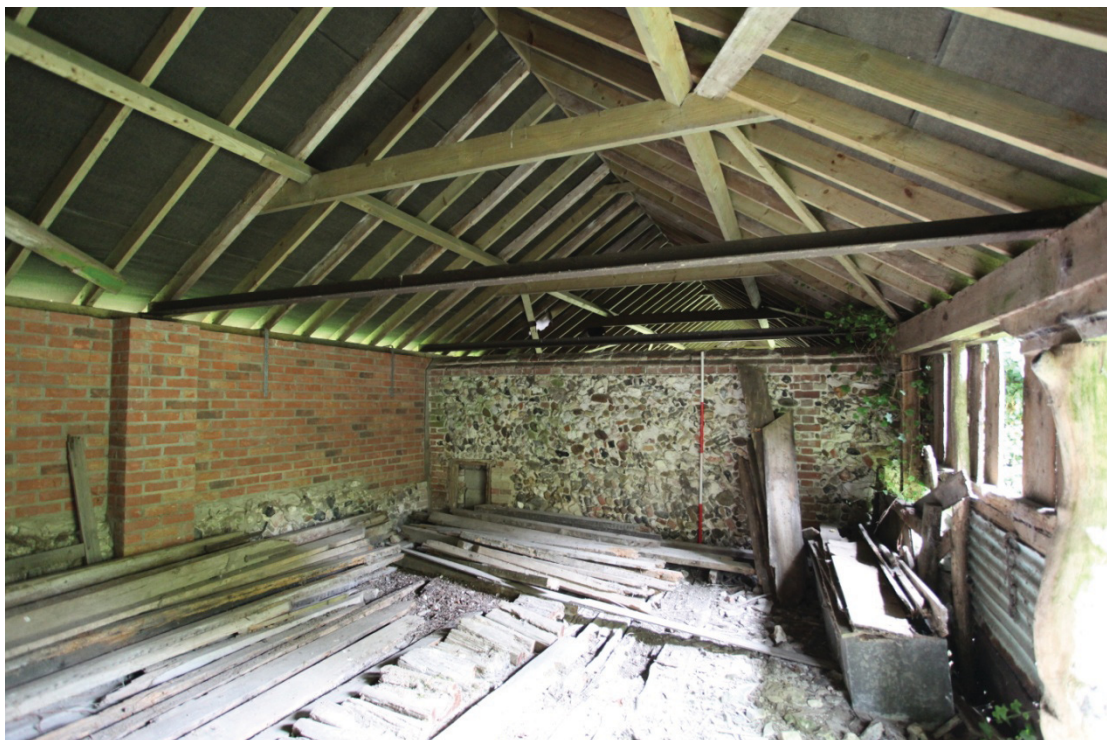
Illus. 8. Interior of western section of shelter-shed (1b) from west showing rebuilt northern elevation to left, open arcade adjoining southern yard to right and flint-rubble partition against the eastern section in centre. The small, blocked hatch or calf creep is visible to the left of this partition.
