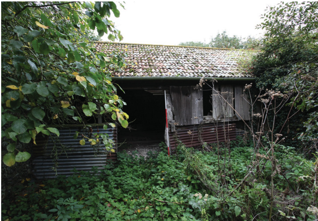
Illus. 4. Southern exterior of western section of shelter shed (1b) from western yard showing 20th century corrugated iron loose box (1a).
