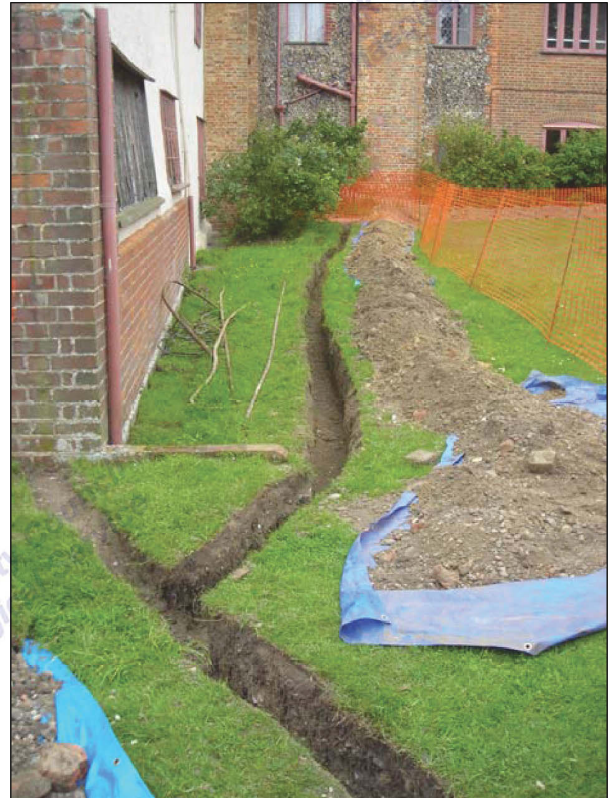
Plate 1. General view of the trench under excavation. Located within the church nave, looking west.
