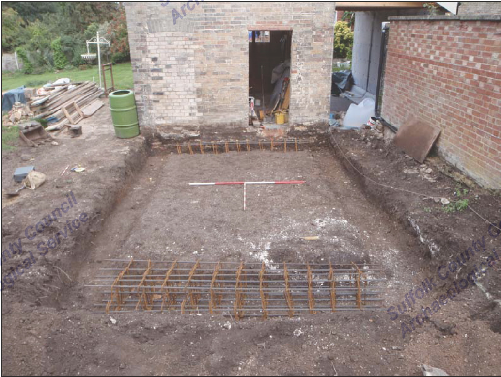
Plate 2. Extension footings, facing north
