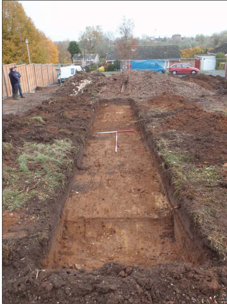
Plate 1. Trench 1, facing north
