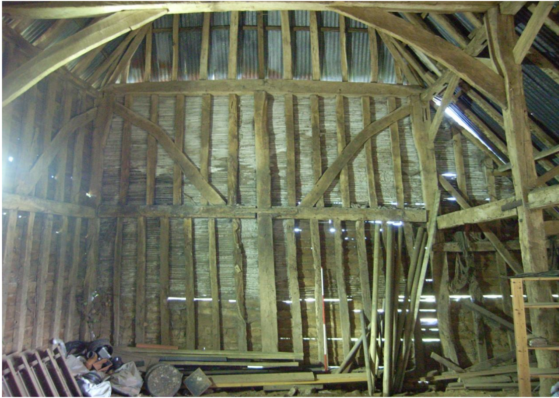
Illus. 7. Barn (1). Interior of northern gable showing original close-studding and internal bracing. This, and the two northern bays of the western elevation visible to the left, represents the only intact 16 th century studwork in the barn. Mortises for the missing studs of the eastern elevation (removed when the aisle was added in the 17 th century) can be seen in the roof-plate and mid-rail to the right.
