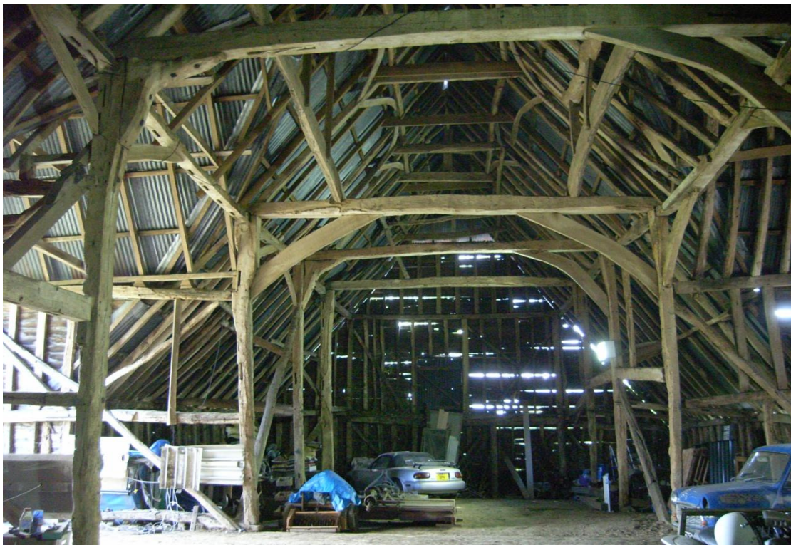
Illus. 8. Barn (1). General view of interior from north showing the original porch to right and the secondary porch & aisle to left.
