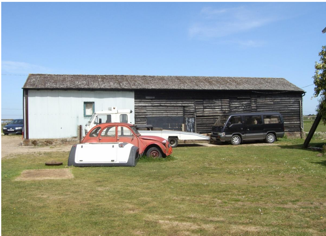
Illus. 12. Southern exterior of the rare but well-disguised early-17 th century stable (2) seen from the yard and showing the late-18 th or 19 th century extension behind modern corrugated cladding to the left.
