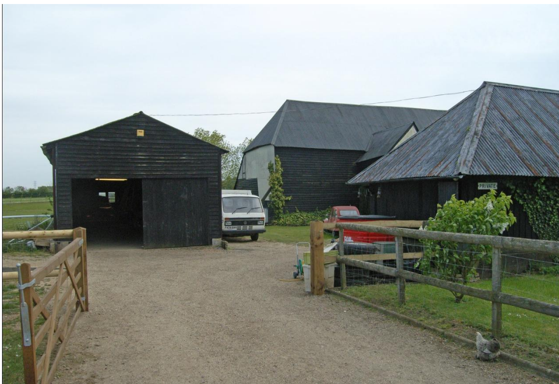
Illus. 2. Modern equivalent of 1898 painting showing stable (2) with replaced roof of reduced pitch to left to left with the barn (1) and shelter-shed (3) to right.
