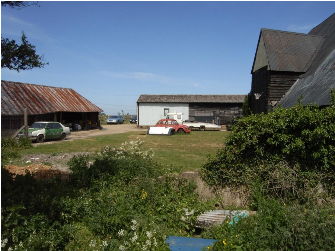
Illus. 4. Farm yard from south showing the late-16 th century barn (1) to right, the early-17 th century stable (2) in centre rear and 19 th century shelter-shed (3) to left.
