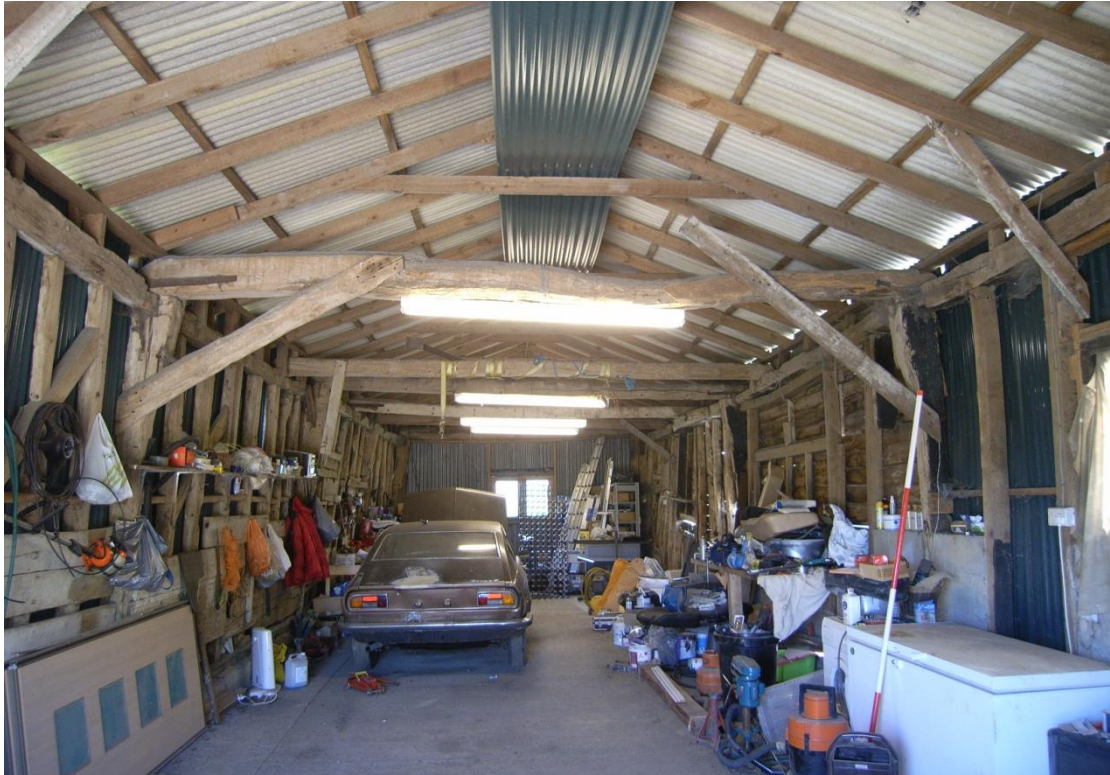
Illus. 13. Stable (2). General view of the interior from modern entrance in western gable showing 20th century softwood roof structure with well-preserved 17 th century framing to right and left.
