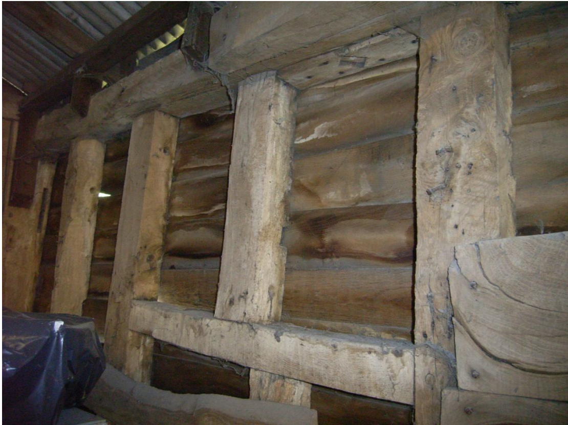
Illus. 15. Stable (2). Detail of secondary diamond-mullion lintel nailed beneath roof-plate in southern interior of eastern bay (immediately above the window lintel shown in illus. 14). This window would have served the missing hay loft
