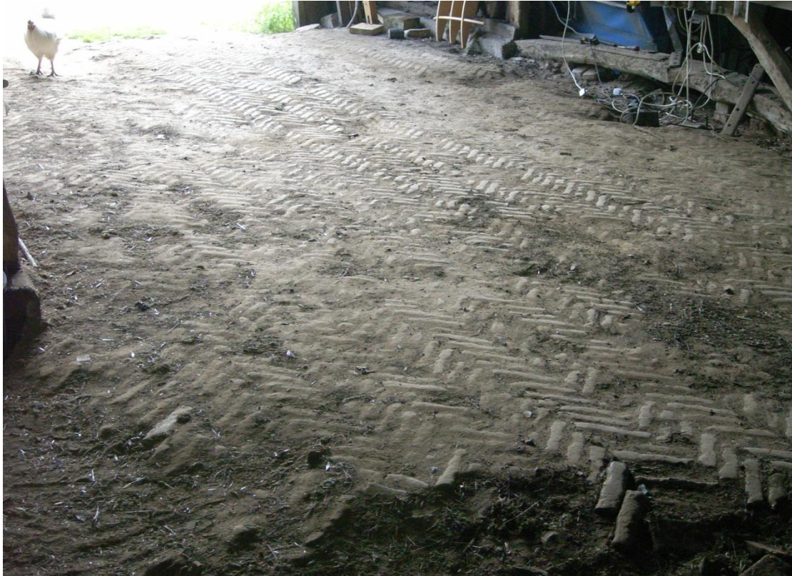
Illus. 11. Barn (1). Detail from east of the good 19 th century threshing floor which extends into both porches. The bricks are laid in a herringbone pattern.
