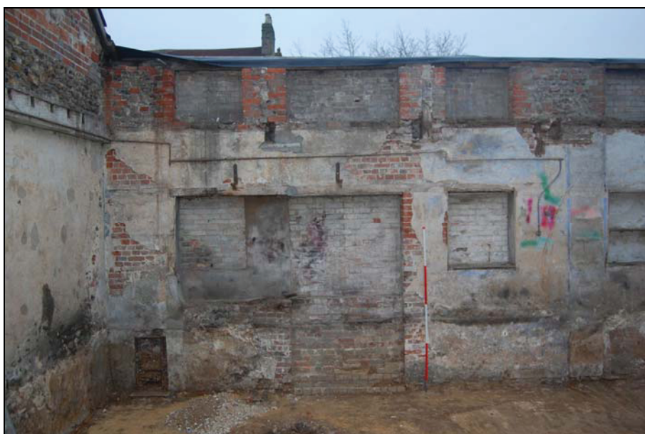
Plate 12. West facing stable wall showing fireplace to the left and bricked in entrance straight ahead. The scale is 2m.
