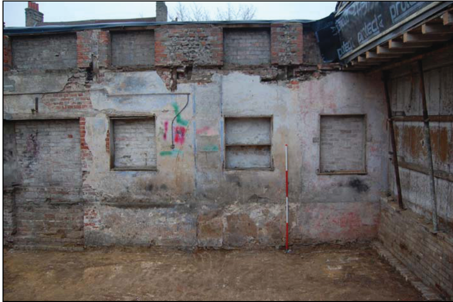
Plate 13. South end of east facing stable wall with bricked in openings prominent and 'watermark' where the floor level was raised. The scale is 2m.
