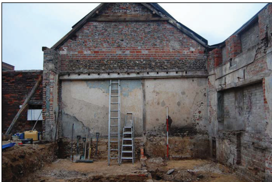
Plate 11. South facing stable wall showing height of the stable block and the collar roof which allowed more space in the hayloft. The scale is 2m.
