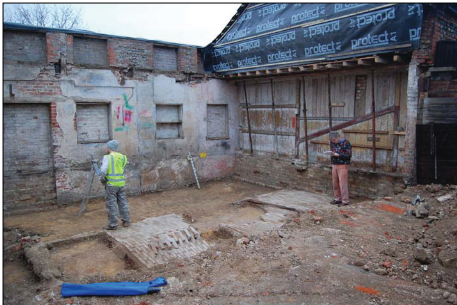
Plate 14. Subdividing south wall of the stable block with bricks to the level of the raised floor and a wooden partition above. The scale is 2m.
