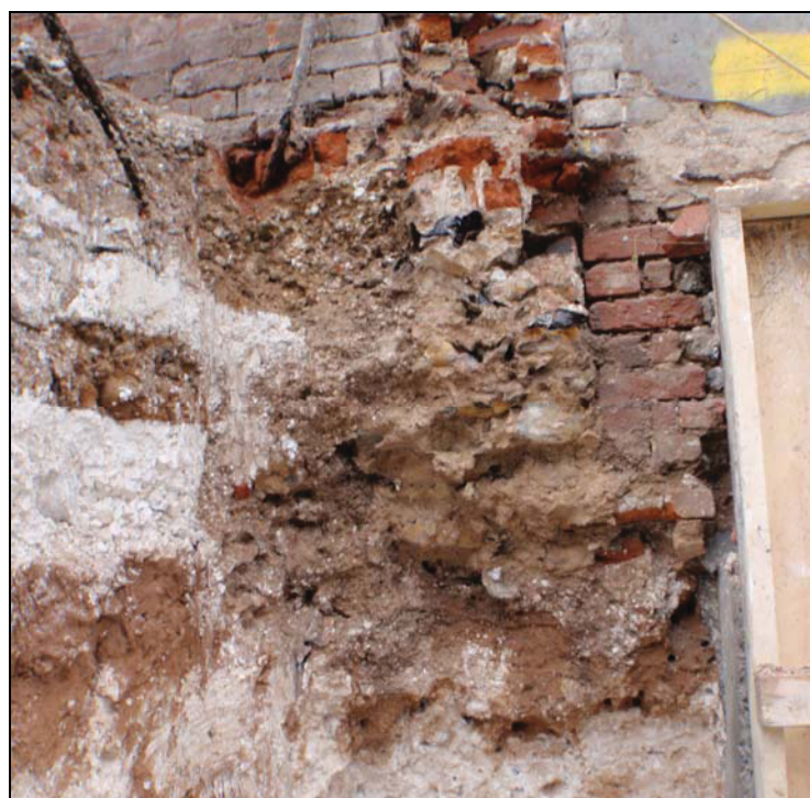
Plate 4. South facing section of wall and the footing trench that was dug into the bank on the north side of the site. The wall perpetuates the line of the original town wall.
