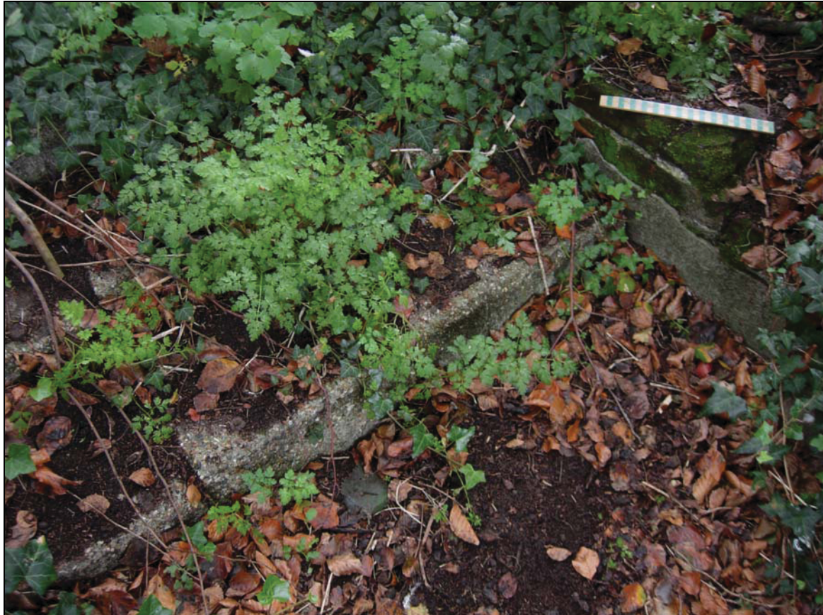
Plate 3. Area 1) Steps and retaining wall
