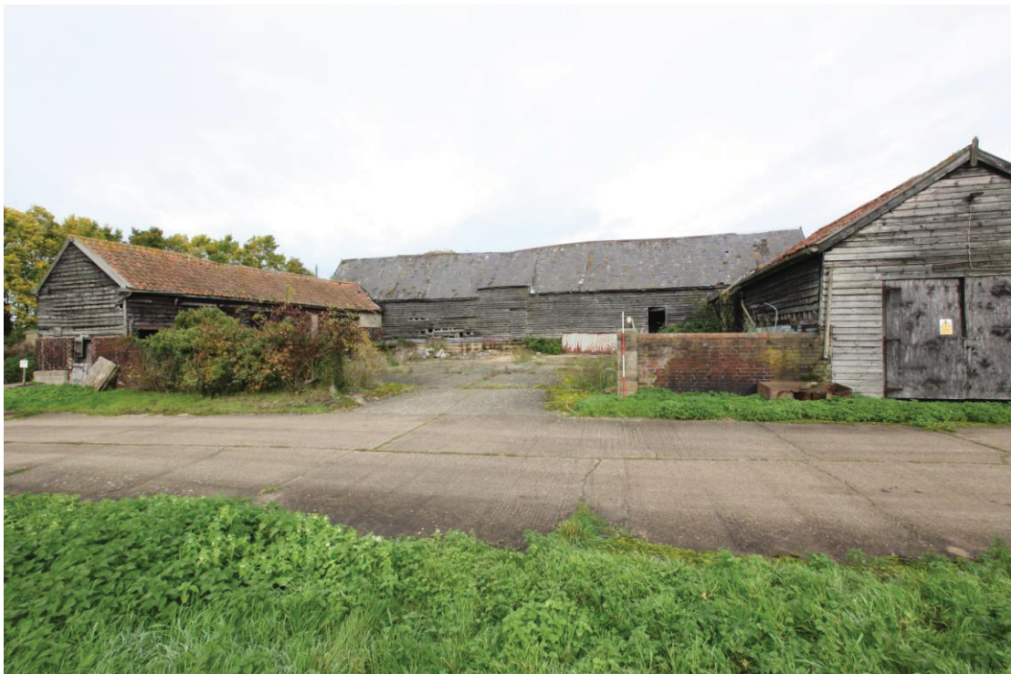
Illus. 2. The farm complex from the south-west, showing the slate-roofed barn and stable (1-3) in rear with the yard sheds (4 & 5) to left and right respectively. The vehicle doors in the gable of the eastern shed (5) are insertions of the 20 th century.
