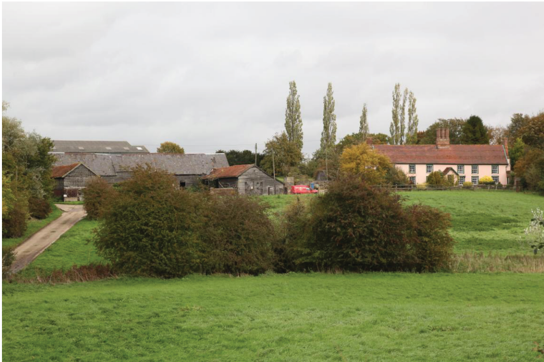
Illus. 1. General view of site from Flowton Road to south showing grade II-listed farmhouse to right and 19 th century barn complex to left.
