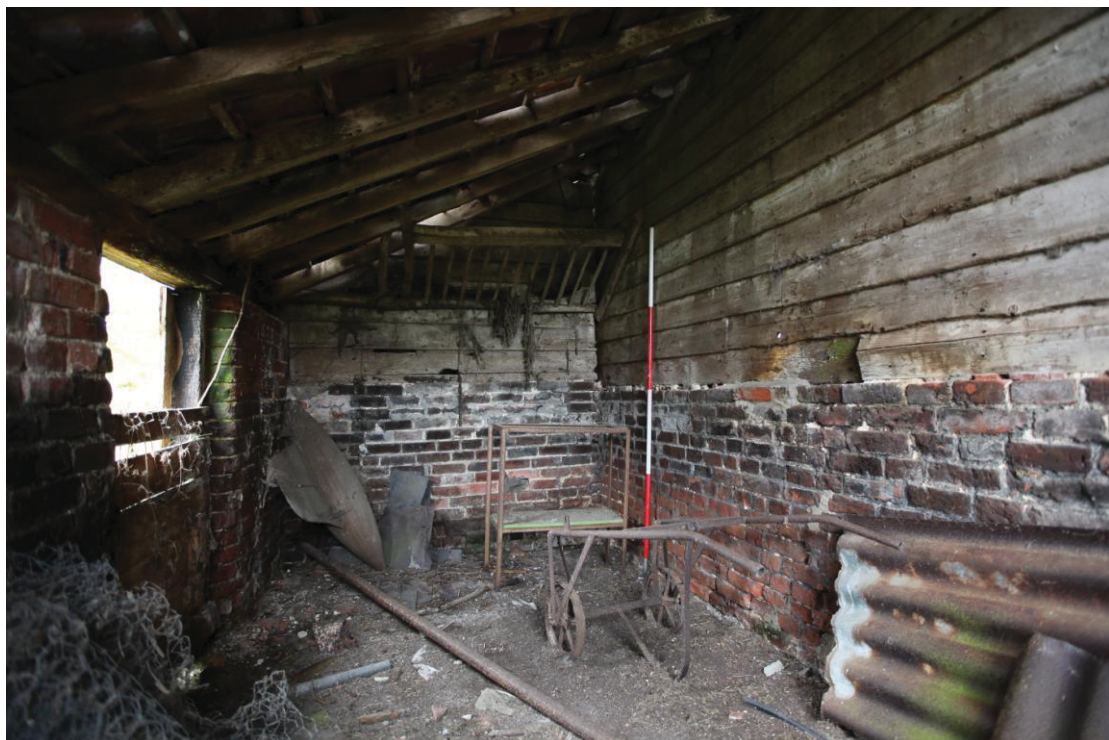
Illus. 12. Interior from north of northern lean-to shed (6a) showing hay rack attached to southern elevation and original entrance to left.
