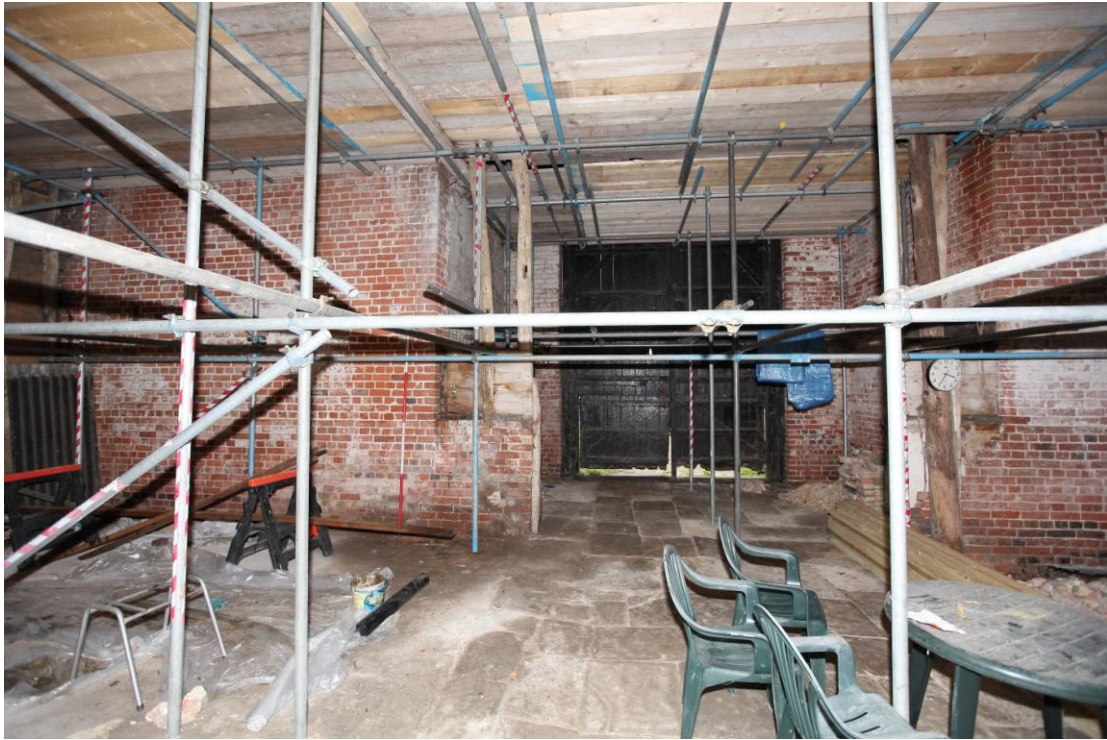
Illus. 9. Northern interior of barn (1) showing its porch with short stub-walls that probably housed grain bins to both sides.
