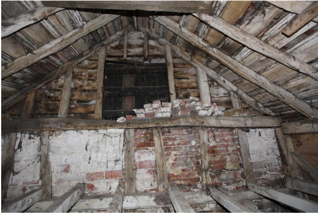
Illus. 11. The southern gable of the hay loft above the stable (2) showing the 17th century tie-beam and studs with later brick infill and hatch.
