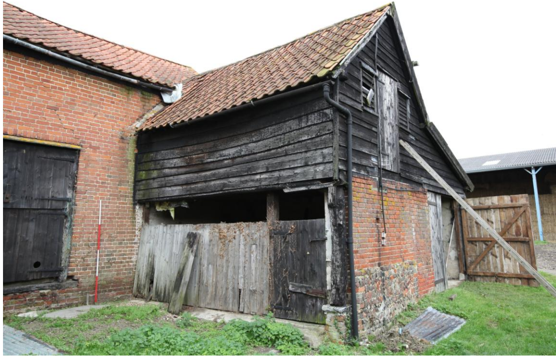
Illus. 5. Exterior of granary wing (3) from south-west showing the open-sided sheltered to the yard on its lower storey with the loading door of the first-floor granary in its southern gable.
