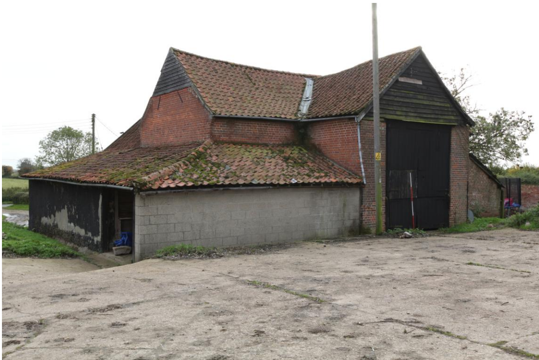
Illus. 2. Exterior of barn from north-east showing the rebuilt cement-block wall of the northern lean-to shed (5) in foreground with the tarred clay-lump wall of the eastern lean-to (4) to the left.
