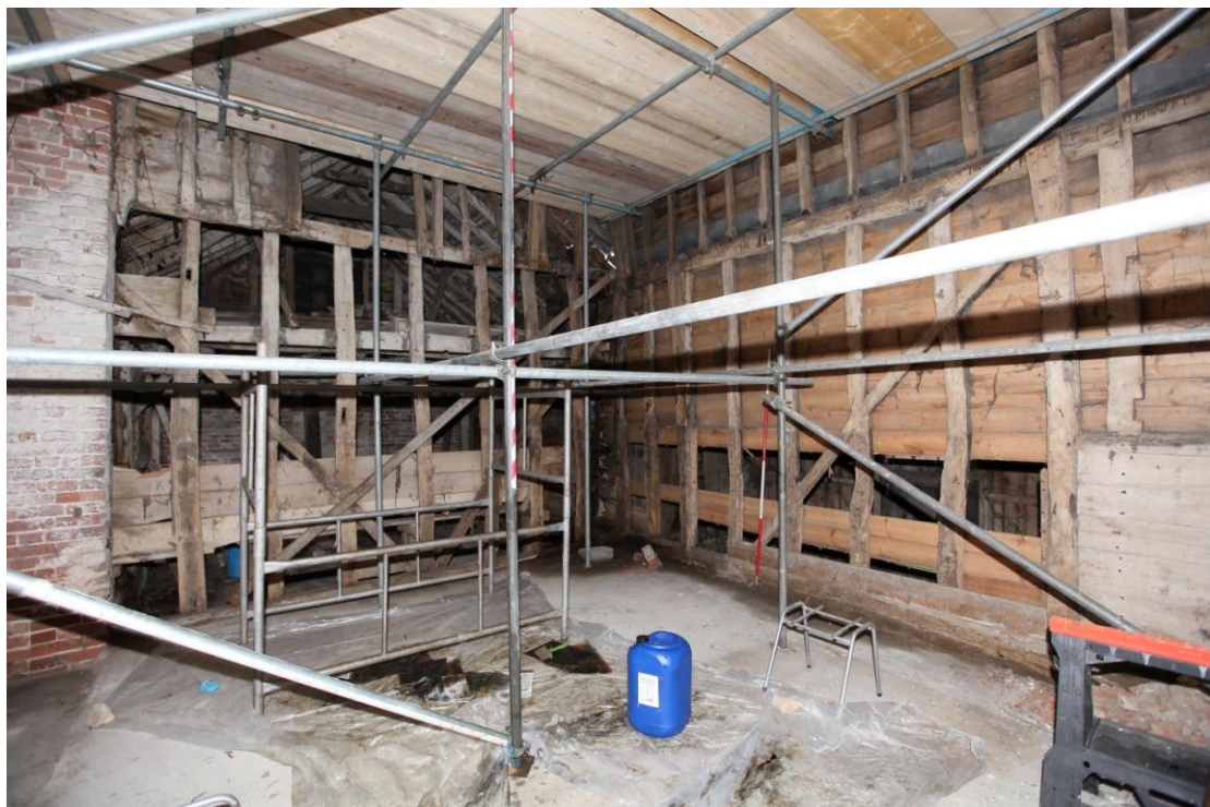
Illus. 8. Internal south-western corner of the barn showing the site of the 17th century structure (1a) with the secondary studwork partition adjoining the stable (2) to the left.
