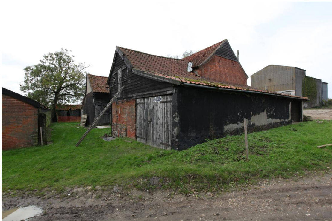
Illus. 6. Exterior from south-east showing the clay-lump lean-to vehicle shed (4) in the foreground with a 20 th century steel-framed grain store in the rear to right.
