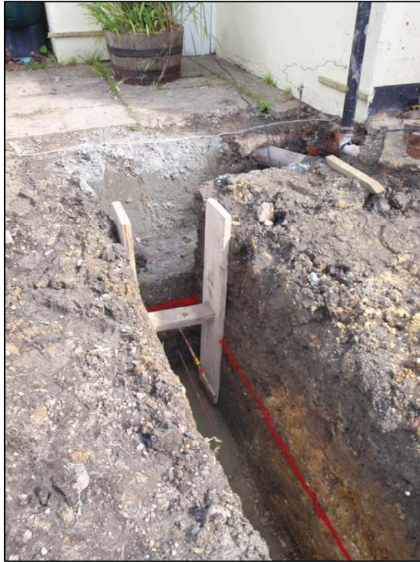
Plate I: view of pit in northeast corner of footing (camera facing east)
