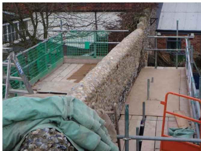
Area 2 Gardener's compound, wall head repaired.
