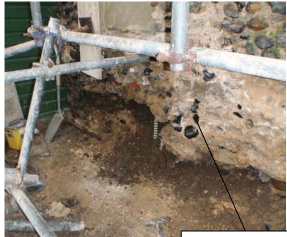
Modern repair, core of the north side reveal
