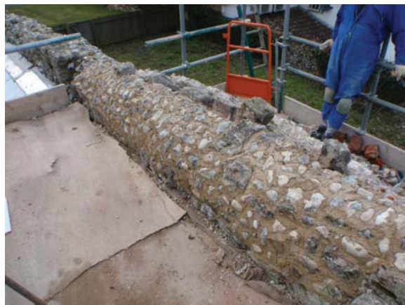
Wall head repairs area 6
