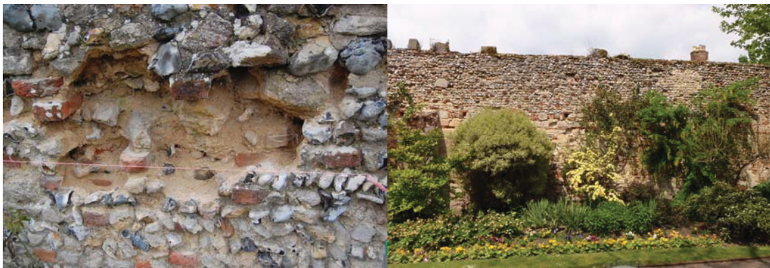
Post medieval wall core area 4, area 3 after repair
