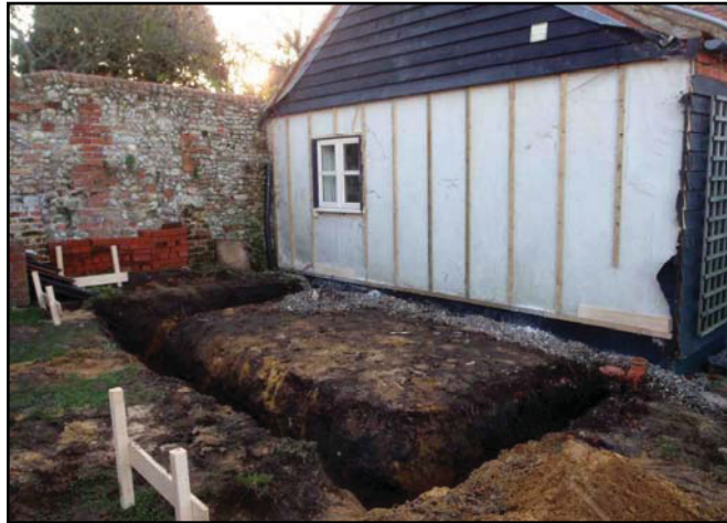
Plate 1. Phase 1 Extension facing SW
