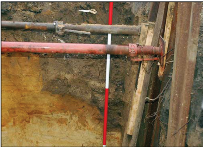
Plate 19. Feature 0407, facing E (scale 0.5m segments)
