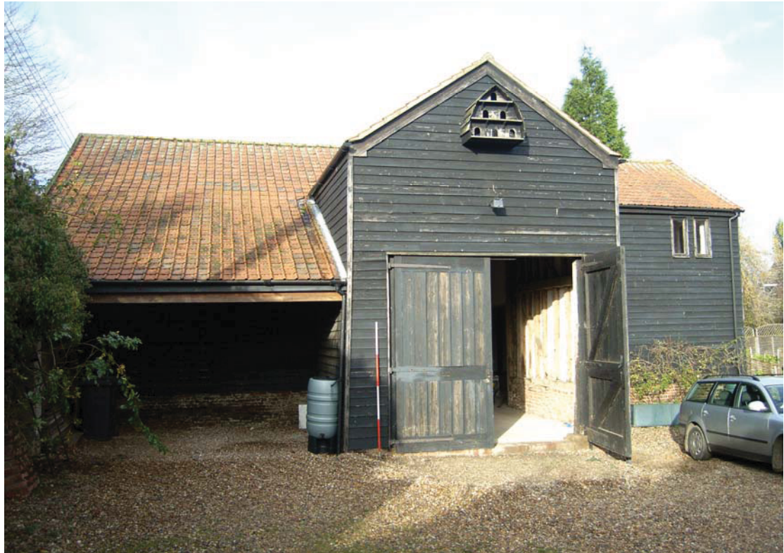
A2.3 External southern elevation showing central porch with lean-to shed to left and windows of converted eastern loft to right
