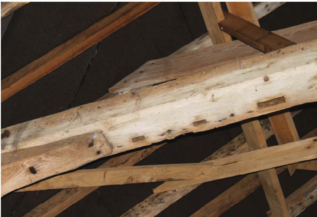
A2.6 Detail of re-used tie-beam to west of porch showing rectangular mullion mortises of clerestorey window with scars of cavetto mouldings in white paint.
