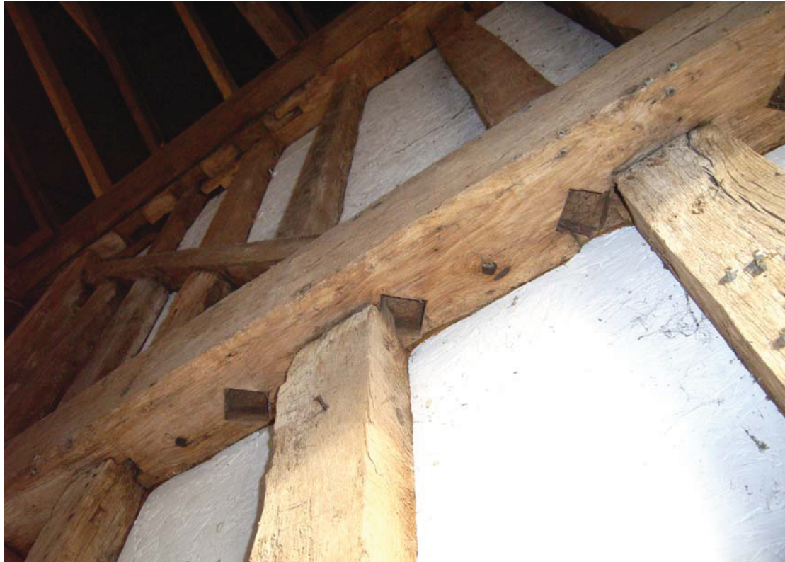
A2.9 Detail of re-used mid-rail in eastern side-elevation of porch showing mortises for diamond window mullions & glazing bars.
