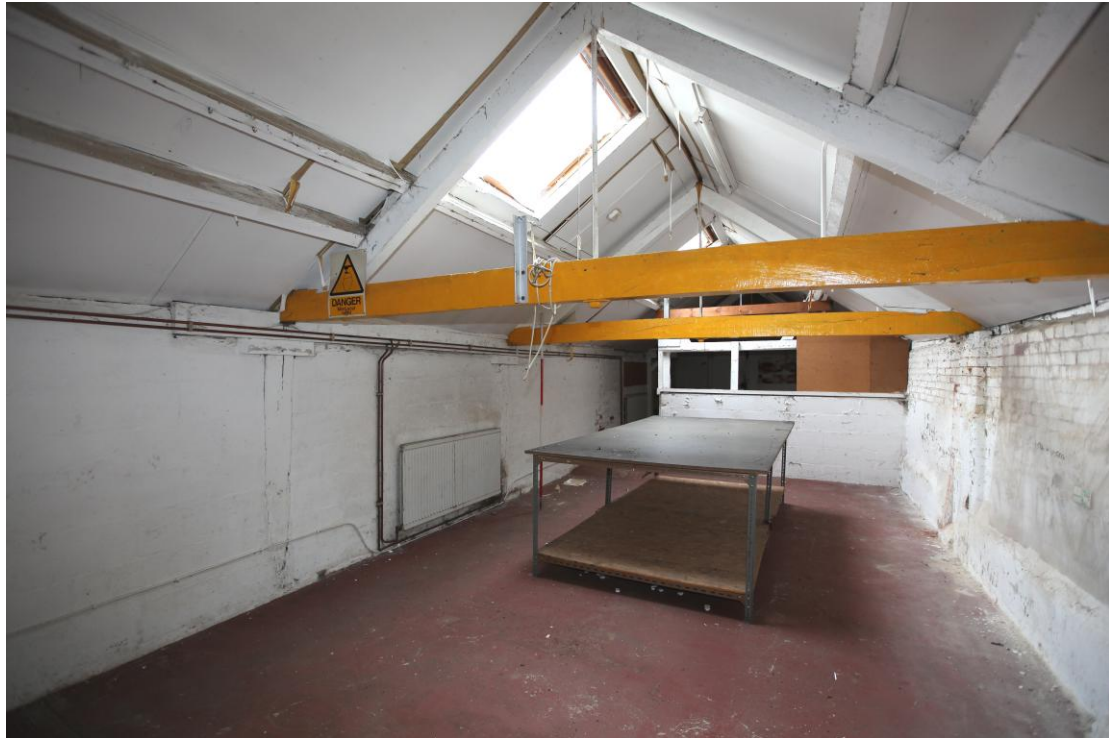
Illus. 11. Interior from north of western yard shed (D) showing arcade posts of blocked open arcade to yard (B) to left.
