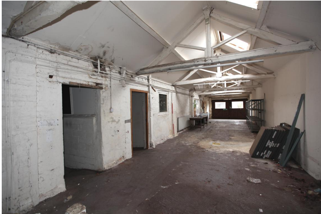
Illus. 9. Interior from east of rear range of yard (E) showing king-post roof trusses and doors to yard and sheds (F, B, D) to left. This area is understood to have operated as a milking parlour in the 20 th century and latterly as a piggery.
