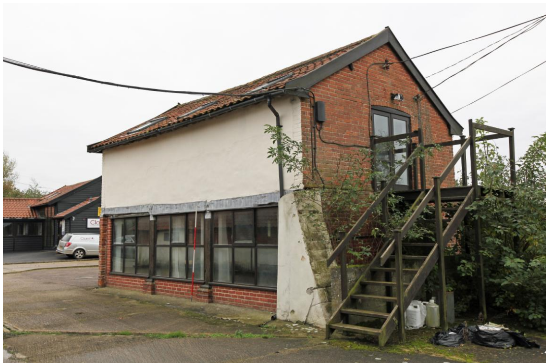
Illus. 6. Exterior of granary (C) from north-east showing renewed external stair to right and recently glazed open arcade of cart lodge to left. The previously converted timber-framed and weatherboarded building to the south of the site entrance is visible in the rear to left.
