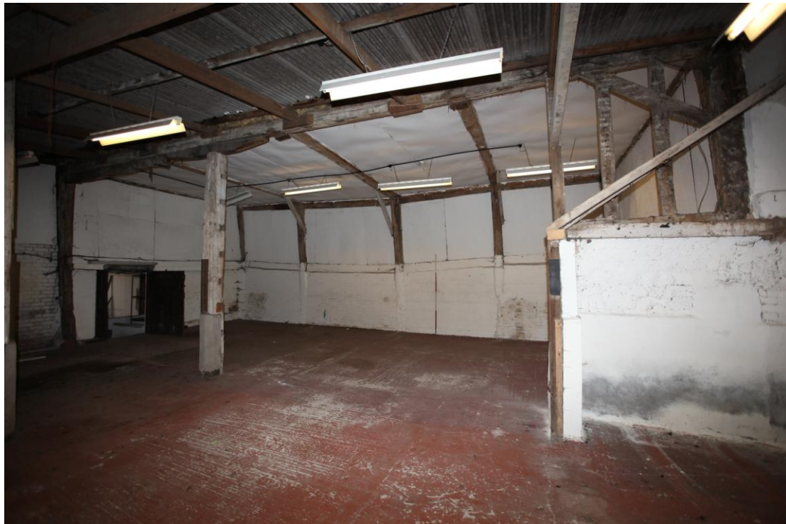
Illus. 14. Southern exterior of 'barn' (G) from 20 th century lean-to showing original studwork with externally trussed brace to right and modern boarding concealing the roof structure and the studs of the northern internal elevation.
