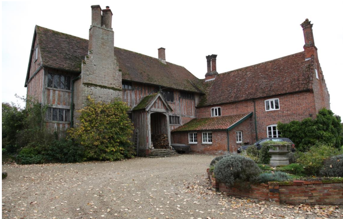
Illus. 3. Abbey farmhouse from rear (north-east) showing 18th century brick wing to right & truncated two-storied porch to cross-passage (with evidence of blocked door to missing porch chamber above). The parlour to the left has been demolished. Included for site context.
