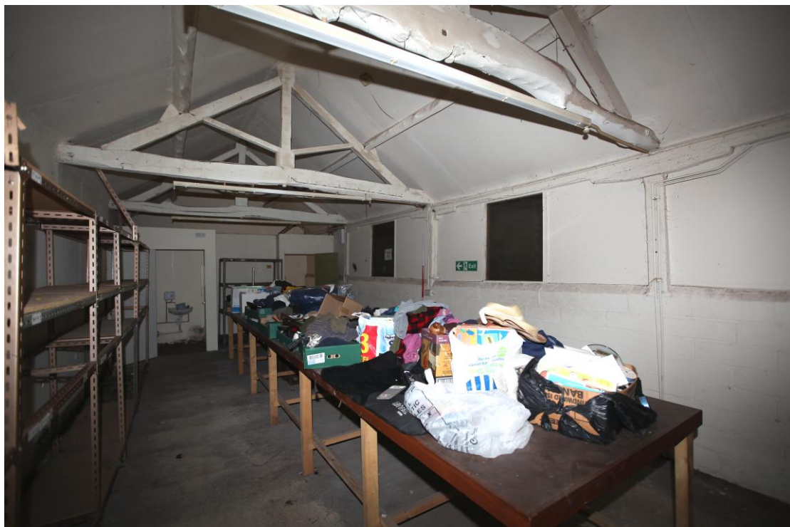
Illus. 10. Interior from north of eastern yard shed (F) showing arcade posts and shaped lintels of blocked open arcade to yard (B) to right.
