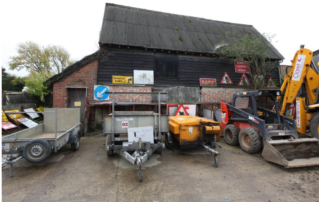
Illus. 12. Northern exterior of 'barn' (G) showing blocked first-floor loading door, corrugated asbestos roof covering and 20th century Fletton brickwork to lower storey. The loading door occupies the approximate position of an original 16 th century loading door with a ground-floor entrance beneath, but is concealed internally. A second first-floor loading door lay to the right.
