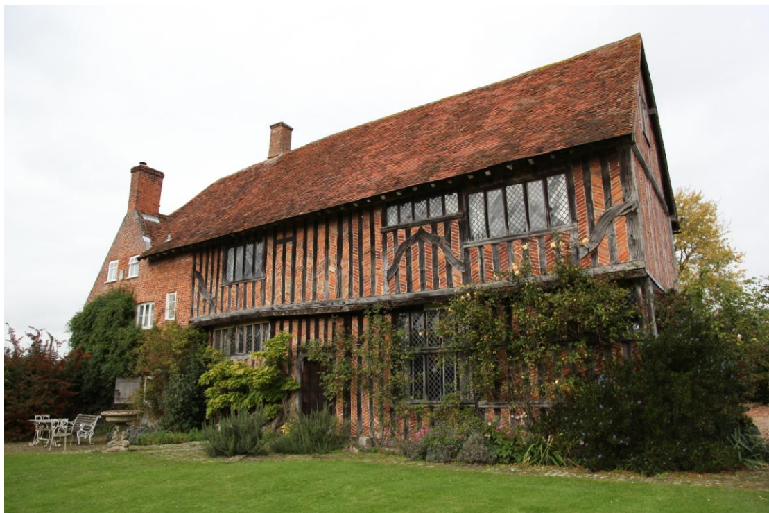
Illus. 4. Much restored jettied southern facade of late-16th century Abbey farmhouse showing position of two-storied porch to cross-passage in centre (with blocked door to porch chamber) with position of missing parlour to right. The 'serpentine' bracing is typical of the final quarter of the century. Included for site context.
