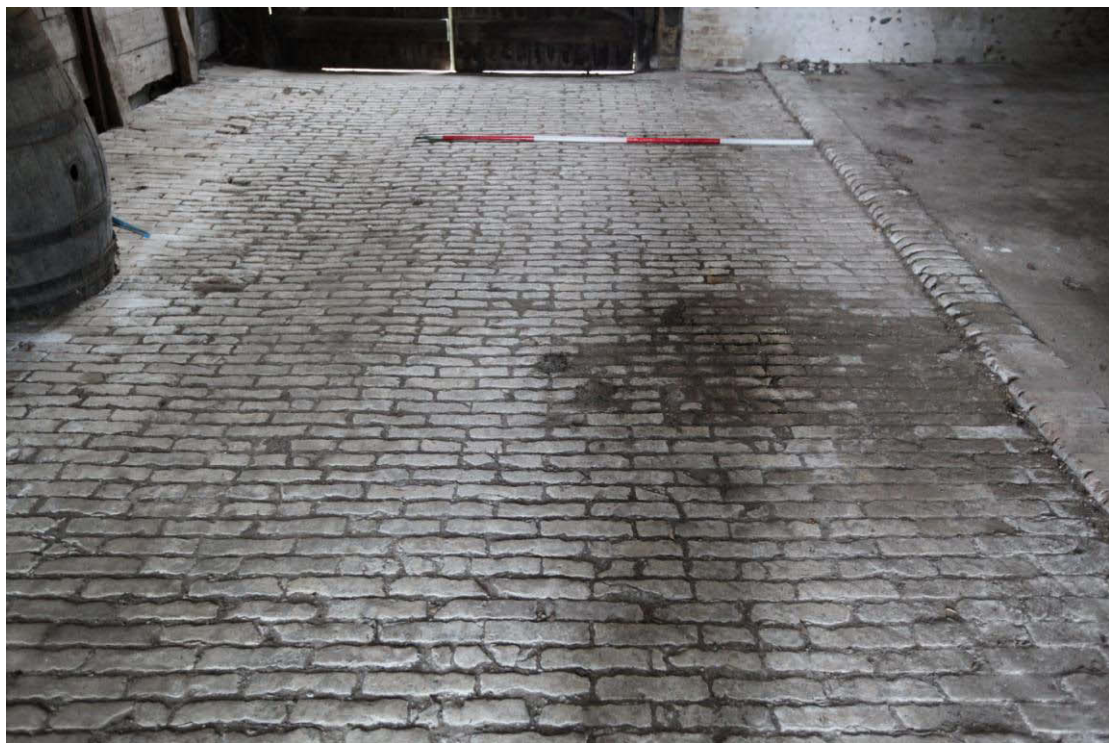
Illus. 12. The exceptionally well preserved threshing floor of gault brick in the flint barn (1) seen from the west, showing its raised southern edge to the right with modern concrete beyond.
