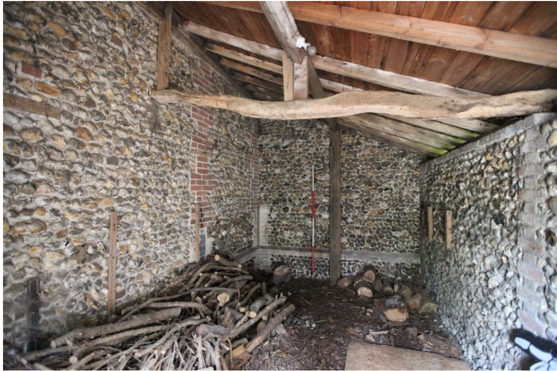
Illus. 9. The interior from the west of the secondary lean-to flint shed (3) adjoining the flint barn (1) and showing the porch to the left. The wall of the lean-to to the right is not integral to the fabric of the barn.
