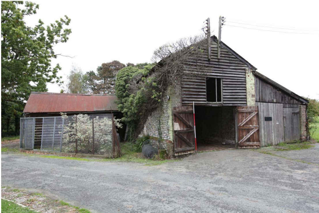
Illus. 1. Exterior of barn complex from west showing the small timber-framed stable (2) to left, the gabled porch of the flint barn (1) with reduced doors in the centre and the slightly later lean-to shed (3) to the right
