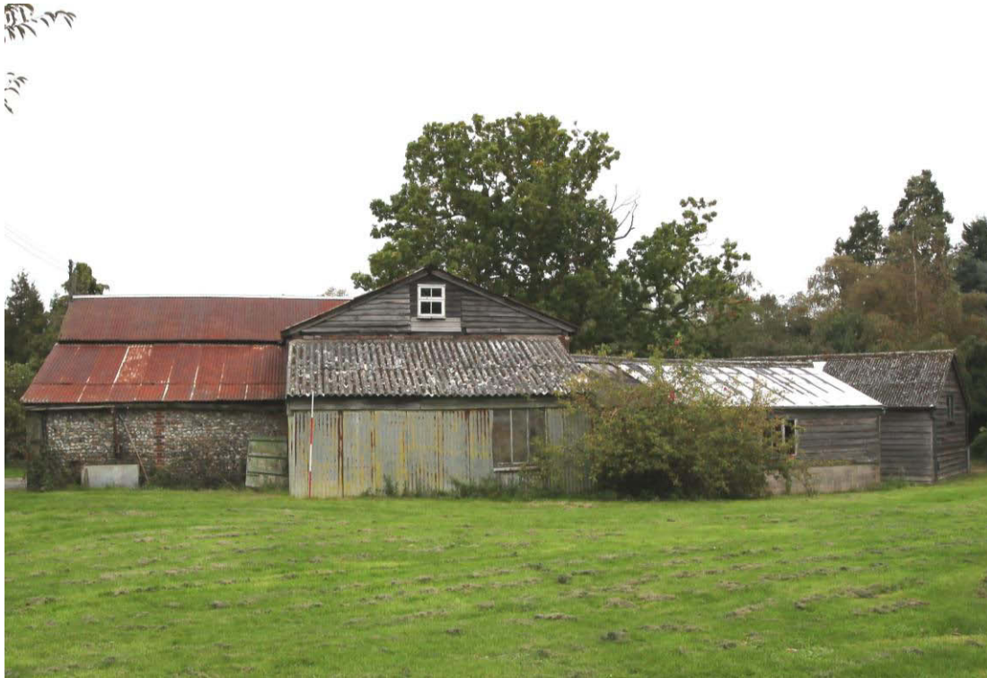
Illus. 3. The view from the garden to the south showing the porch and lean-to shed (3) to the left, the southern gable of the flint barn (1) with its lean-to shed (4) in the centre and the two late-20 th century boarded sheds at irregular angles to the right.
