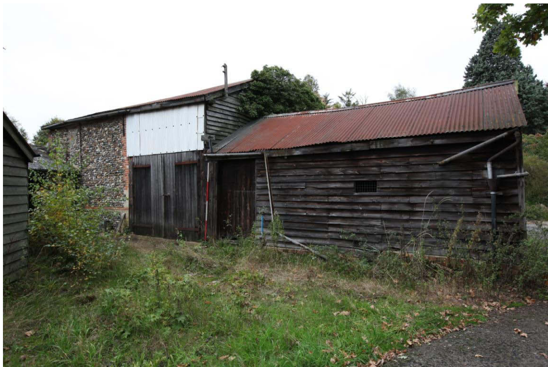
Illus. 6. The Eastern exteriors of the stable (2) to the right and the flint barn (1) to the left showing their respective doors side-by-side. Both buildings were re-roofed in the 20 th century and are covered in corrugated iron. The barn doors have been reduced in height.
