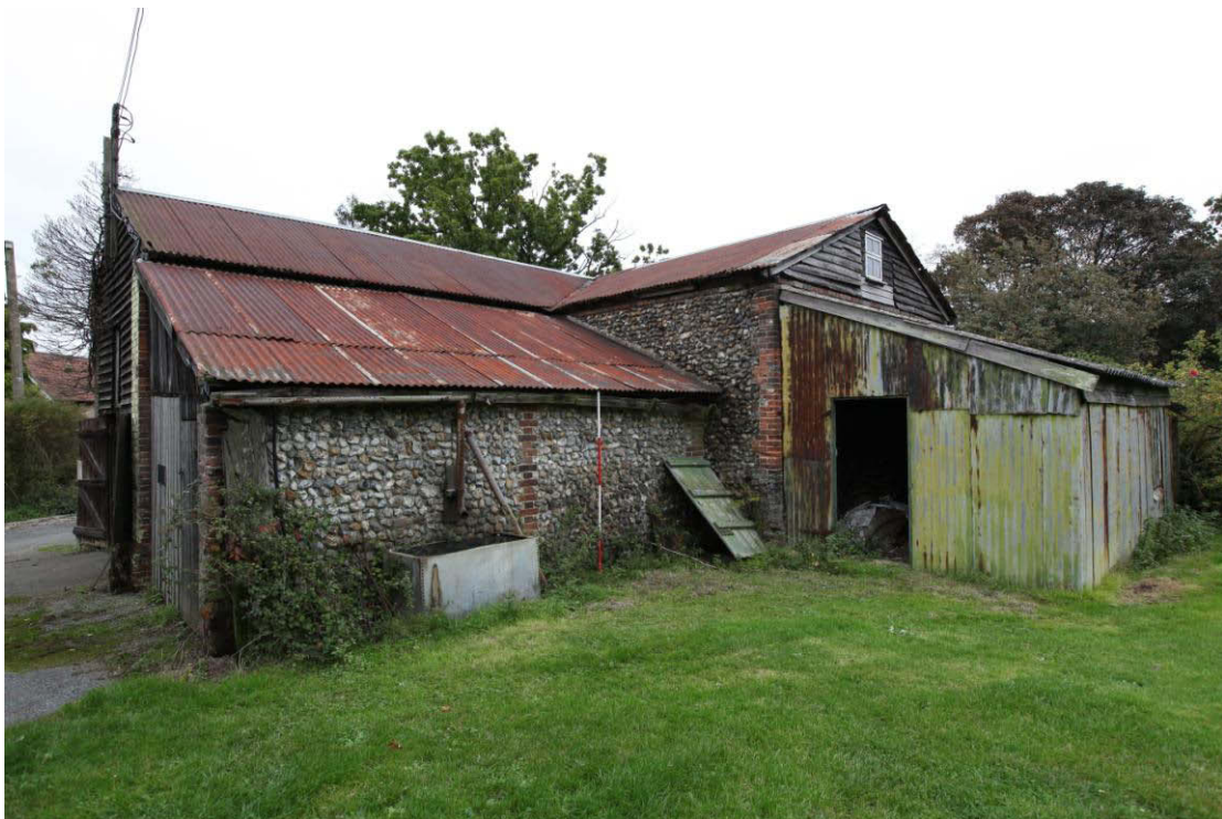
Illus. 2. Exterior from south-west showing the flint barn (1) with its unusually long porch and lean-to shed (3) to the left and the 20 th century corrugated iron lean-to (4) adjoining its southern gable to the right.
