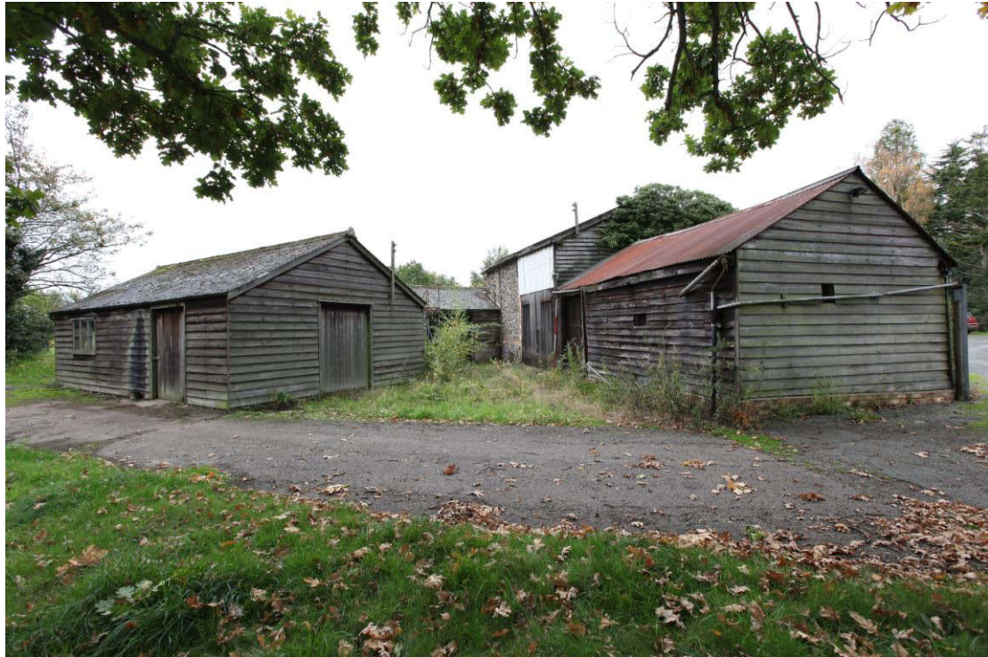
Illus. 5. Exterior from north-east showing the single-storied timber-framed stable (2) to the right and the 20th century shed (6) to the left with the flint barn (1) in the centre.
