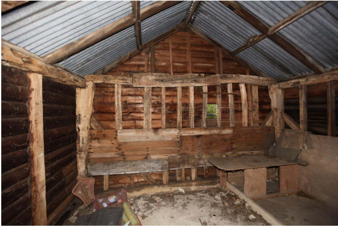
Illus. 7. The internal northern gable of the stable (2) showing extensive re-used timber with primary bracing and 20 th century roof.
