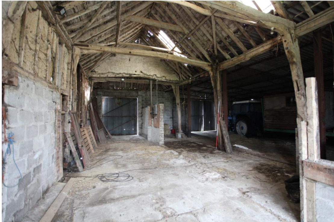
Illus. 5. General internal view of the barn (5) from the north showing the missing studs of the rear (western) elevation to the right and the largely intact studs of the eastern facade to the left. The remaining section of the daub partition against the stable bay (5a) is visible in the rear.
