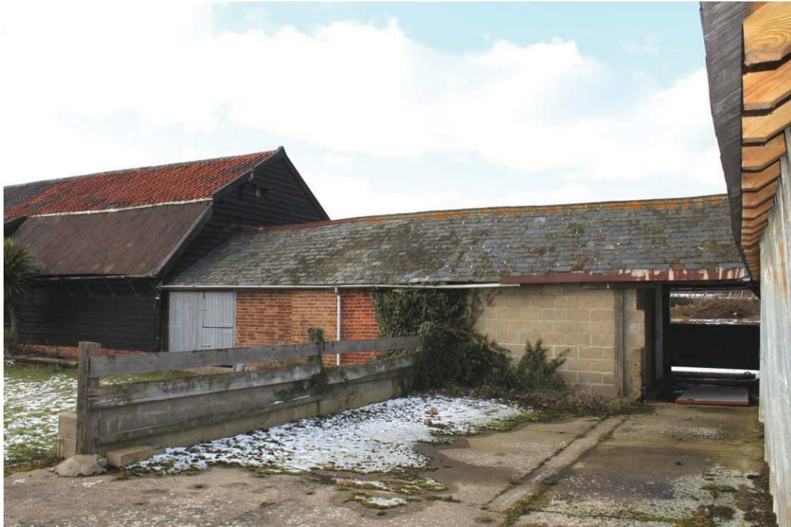
Illus. 3. The southern exterior of the enclosed shed (1) showing the secondary through-passage adjoining the corner shed (2) to the right and the barn (6) to the left. This elevation was extensively altered in the 20 th century with new doors to the left and cement-block rebuilding to the right.
