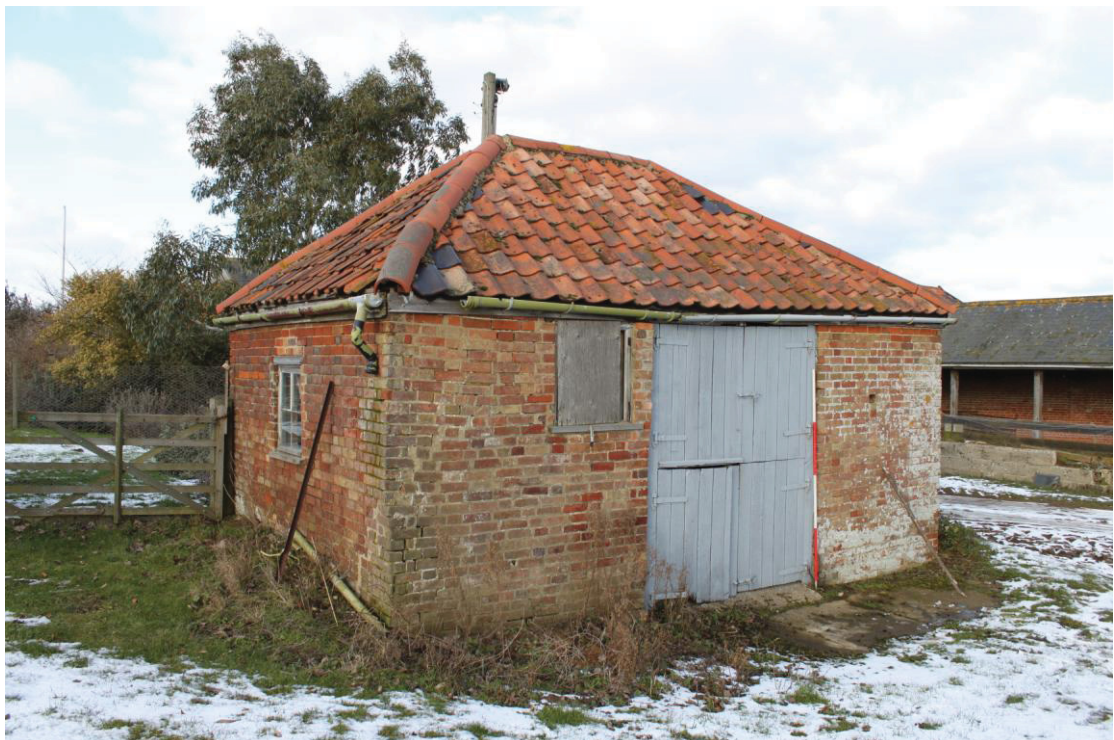
Illus. 10. The exterior of the workshop (5), which probably originated as a bull box or possibly a vehicle shed with its present double doors but without windows.
