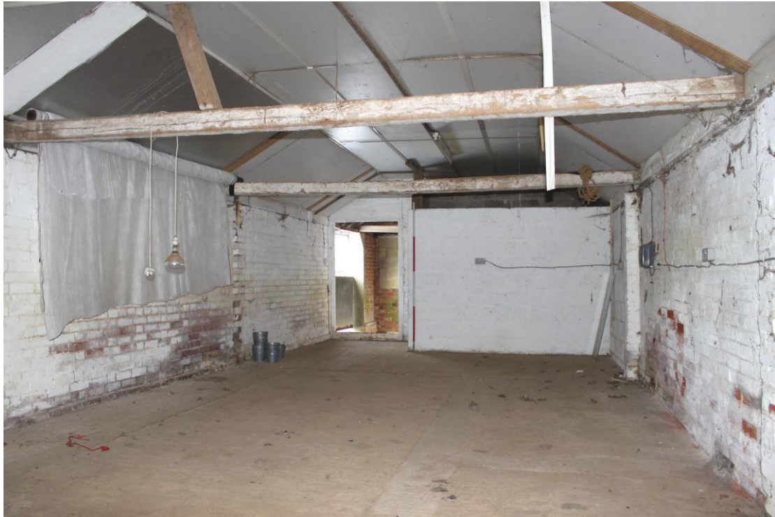
Illus. 5. The interior of the heavily altered enclosed shed (1) from the west showing the cement-block partition adjoining the secondary through-passage in the rear with the scar of a missing original lateral partition to the left.
