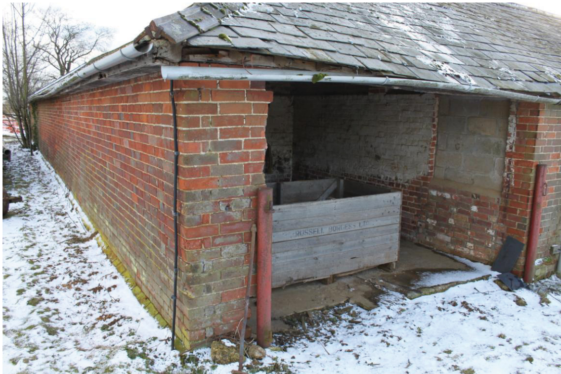
Illus. 4. Exterior of the corner shed (2) from the north showing its secondary access (breaking the original brickwork) with the eastern elevation of the adjoining shelter-shed (3) to the left. The blocked original internal entrance is visible to the right.
