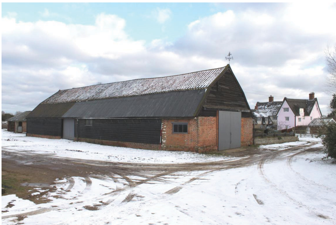
Illus. 2. General view of the site from the north-west showing the grade II*-listed timber-framed barn of circa 1300 (6) in the foreground with the corner shed (2) to the left and the unlisted farmhouse to the right.
