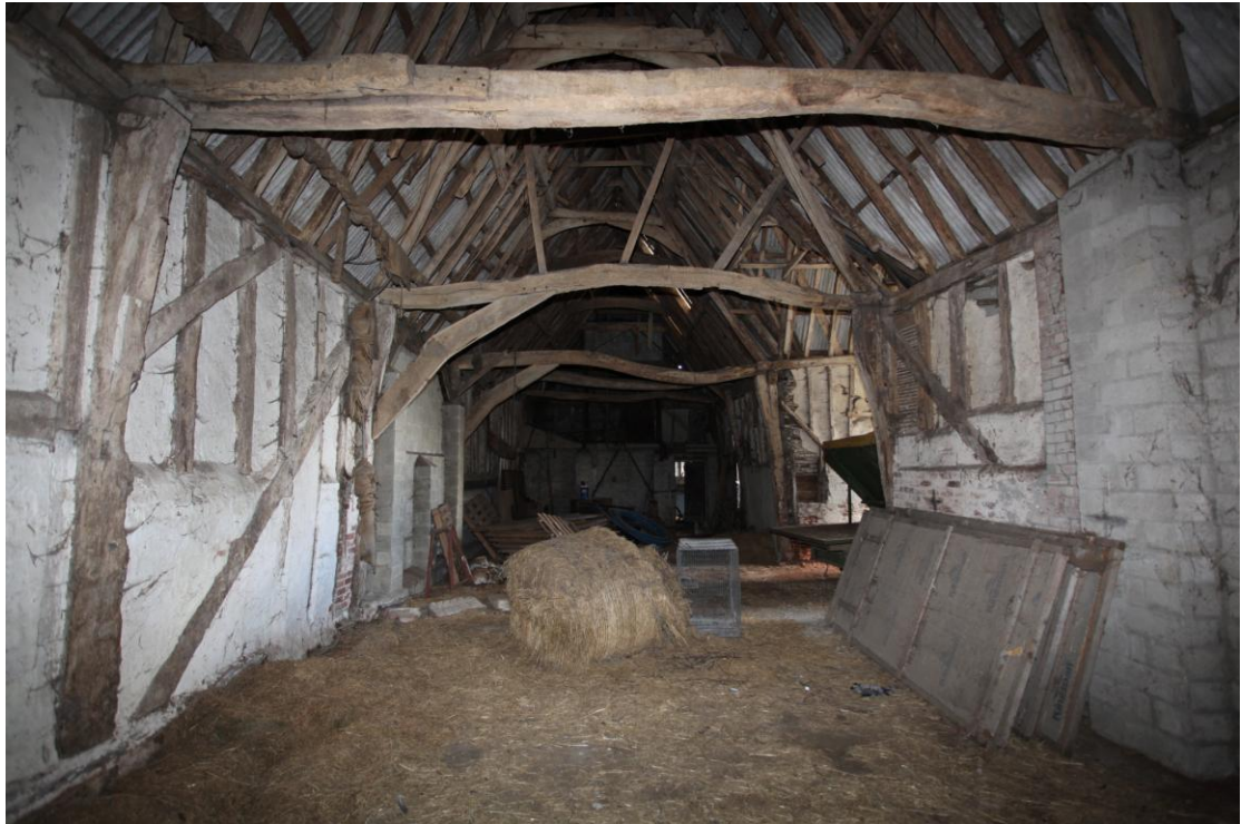
Illus. 3. Interior of barn (1) from north-west showing the two original arch-braces flanking the blocked north-eastern door to the left. The tie-beam in the foreground was inserted to replace the tie-beam of the original partition between the stable (1b) and three-bay barn (1a), of which a small section survives to the left.
