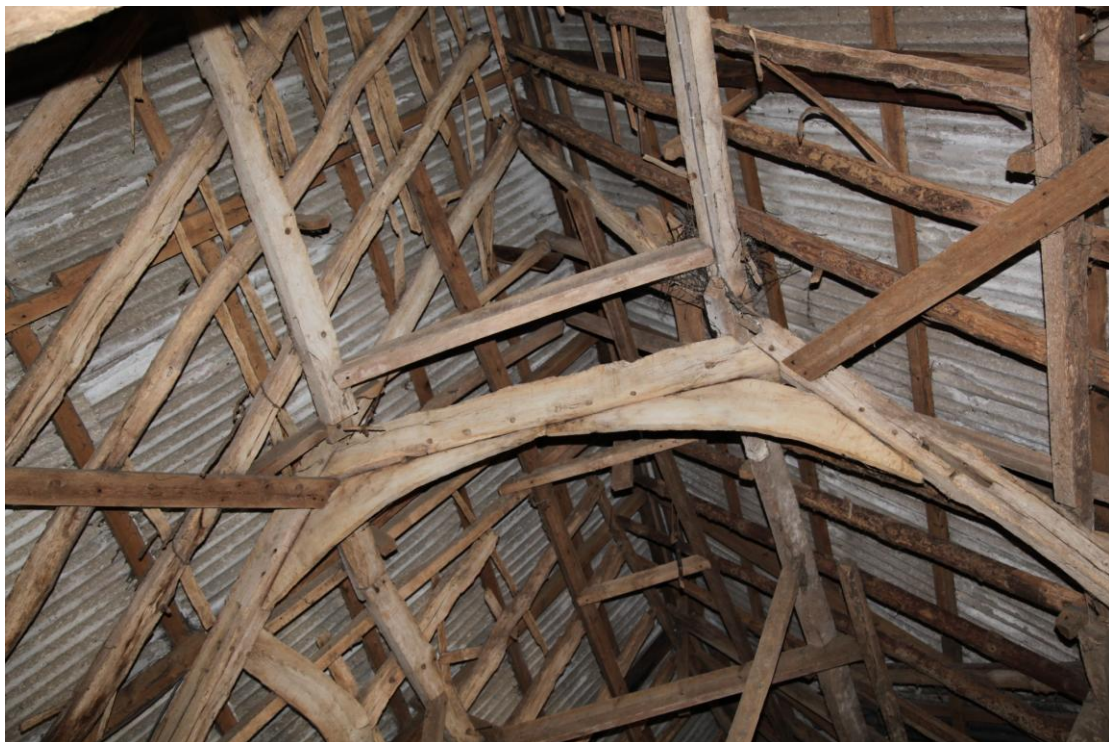
Illus. 6. Detail of the intact 16 th century roof truss to the north-west of the threshing bay of the barn (1a), seen from the north-west, showing its tenoned collar braces and empty mortises for missing wind-braces beneath. An original wind brace is visible at bottom-left (now nailed to the rafters).
