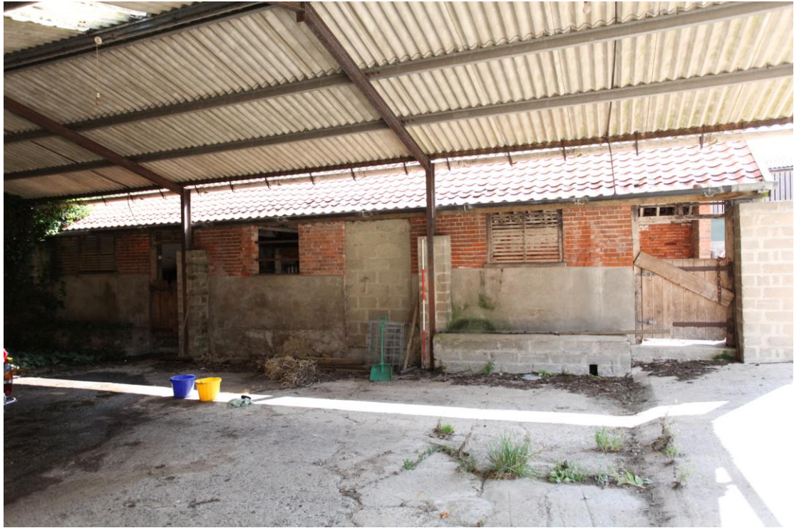
Illus. 13. The north-western exterior of the eastern cow-shed (6a) seen from the adjoining 20 th century covered yard showing its original doors and louvered windows (the central door blocked).
