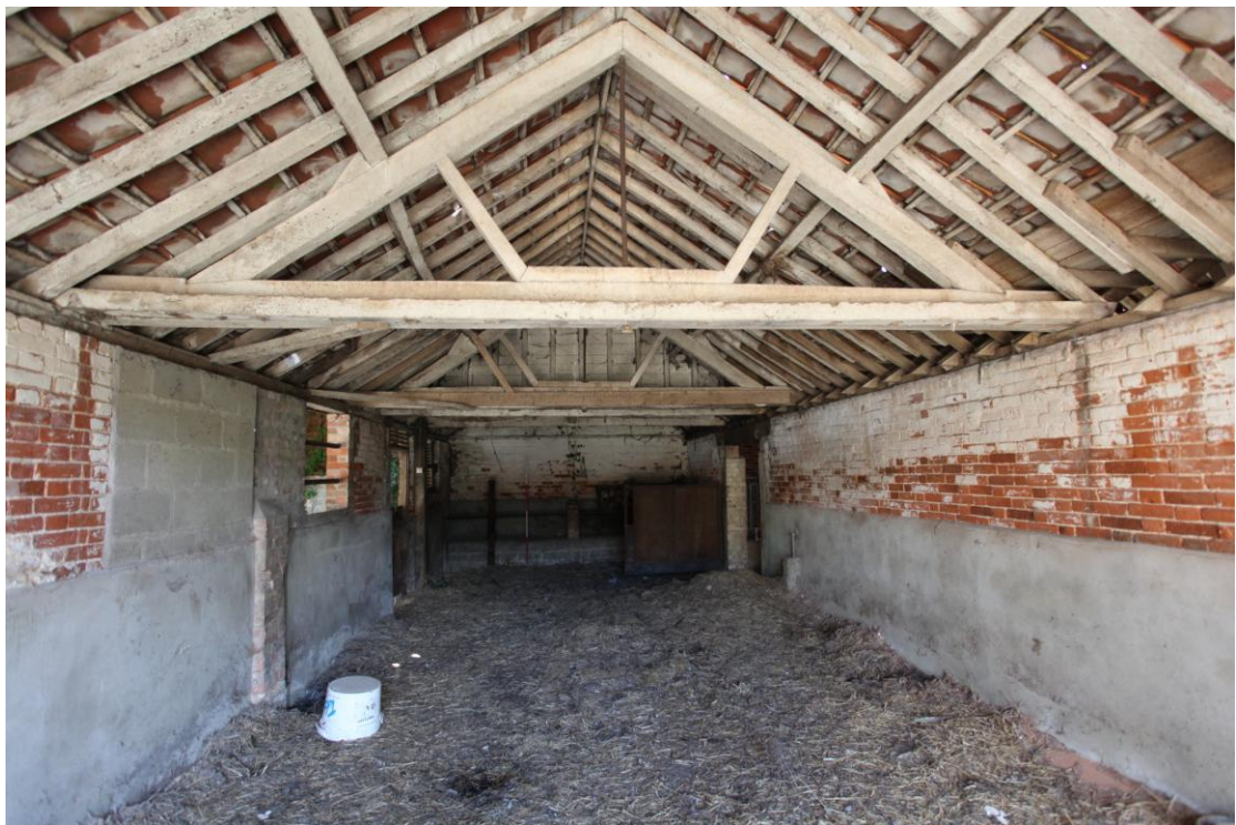
Illus. 14. The interior of the eastern cow-shed (6a) from the south-west its missing internal partitions and a low, 20th century concrete manger in the rear.
