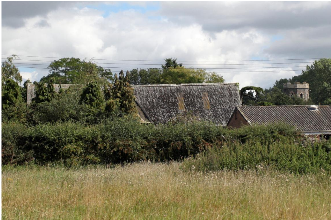
Illus. 1. Exterior of barn (1) from south-west showing profile of corrugated roof and gabled porch with 20th century brick shed & the 12 th century round tower with 19 th century octagonal top of St Mary's parish church to right.
