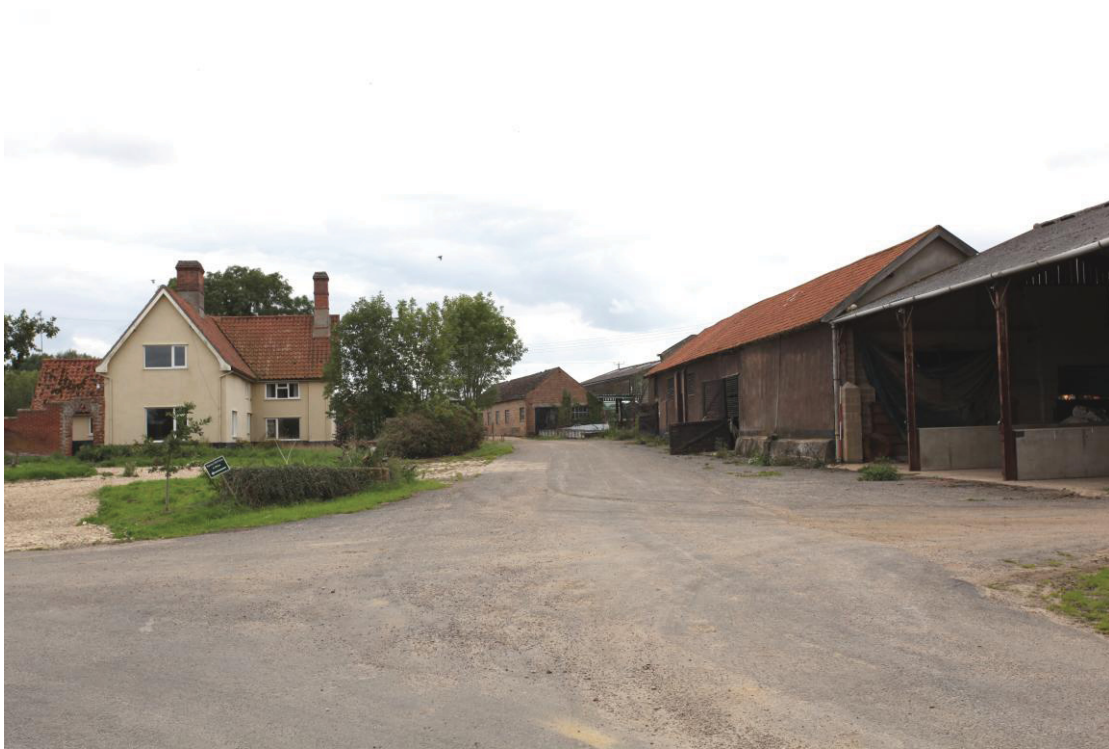
Illus. 1. General view of site from northern approach showing the unlisted former farmhouse to the left (marked as Warrenhill Farm Cottages in figure 1 but unified and unoccupied at the time of inspection) and the pantiled barn to the right. The right-hand wing of the house was severely truncated to widen the farm track in the early-20 th century
