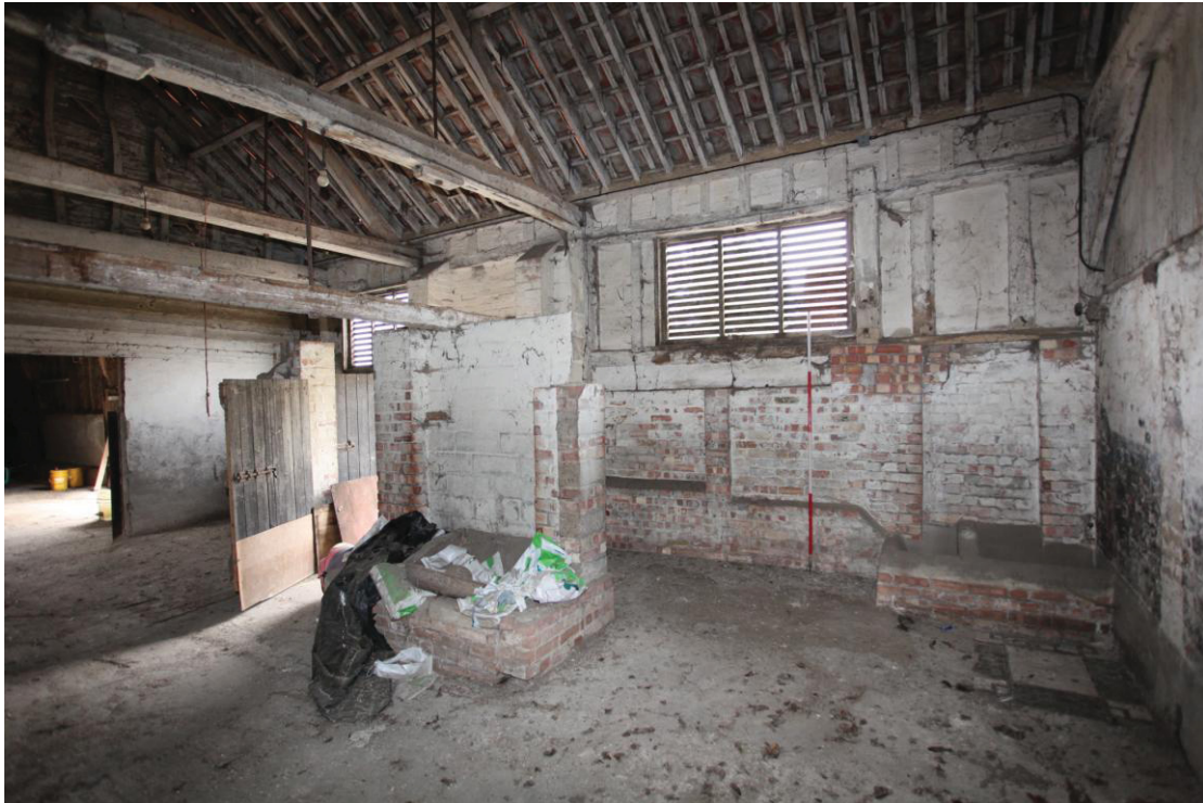
Illus. 9. The eastern interior of the northern stable (2a) showing the raised walls which have been largely rebuilt in 20th century brickwork.
