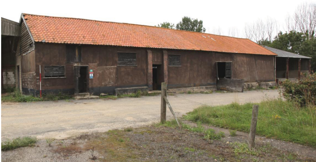
Illus. 2. The eastern external elevation seen from the former farmhouse, showing the colour-washed cement render and the entrances to the threshing barn (1) to the right and the two stables (2a and 2b) to the left.
