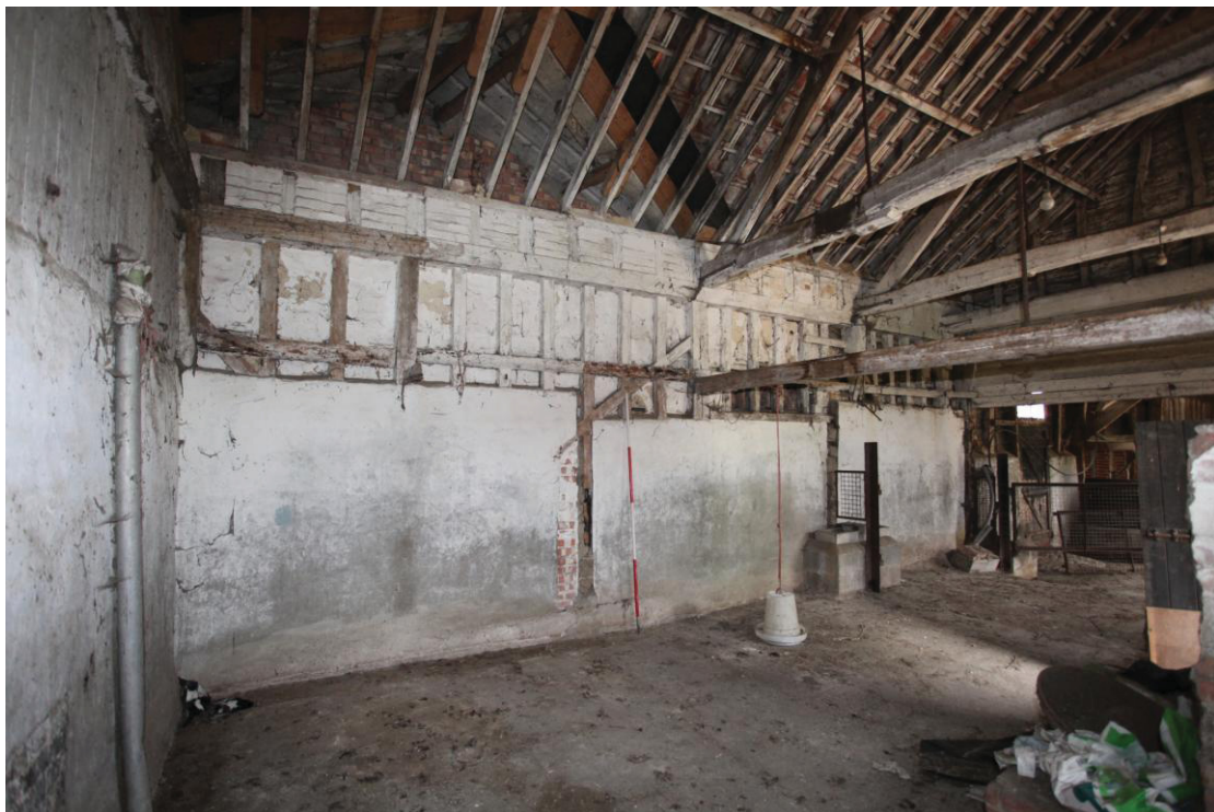
Illus. 8. The western interior of the northern stable (2a) showing its raised walls and primary bracing with a horizontal rail or clamp which supported the joists of a missing hay loft.
