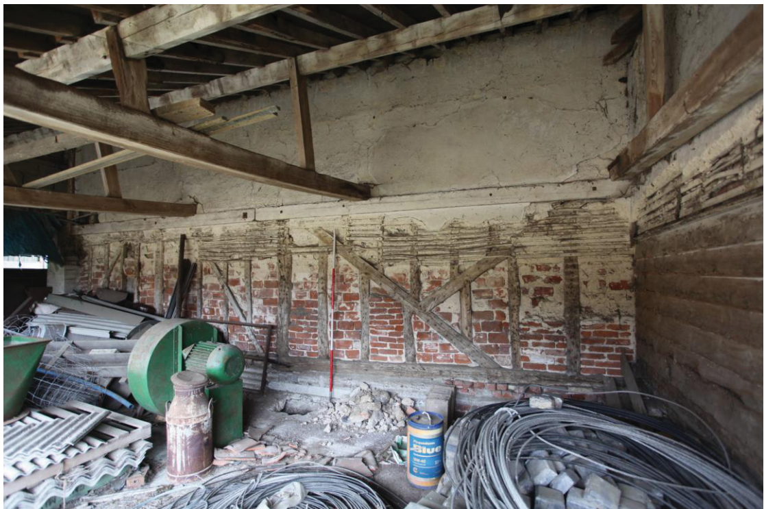
Illus. 4. The western exterior of the barn (1) protected within the shelter-shed (3) showing its original whitewashed lath-and-plaster with brick infill to the studwork beneath. The porch (1a) to the right is clad in horizontal boarding with render above – a common ‘two-tier’ technique of the early-19 th century.
