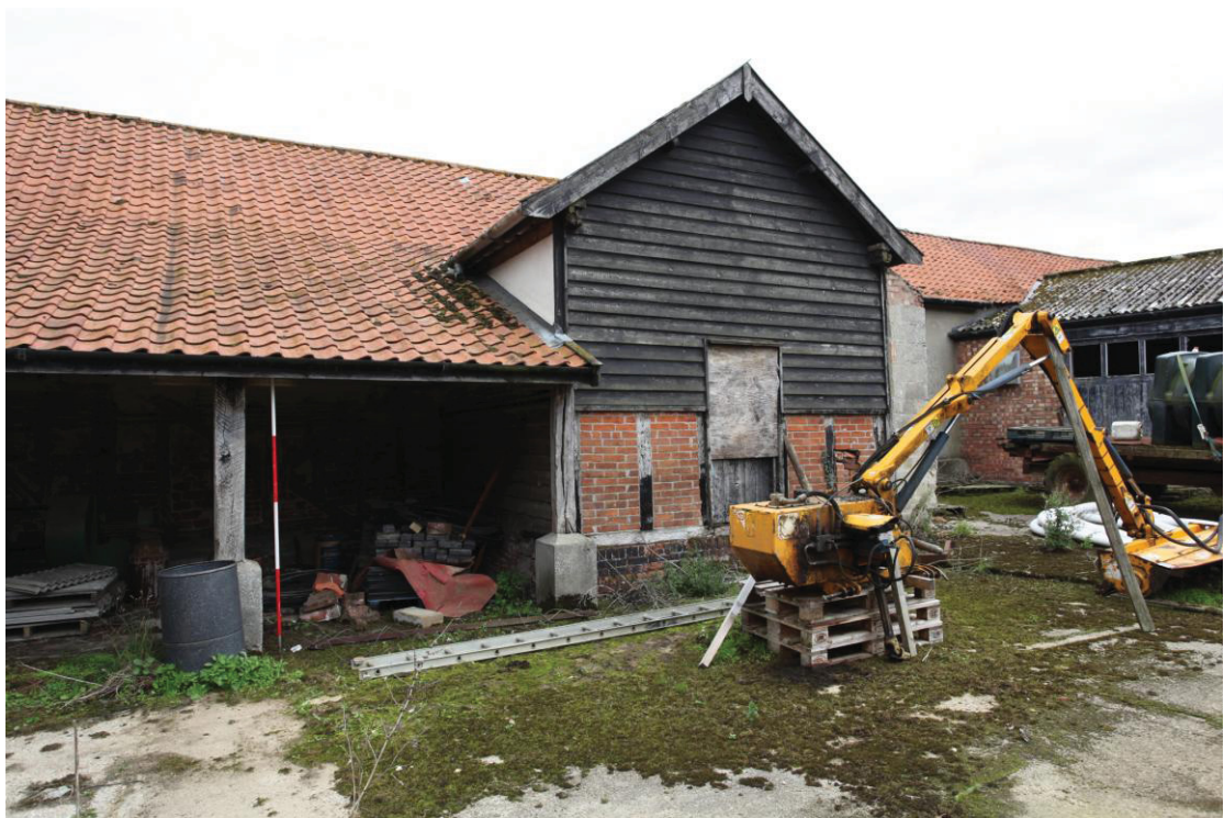
Illus. 3. The western exterior of the gabled porch of the barn (1a) showing its modern weatherboarding and brickwork with the open-sided shelter-shed (3) to the left.
