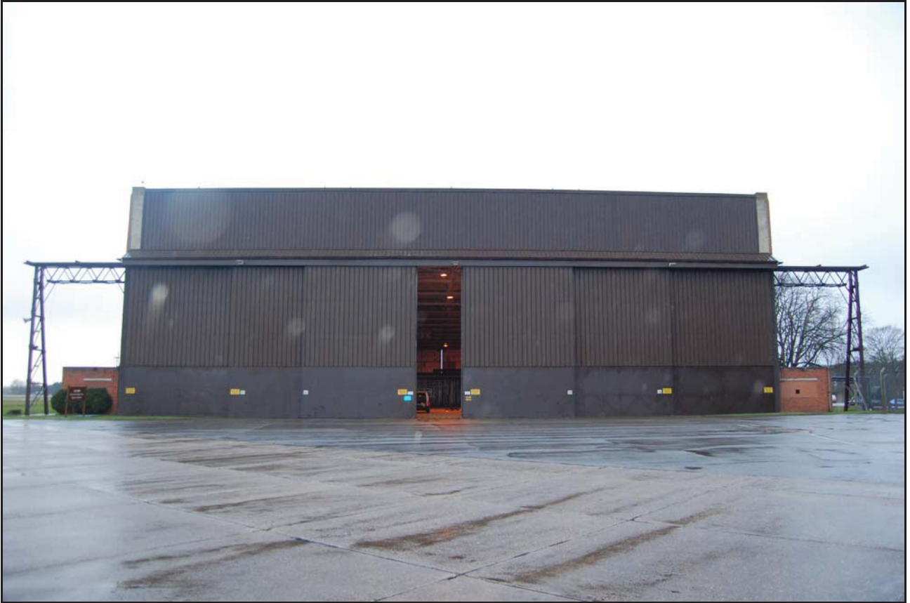
Plate 2. Hangar doors, facing WSW
