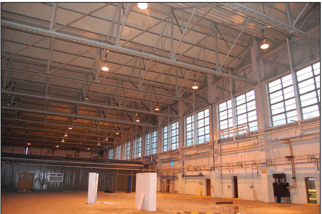
Plate 7. Internal, showing roof and structural detail
