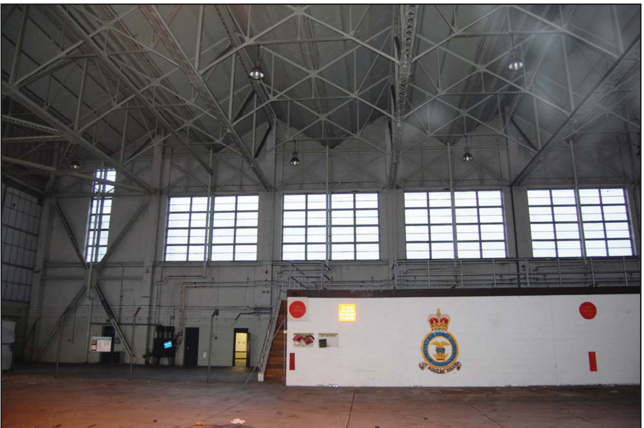
Plate 3. Internal elevation showing window and roof detail, facing SSE
