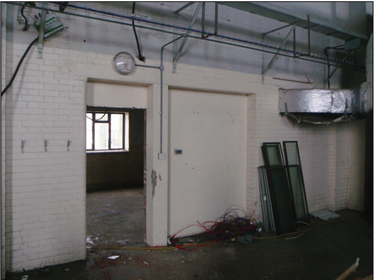
Plate 5. Blocked large door, converted into single door
