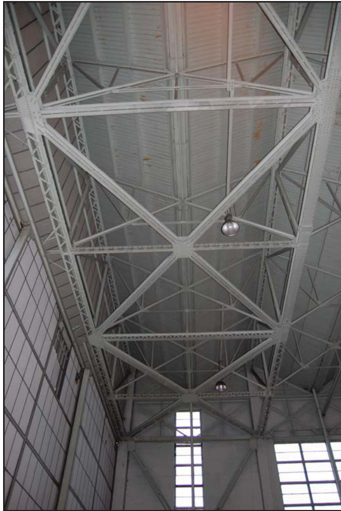
Plate 8. Roof structure of end bays
