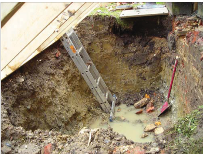
Plate 1. View of the underpinning trench, looking east.
