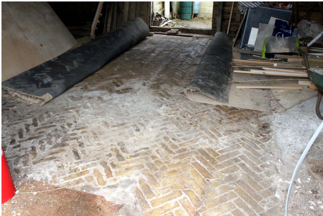
Illus. 4. The unusually well preserved original herringbone threshing floor of gault brick in the barn's central bay, as seen from the north-west.
