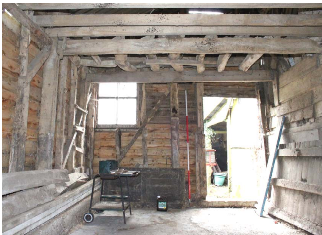
Illus. 6. Interior of lean-to stable (2) from north-west showing the remaining original ceiling joists in the rear with the loft ladder to the left. The joists in the foreground are modern replacements
