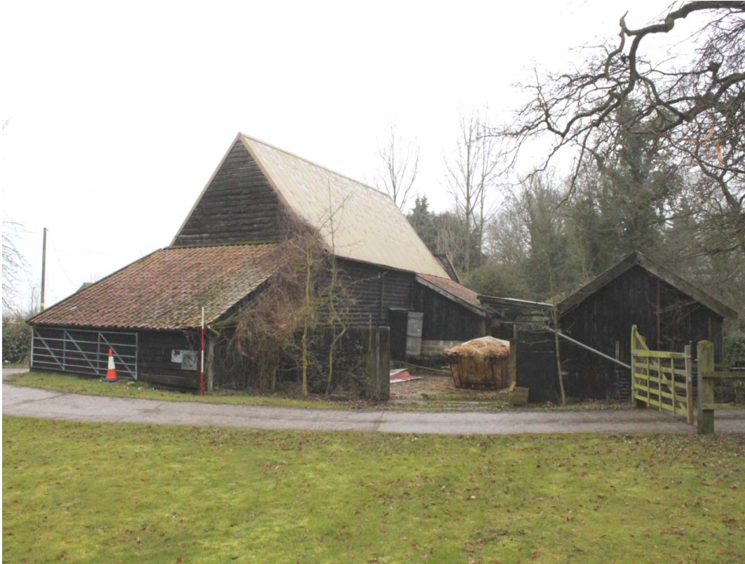
Illus. 3. Exterior of barn complex from south showing barn to left and pantiled shelter shed (8) to right.
