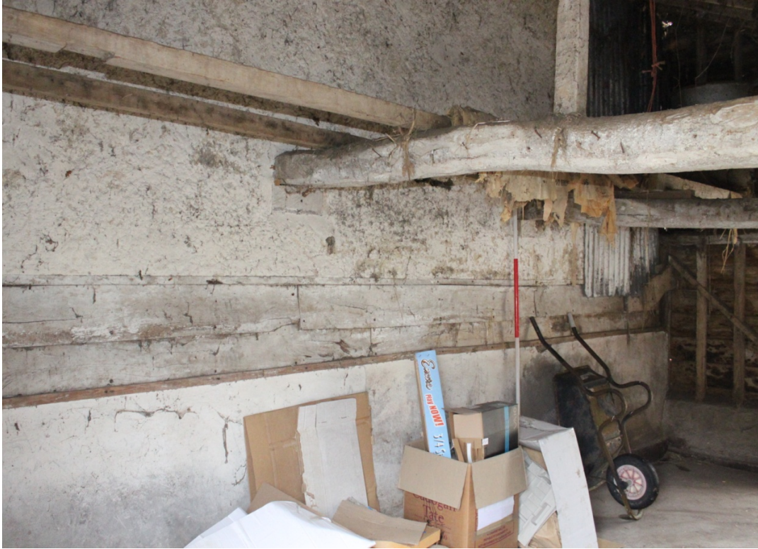
Illus. 7. The original two-tier external cladding of the barn's south-western gable preserved in the adjoining lean-to shed (3). The lower tier of weatherboarding is partly hidden by 20 th century render, but the roughcast clay daub remains intact above.
