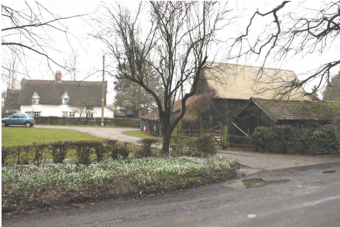
Illus. 1. General view of site from Fingal Street to south-east showing farmhouse to left and barn to right.
