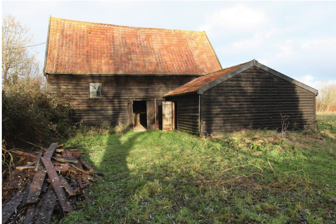
Illus. 3. The southern exterior of the barn showing the much altered single-storied shed (2) adjoining the original low rear doorway of the main barn (1).
