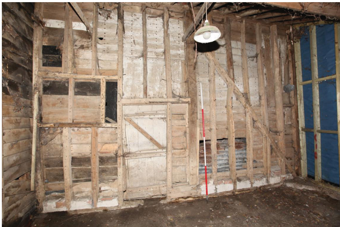
Illus. 10. The interior of the southern shed (2b) from the west showing the unusual internal partition consisting largely of re-used doors which adjoins the eastern section of the same shed (2a).
