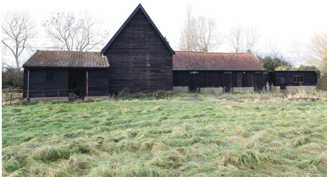
Illus. 4. The eastern exterior of the complex showing from left to right the southern shed (2), the main barn (1), the roadside shed divided into three loose boxes (3) and the 20 th century pentice sheds (4 & 5).
