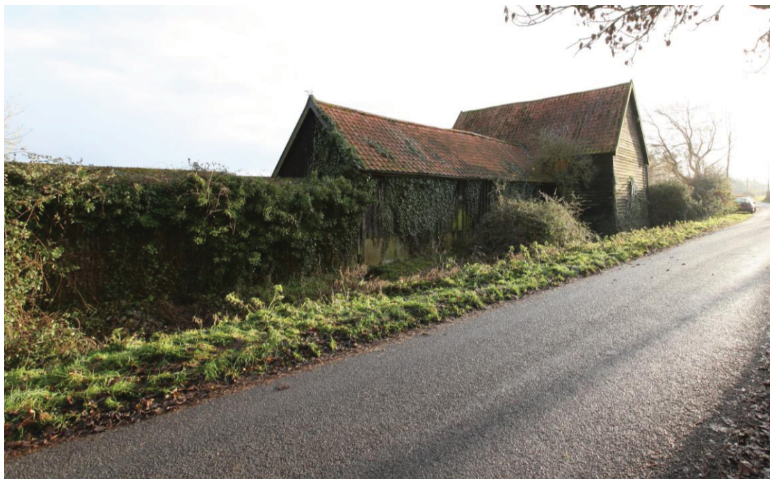
Illus. 2. General view of the site from Rookery Road to the north showing the main barn (1) at right-angles to the road in the rear with the later roadside shed (3) blocking its original central entrance in the centre and the overgrown wall of the pentice (single-span) 20 th century sheds (4 and 5) to the left.
