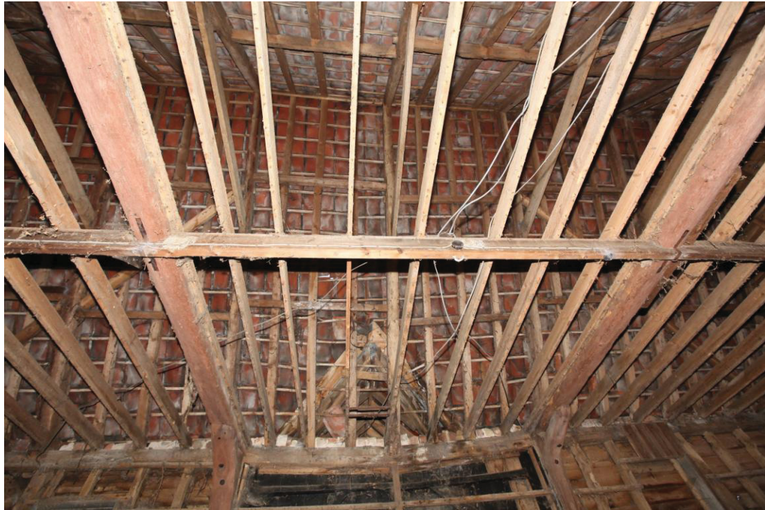
Illus. 7. The roof structure of the barn (1) viewed from the south showing two tiers of staggered butt-purlins with the joists of the inserted 20 th century ceiling in the foreground.
