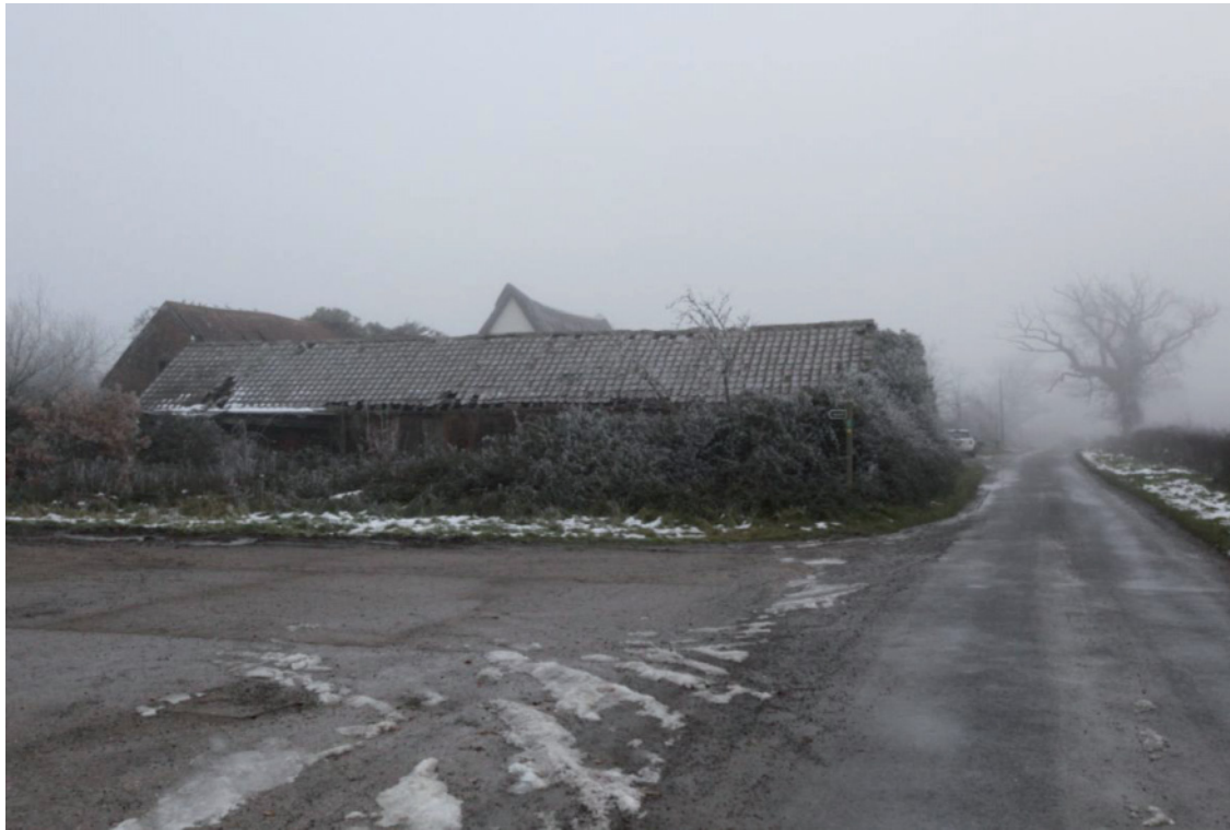
Illus. 1. Exterior of complex from north showing the site of the demolished cart lodge (11) with the pantiled roof of the stable (5) in the foreground and the steeply pitched thatched gable of the previously converted barn (4) in the rear.
