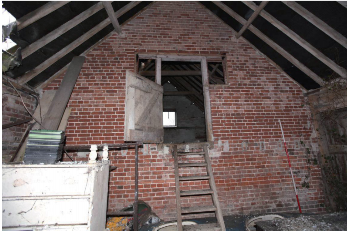
Illus. 5. Southern external gable of the granary (1) seen from the slightly later granary shed (2) and showing the ladder to the first-floor grain floor and the windows flanking the door. This gable was open to the elements before the granary shed was constructed.
