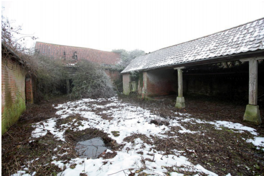
Illus. 7. Western end of the horse yard showing the open arcade (6b) and enclosed loose box (6a) to the right with the granary (1) in the rear and the stable (5) to the left. The boarded upper storey and open lower storey of the granary is visible between the brambles.
