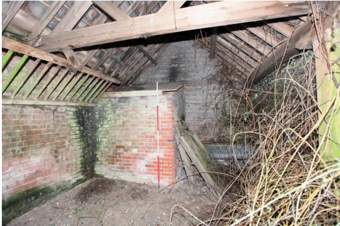
Illus. 9. Western interior of the shelter-shed (6b) showing the hay rack to the left and the enclosed brick shed (10) in its south-west corner which unusually extends across only half the shelter-shed's width. This is an entirely original arrangement.
