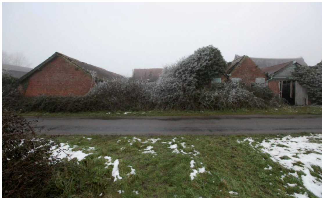
Illus. 2. Exterior of roadside western gables showing the stable (5b) to the left with the converted thatched barn (4) in the rear to right. The doors and windows of the enclosed feed sheds in the ends of the shelter-sheds (6 & 7) are visible behind brambles in the centre, with the shallow-pitched gable of the later covered yard (8) to the extreme right.
