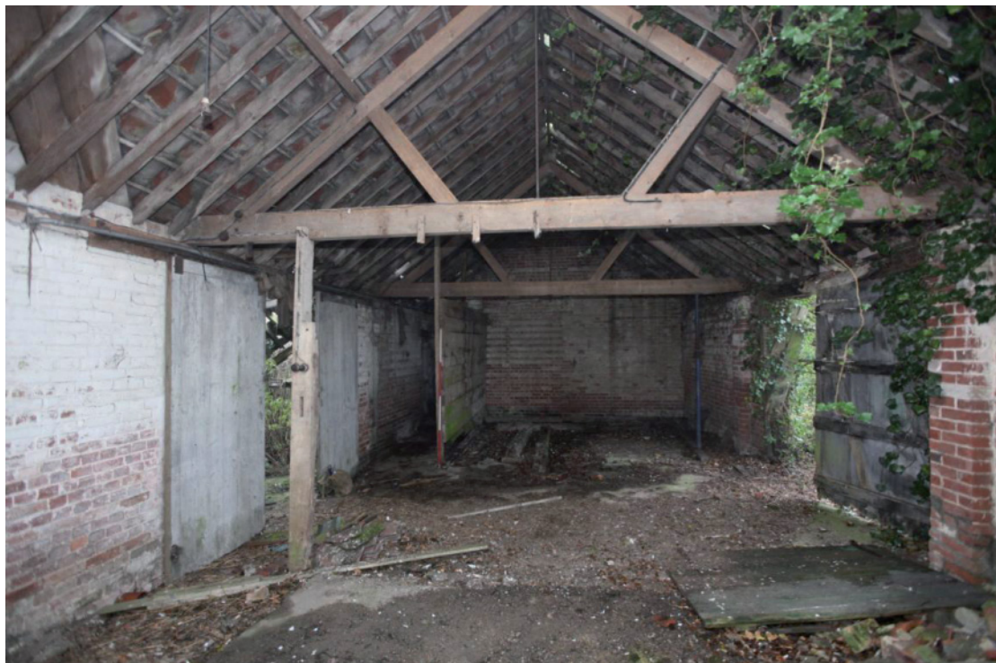
Illus. 4. Interior of the eastern shed (3) seen from the south, showing its softwood roof structure with original external double-doors to the right and inserted double doors to the southern yard (8) to the left. The narrow boarded passageway in the rear leads to a door which opens onto the horse yard.
