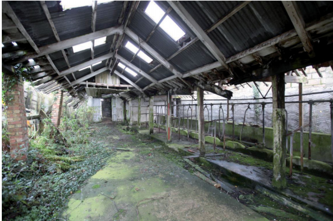
Illus. 3. Interior from west of the 20 th century covered yard (8) showing the 20 th century milking parlour stalls in the southern shed (9) to the right and the 20 th century Fletton-brick piers of the largely collapsed shelter-shed (7) to the left.
