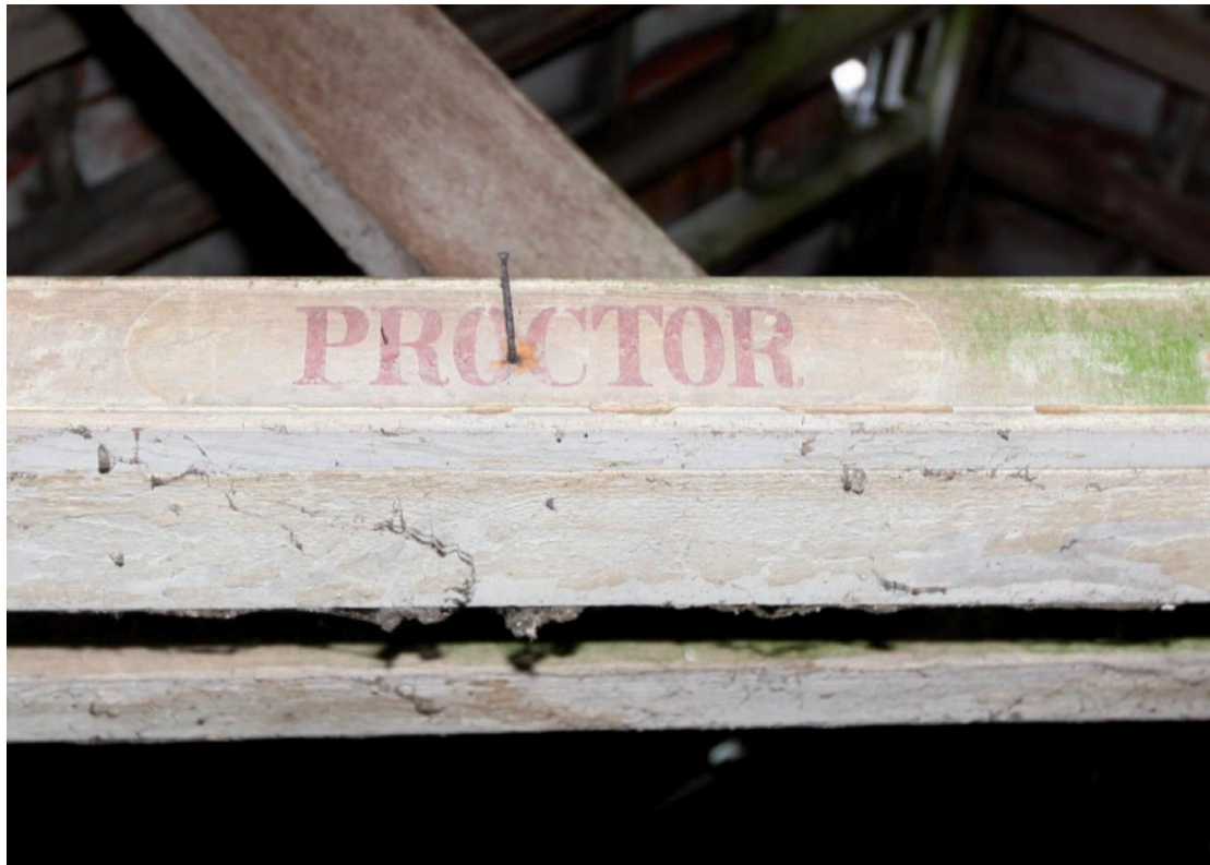
Illus. 15. Detail of the original painted name 'Proctor' on the door lintel of the north-eastern stall of the western stable (5b). The name is picked out in red on a white cartouche with curved ends, but was subsequently covered with whitewash.
