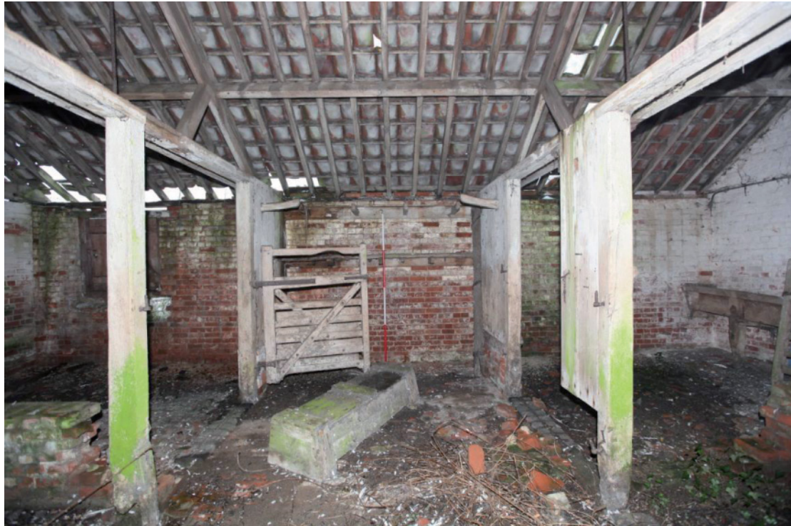
Illus. 11. Interior of the eastern stable (5a) showing its central passage with mutilated stall divisions to left and right. The remains of a boarded manger are visible to the right (in the stall marked Darling) and a window hatch to the left (Diamond), with two tiers of wooden harness hooks in the centre. The stalls in the foreground are named Bonny (left and Brag.
