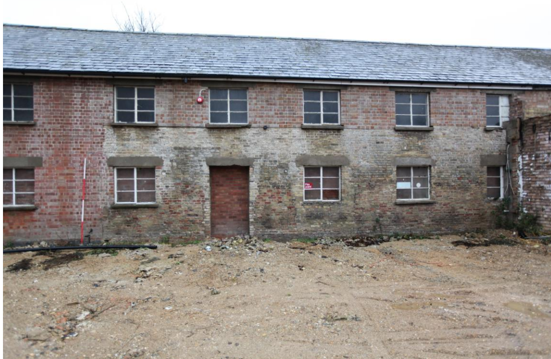
Illus. 5. The western exterior of the malting range (1) showing the remaining original brickwork to the right with 20th century Fletton brickwork above & left. The metal-framed Crittall windows date only from the building's extensive mid-20 th century refurbishment which appears to have included the raising of its walls.
