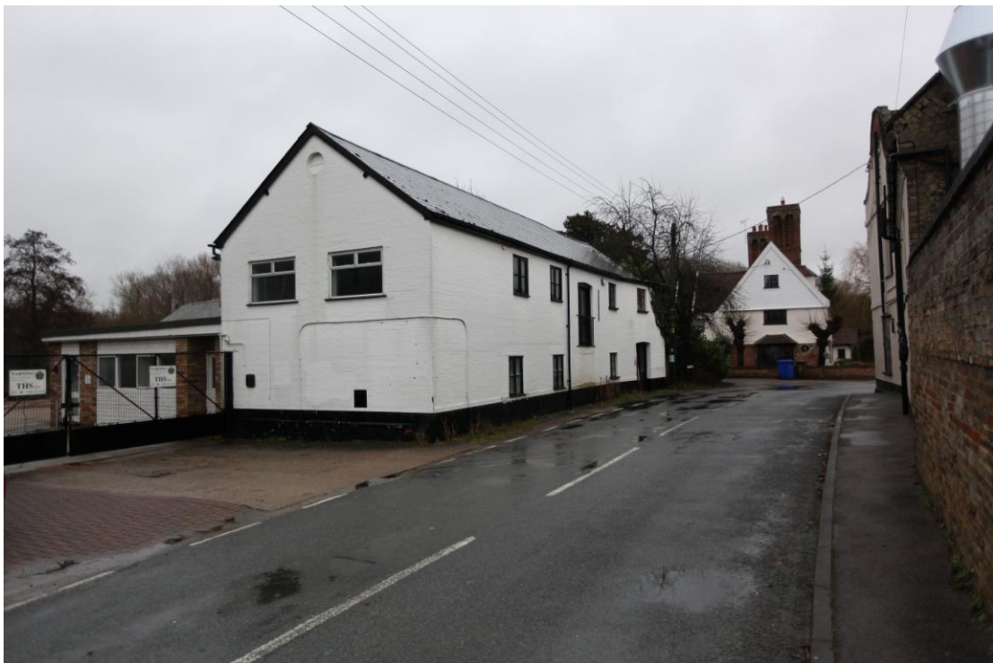
Illus. 2. The maltings from The Street to the west showing the late-19 th century roadside range of painted brick (2 & 3) with the 20 th century offices (4) to the rear (left).
