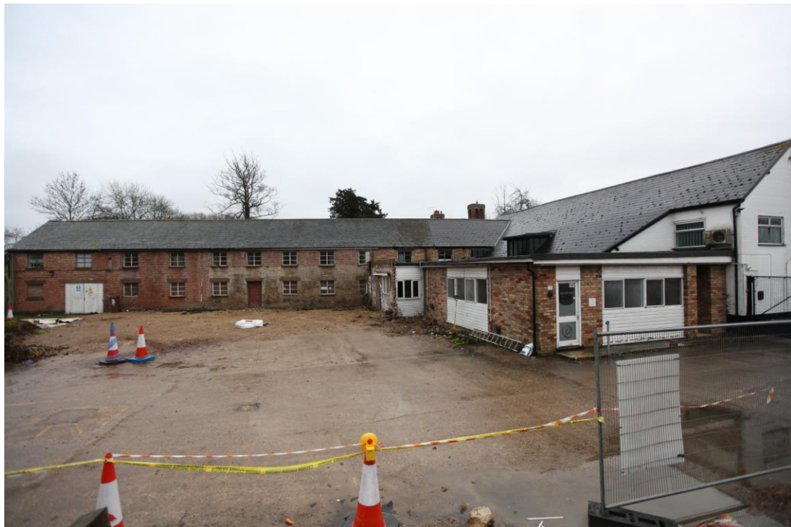
Illus. 4. The maltings from the west showing the 19 th century street range (2 & 3) with the 20 th century flat-roofed offices (4) to the right, and the much altered 18 th century brick malting range (1) to the left.
