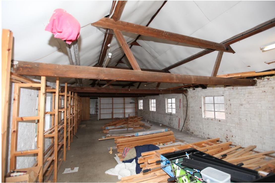
Illus. 11. The upper storey of the malting range (5b) from the north showing the 20th century softwood roof trusses and exposed brickwork of the external walls. Both the front and rear elevations have been raised by varying degrees, and the western elevation to the right largely rebuilt.
