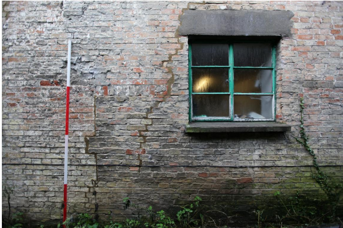
Illus. 7. Detail of the eastern external elevation of the malting range (1) showing its northernmost window (lighting the modern stair lobby, 1e) with evidence of a blocked original low door or window between it and the scale bar to the left. Note the straight joint respected by closers (quarter bricks) and the horizontal lintel of bricks set on edge (at the same height as the lower glazing bars).
