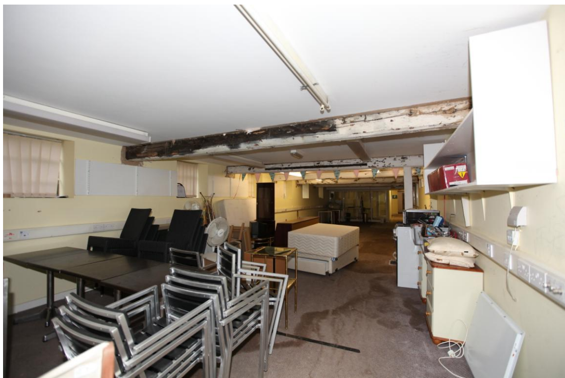
Illus. 10. The interior of the malting range (1) from the north showing the recently exposed and ostensibly original chamfered binding joists (with early grey pigment beneath later whitewash). The internal walls and common joists are concealed by late-20 th century dry-lining.
