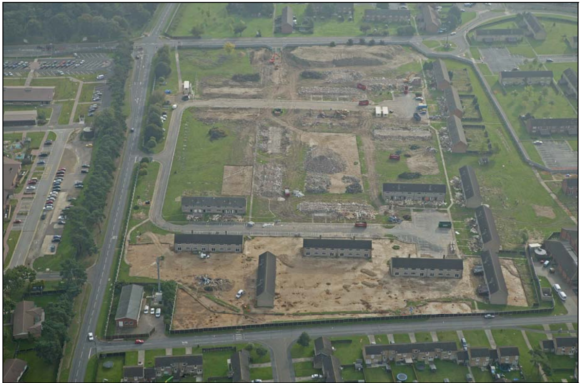
Plate 1. Liberty Village Phase I, facing east with ERL 147 in foreground
