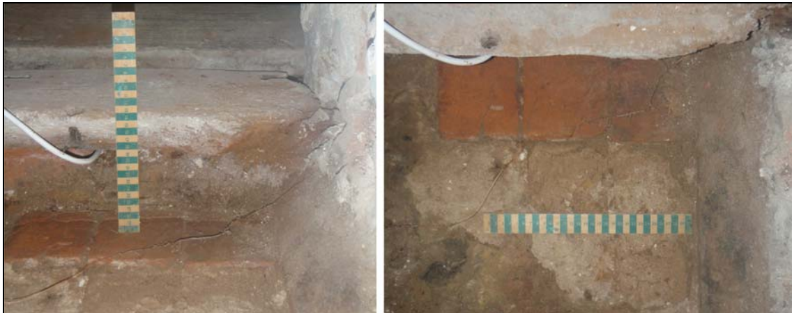
Figure 4. Tiled floor against dressed stone foot of the tower arch
