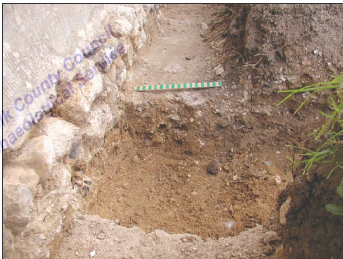
Plate 1: nave wall test-pit & stepped footing
