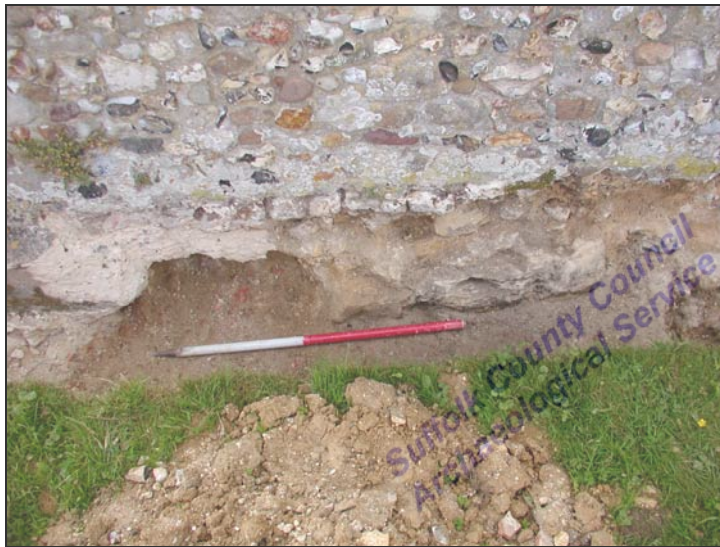
Plate 2: chancel, sandstone boulder in stepped footing
