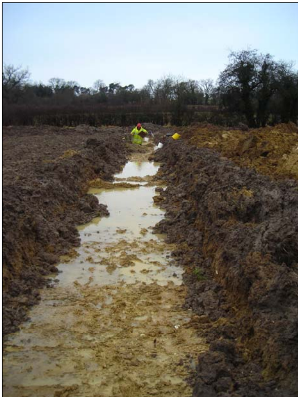
Plate 1. Trench 1, looking west
