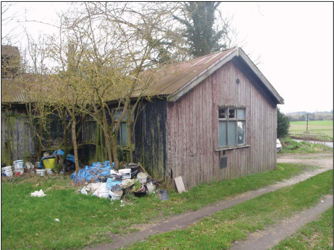
Plate X. The Sunday School, camera facing south-east (ref. HGK 79)
