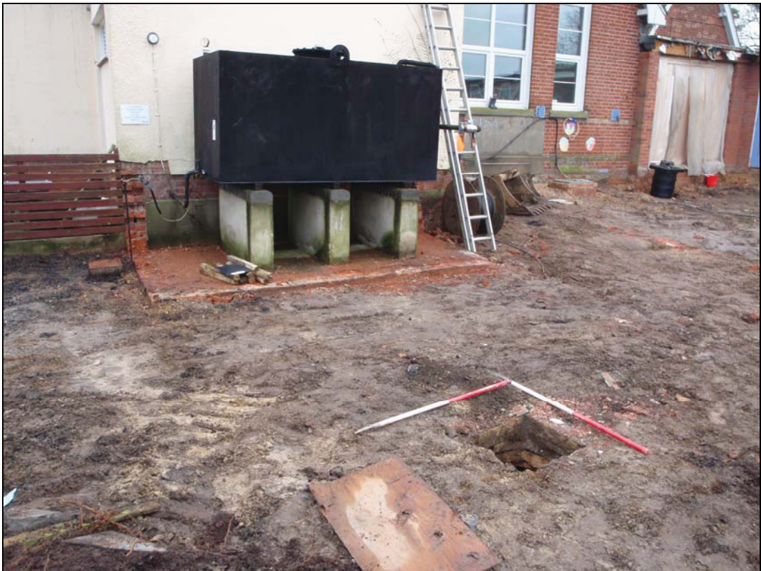
Plate IV. soakaway (S1) in the foreground, camera facing east
