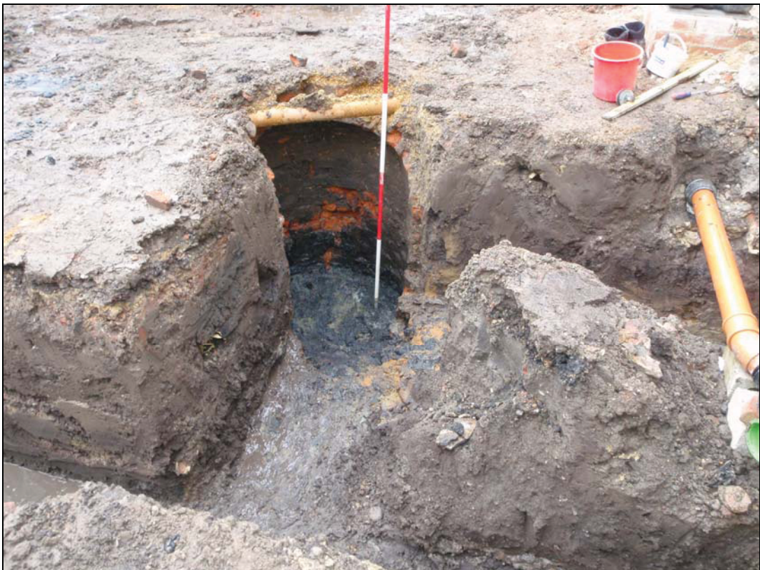
Plate II. foundation trenches with soakaway S2 in the background. Ditch 0002 runs from left to right. (camera facing north-west)
