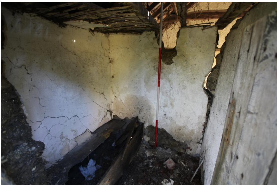
Illus. 8. The interior of the privy (1) from its western entrance showing the whitewashed walls and decayed lath-and-plaster ceiling with the remains of two chamfered circular apertures in the damaged boarded seat to the left.
