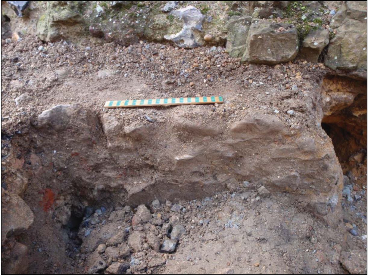
Plate 1. Poor House foundation, facing south-west
