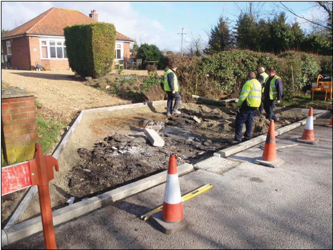
Plate I. improvement works to the site access road
