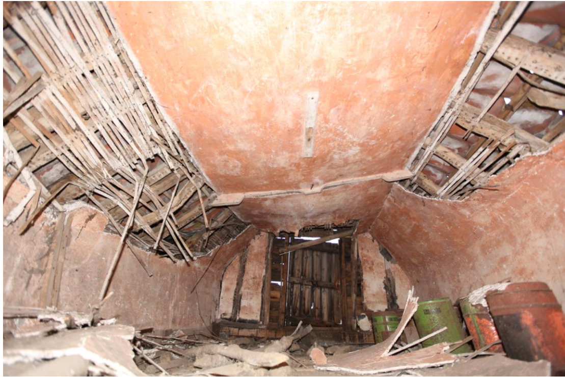
Illus. 15 Interior of the first-floor granary (2) seen from the south, showing the loading door in the northern gable and its 19 th century lath-and-plaster with unusual red ochre pigment. Most interiors of this kind were whitewashed.
