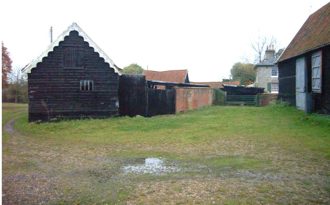
Illus. 3 The site from the south-west, showing the stable (4) to left and the barn (5) right with the granary (2) and house (7) in the rear
