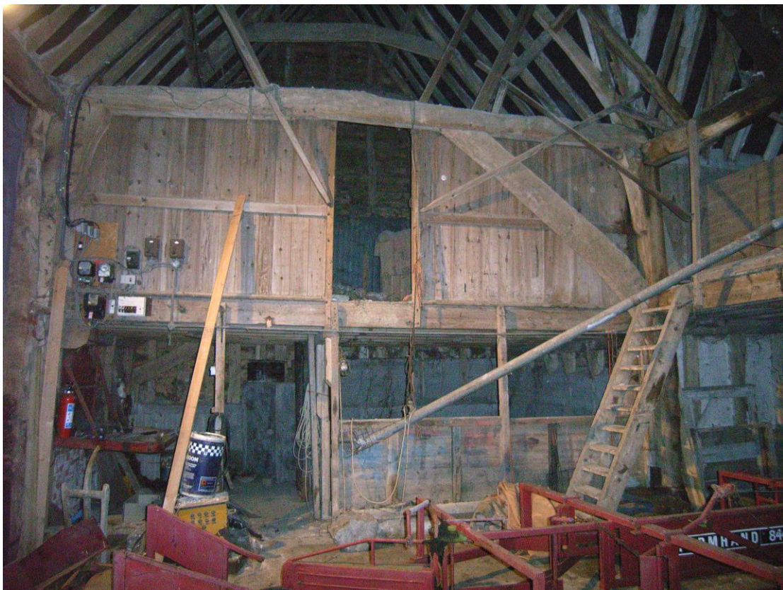
Illus. 12 Interior of barn (5) from south, showing the 20 th century granary and milling floor in the northern bay, with an original arch brace to the right
