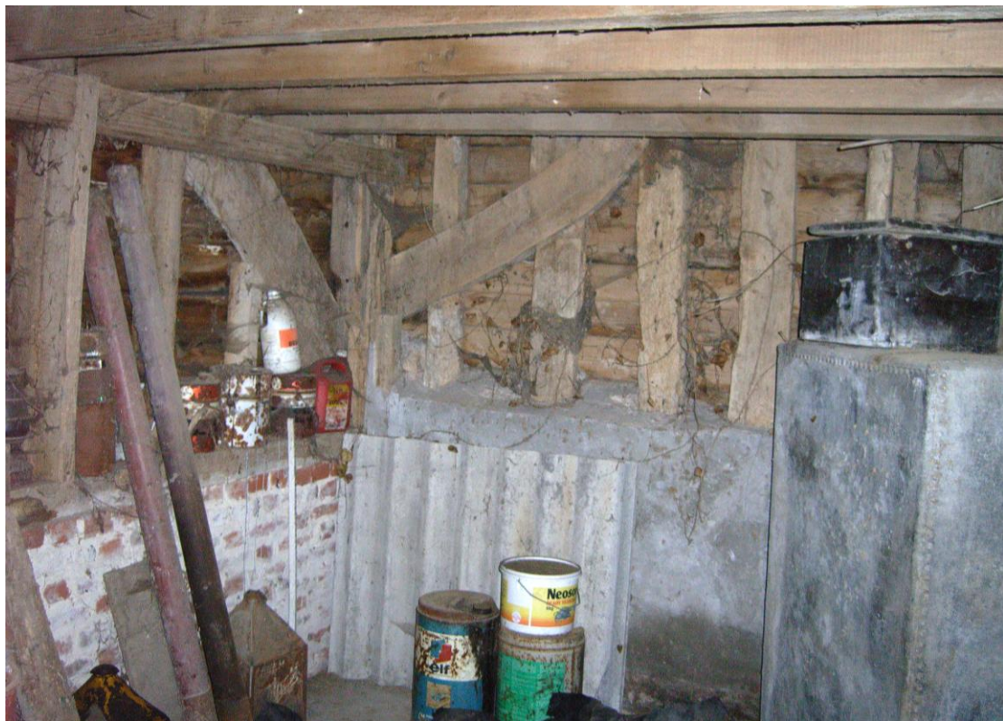
Illus. 14 Detail of the barn (5) showing the curved primary braces in its north-eastern corner – largely hidden by the later granary ceiling and shuttering. Far more of the original structure would be revealed if these later insertions were removed
