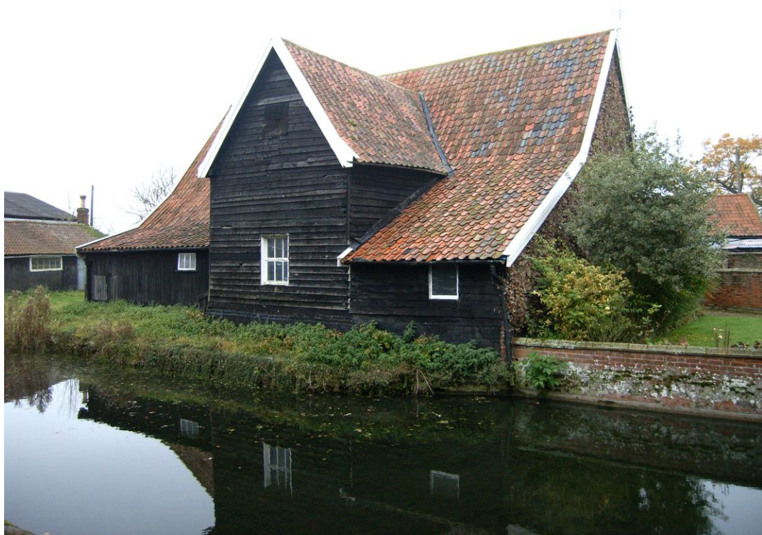
Illus. 1 The 17 th century barn (5) from the south-east, showing the 19 th century pantiled roof
