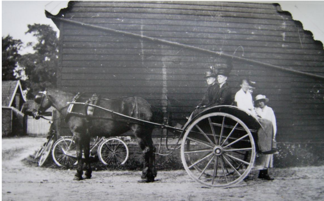
Illus. 5 Southern gable of the barn (5) in an early-20 th century photograph, showing its distinctive Victorian Mock-Gothic barge-boards with the granary (2) visible to left
