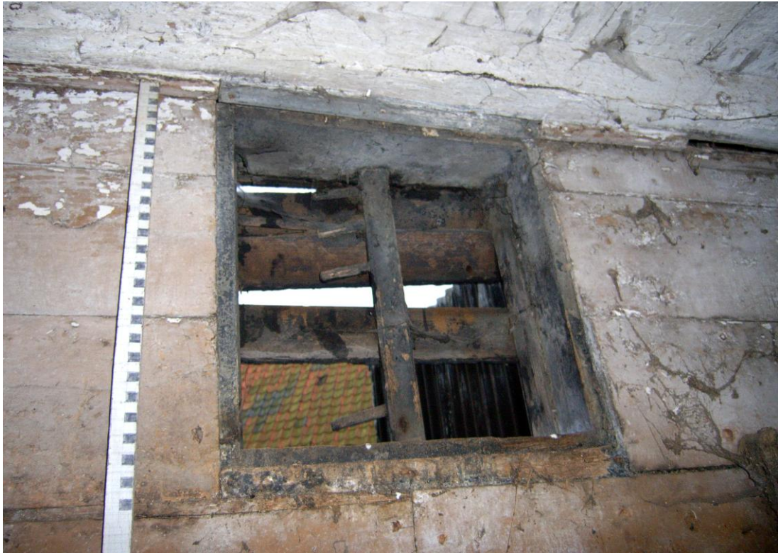
Illus. 11 Detail of the 19 th century shuttered window in the stable (4), the shutters of which could be opened or closed by revolving the central mullions (centimetre scale)
