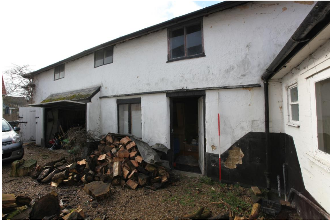
Illus. 5. The cement-rendered eastern exterior seen from the house to the north-east showing the late-20 th century garage door (2) to the left and the door to the bakery (3) to the right with an adjacent fragment of exposed clay lump.
