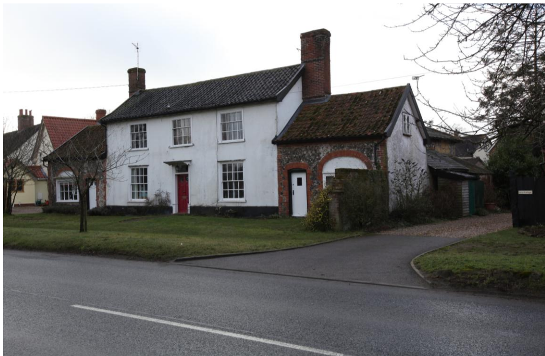
Illus. 2. Exterior of Kent House from the north-east showing the flint-rubble sometime Baker's shop to the right and the identical sometime butcher's shop to the left. The northern gable of the clay-lump outbuilding with its lean-to shed (4) is visible to the extreme right where it adjoins the drive of the neighbouring property (Fox Cottage).
