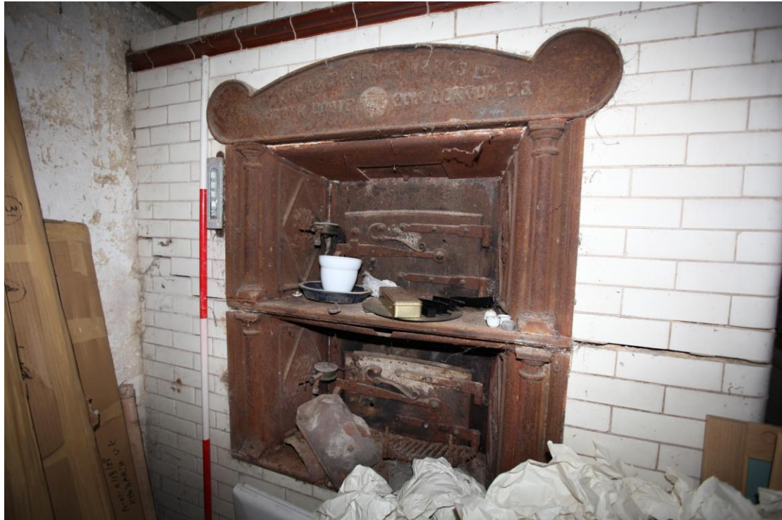
Illus. 9. The iron doors and decorative surround of the bread oven in the bakery (3) showing its cast wheatsheaf ornaments and the superscript 'Kent & Co. Globe Works Ltd. South Grove Bow London E3'.
