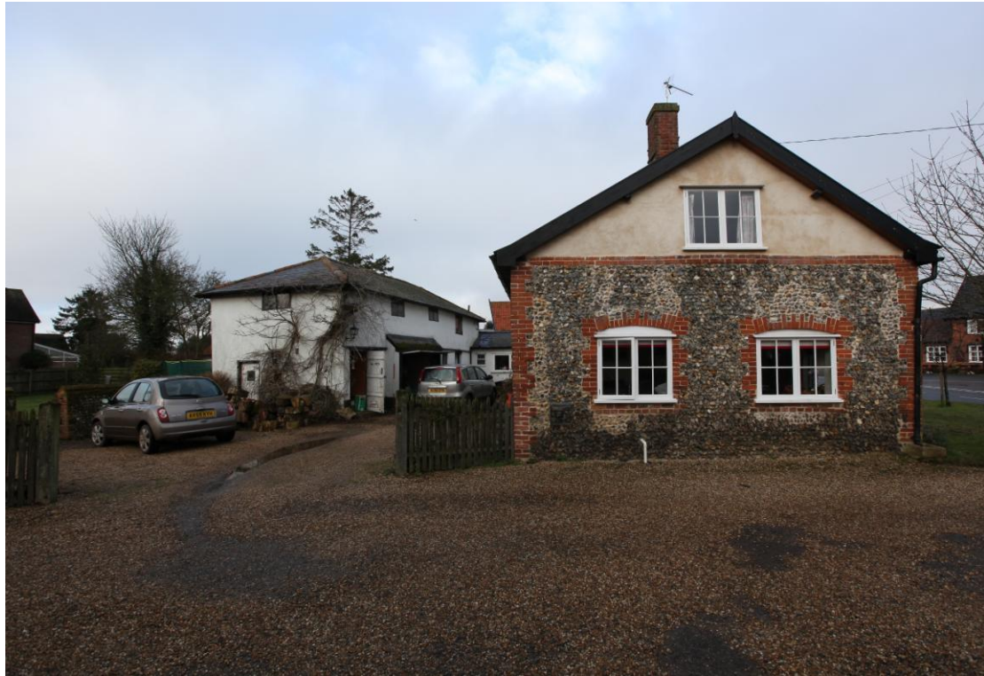
Illus. 3. General view of the site from the south-east showing the clay-lump outbuilding in the rear to the left and the gable of the flint-rubble sometime butcher's shop (now the kitchen of Kent House) to the right.
