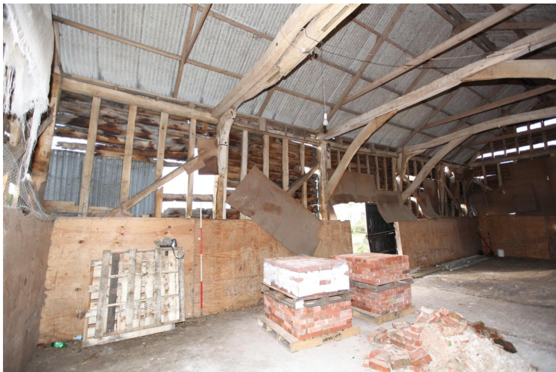
Illus. 10. The southern interior of the barn (1) showing the low doors of the central threshing bay to the right (replacing original full-height entrance doors in the same position).
