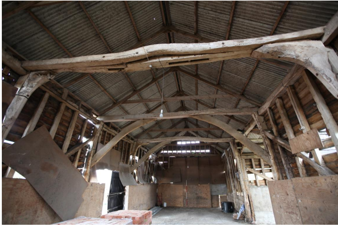
Illus. 9. The interior of the barn (1) from the east showing its 20 th century rebuilt roof with the re-used tie-beam and original knee-braces in the foreground.
