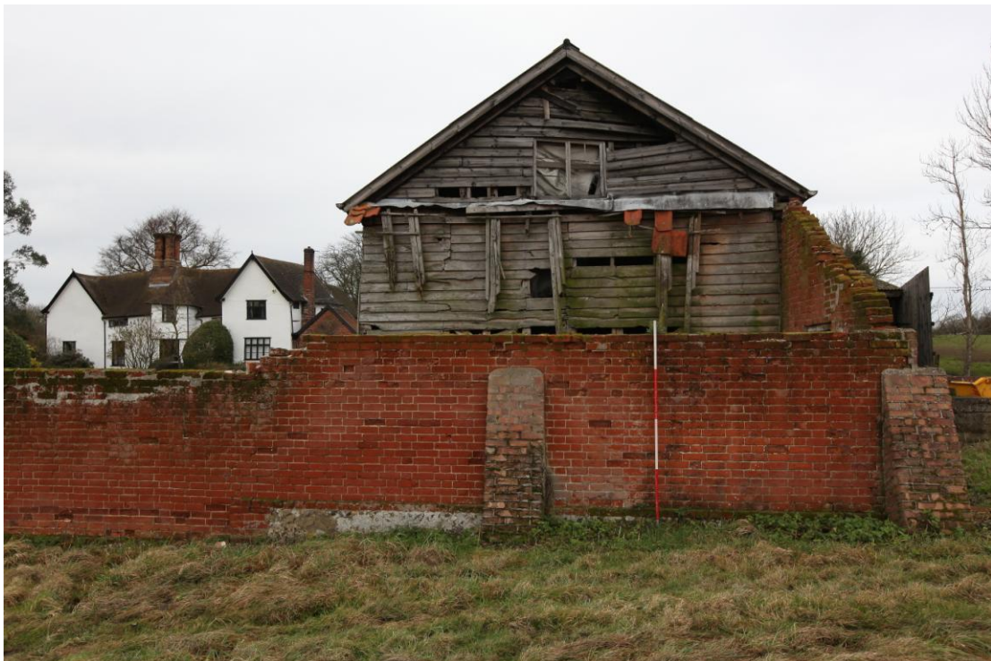
Illus. 8. The eastern external gable of the barn (1) showing the hanging rafters of a demolished lean-to shed with the wall of the yard (3) in the foreground.
