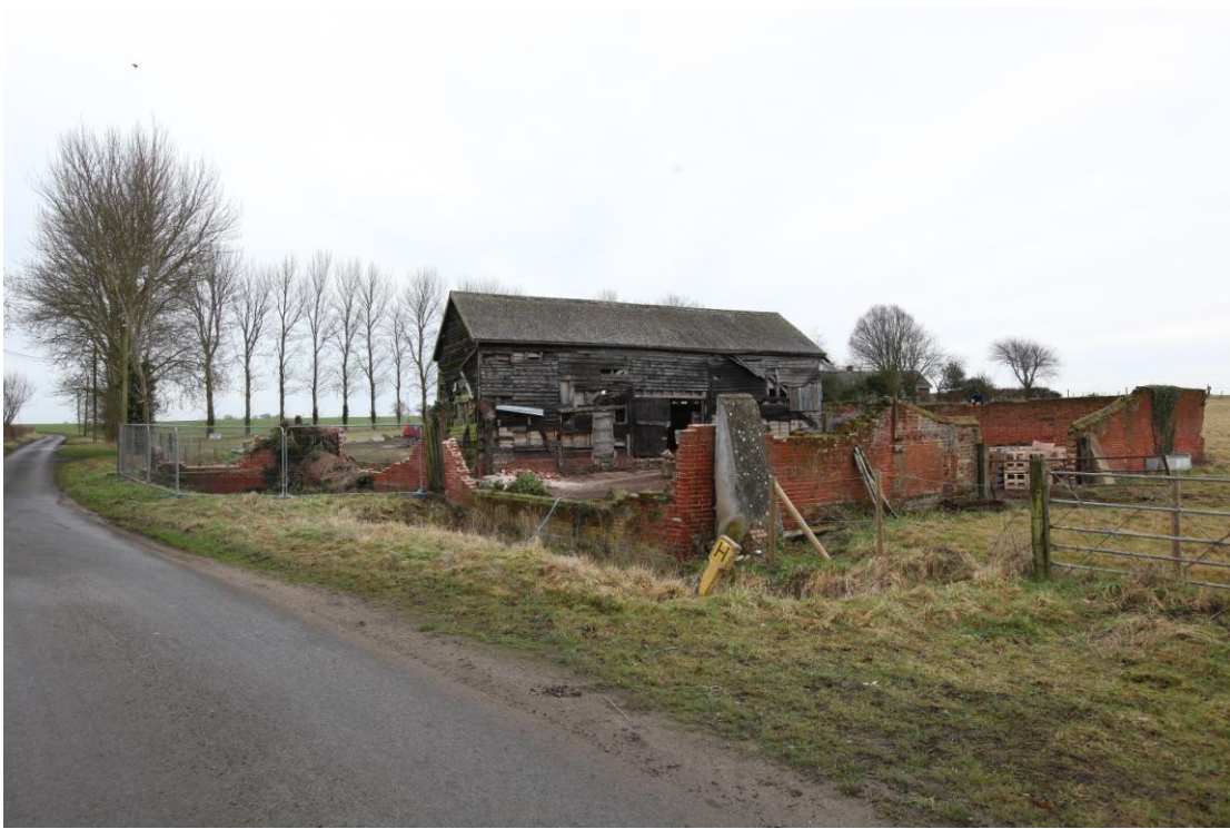
Illus. 3. The exterior of the barn and yard complex from Clockhouse Lane to the south-west, showing the extent to which the yard walls had been demolished at the time of inspection.
