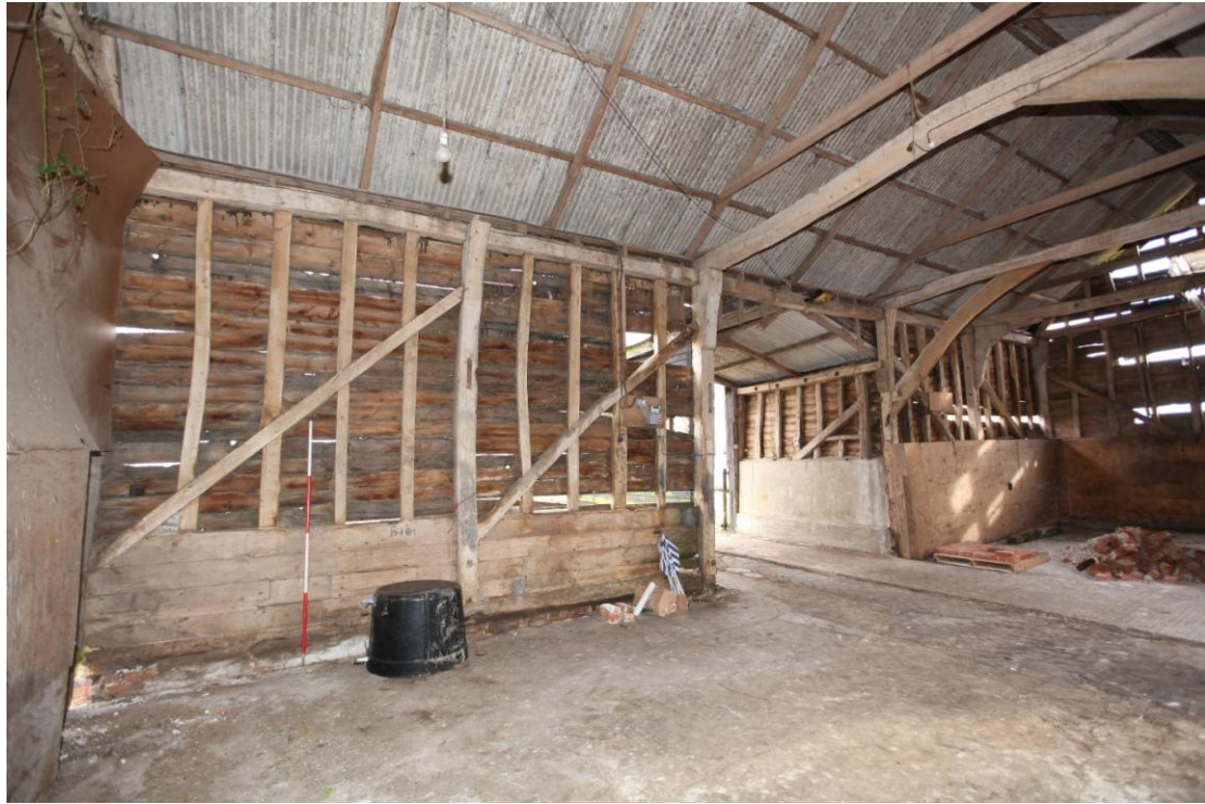
Illus. 11. The northern interior of the barn (1) from its south-western corner showing the original porch of the central bay and the straight, diagonal primary wall braces.
