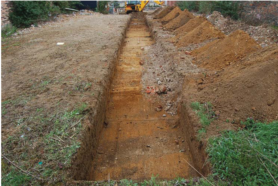
Plate 1. Trench 1, facing north-east (2m scale).
