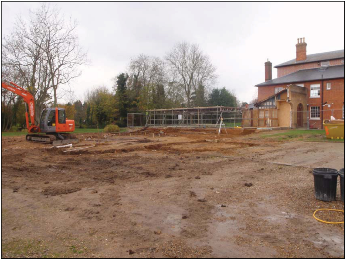
Plate I. general view of the area of the development (camera facing south)
