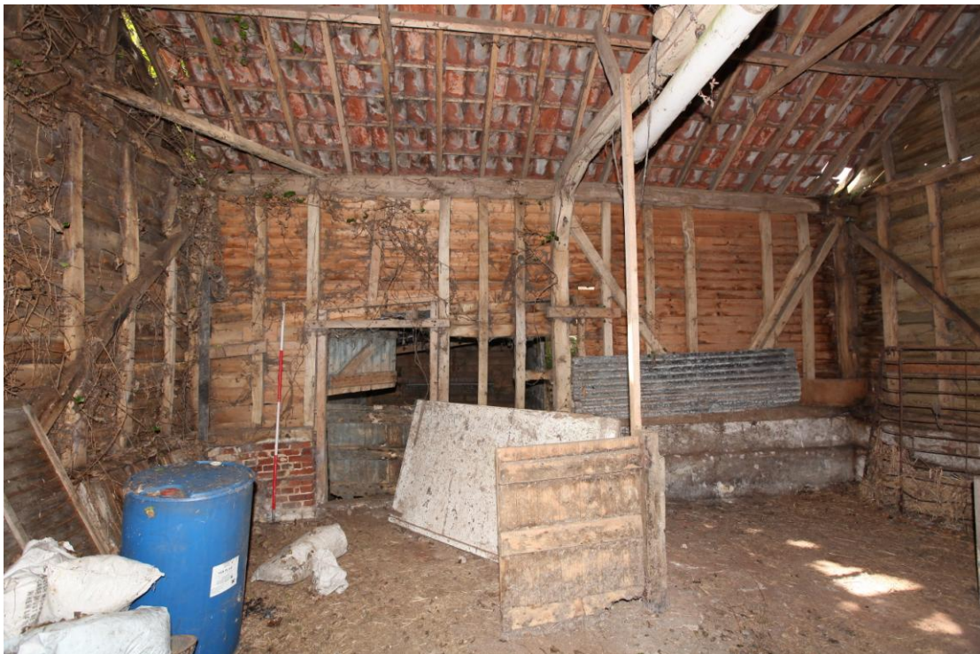
Illus. 4 The western interior of the two-bay barn (1) showing its original small rear doorway to the left with a section of exposed red-brick plinth. The oak studs respect the door, and the ground sill is tenoned and pegged to its jamb.
