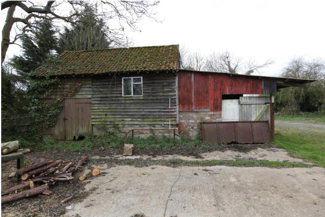
Illus. 3 The eastern exterior of the barn (1) showing its principal entrance doors (reduced in height) to the left and the open shed (5) to the right.
