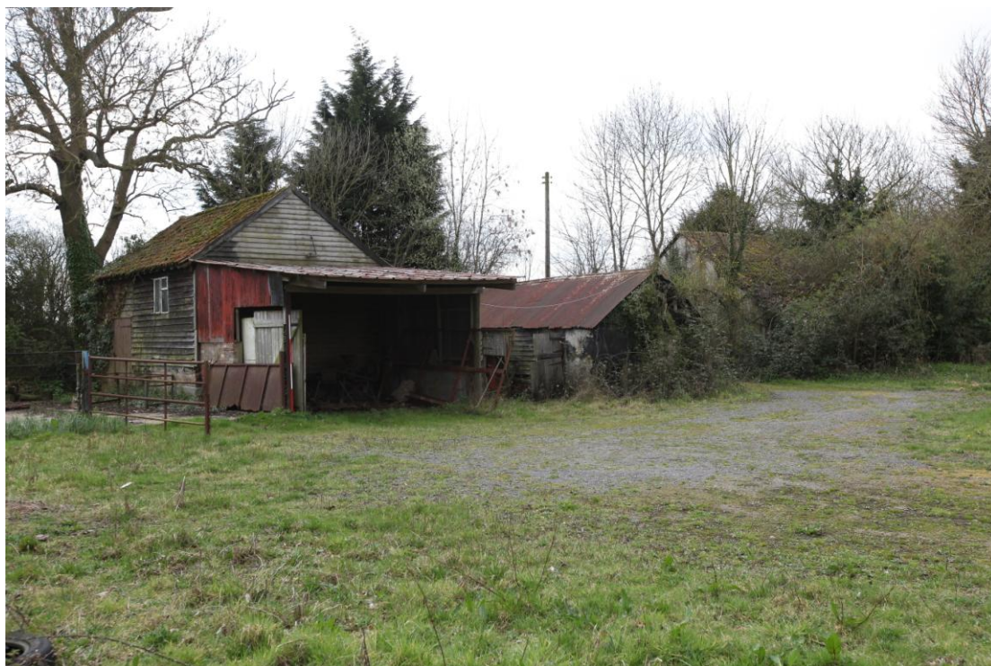
Illus. 2 The exterior of the barn complex from the north-east showing the barn (1) with the open shelter (5) adjoining its northern gable to the left and the clay-lump shed (4) to the right. The former farmhouse is visible in the trees to the rear.
