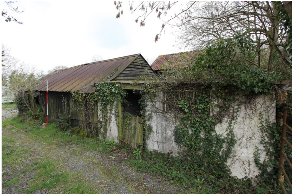
Illus. 7 The western exterior of the clay-lump shed (4) seen from the site entrance to the south-west showing the 20 th century block-work shed (2a) to the right and the studwork addition (3) in the centre.
