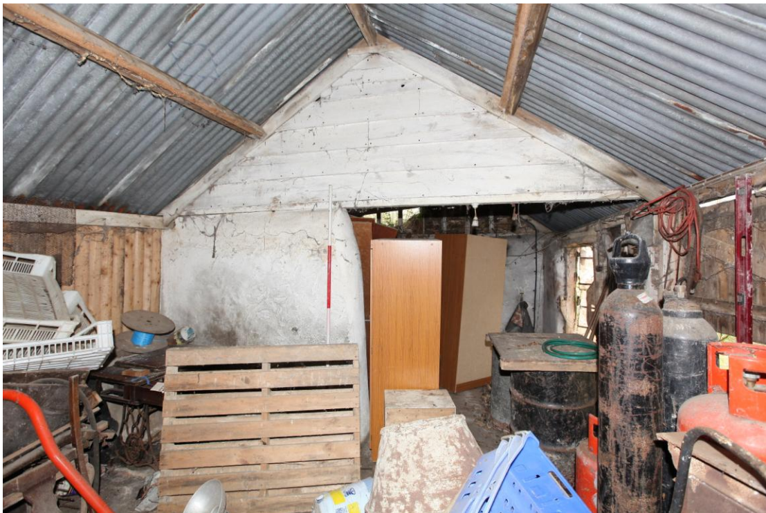
Illus. 10 The southern exterior of the clay-lump shed (4) as seen from the adjoining studwork shed (3) showing its boarded roof-gable and original clay-lump fabric to the left. The right-hand section of the gable has been removed to link the two sheds.
