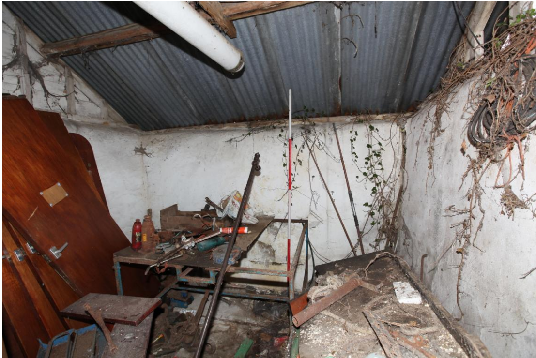
Illus. 9 The western interior of the clay-lump shed (4) showing its cement-rendered walls and 20th century corrugated iron roof.
