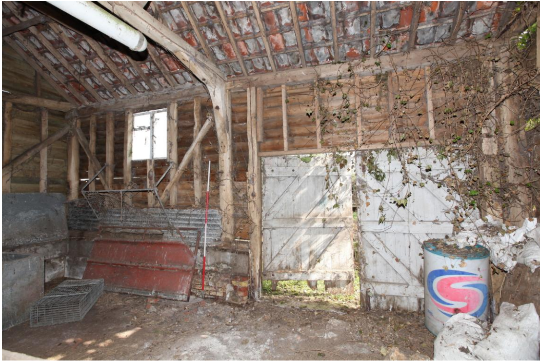
Illus. 5 The eastern interior of the barn (1) showing the position of the original full-height entrance doors to the right. The present doors and the narrow softwood studs above were inserted in the 20 th century (along with the roof structure and section of roof-plate immediately above) but the jambs to left and right are original features.
