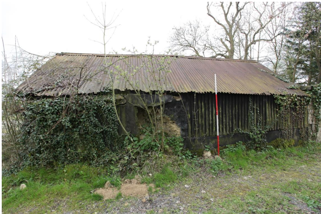
Illus. 8 The western exterior of the clay-lump shed (4) showing its tarred daub with the vertical boarding of the studwork addition (3) to the right. A section of decayed clay-lump fabric is exposed to the left of the scale.
