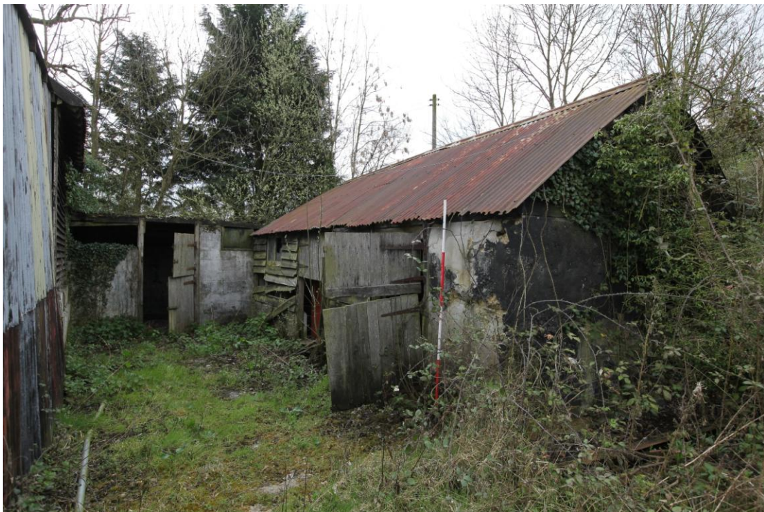
Illus. 6 The narrow central yard from the north showing the barn (1) to the left and the clay-lump shed (4) with its later southern extension (3) to the right. The 20 th century cement-block shed (2b) is visible in the rear.
