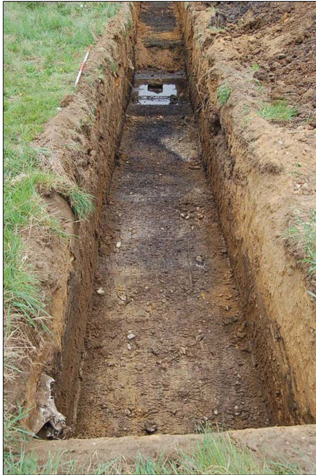
Plate 4. Trench 4 facing south-east (2m scale)
