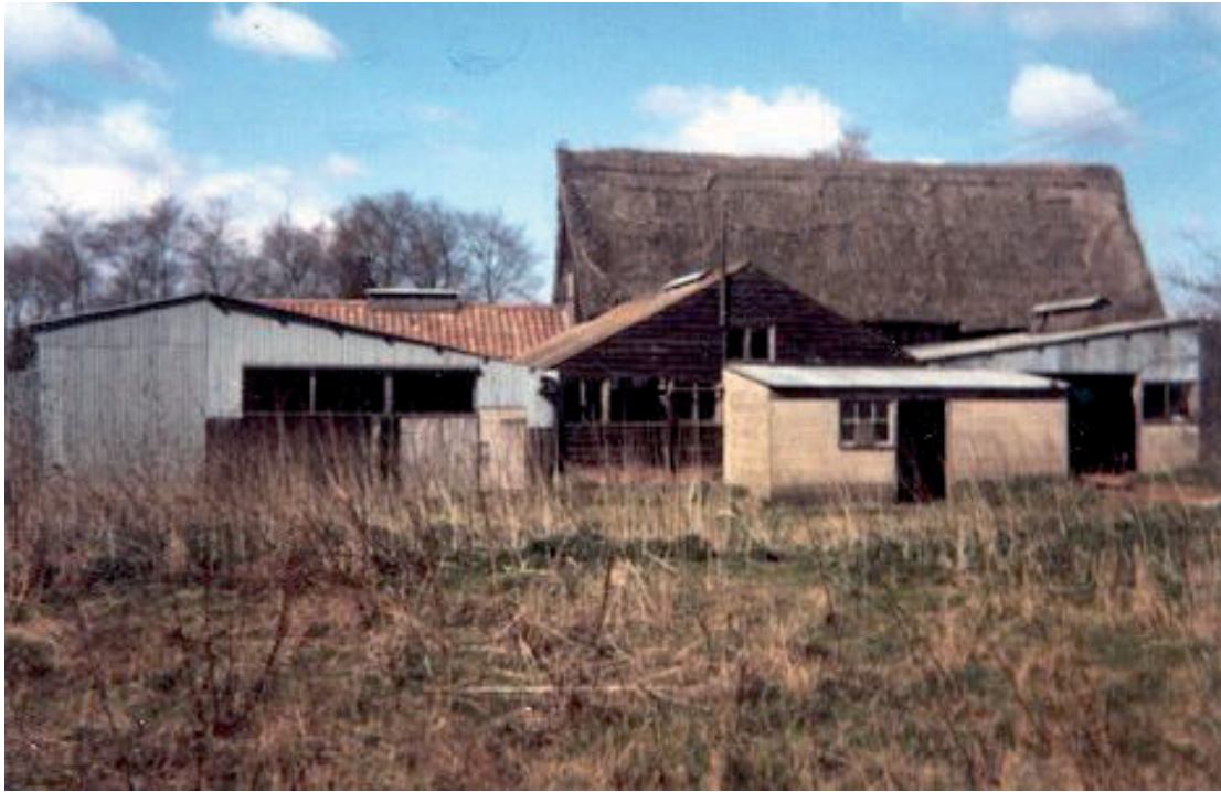
Illus. 1 Circa 1974. The farm buildings from the east showing the original thatched roof of the barn (1) in the rear to the right and the pantiled roof of the southern shed (4) to the left. From an old photograph in the possession of the current owner.
