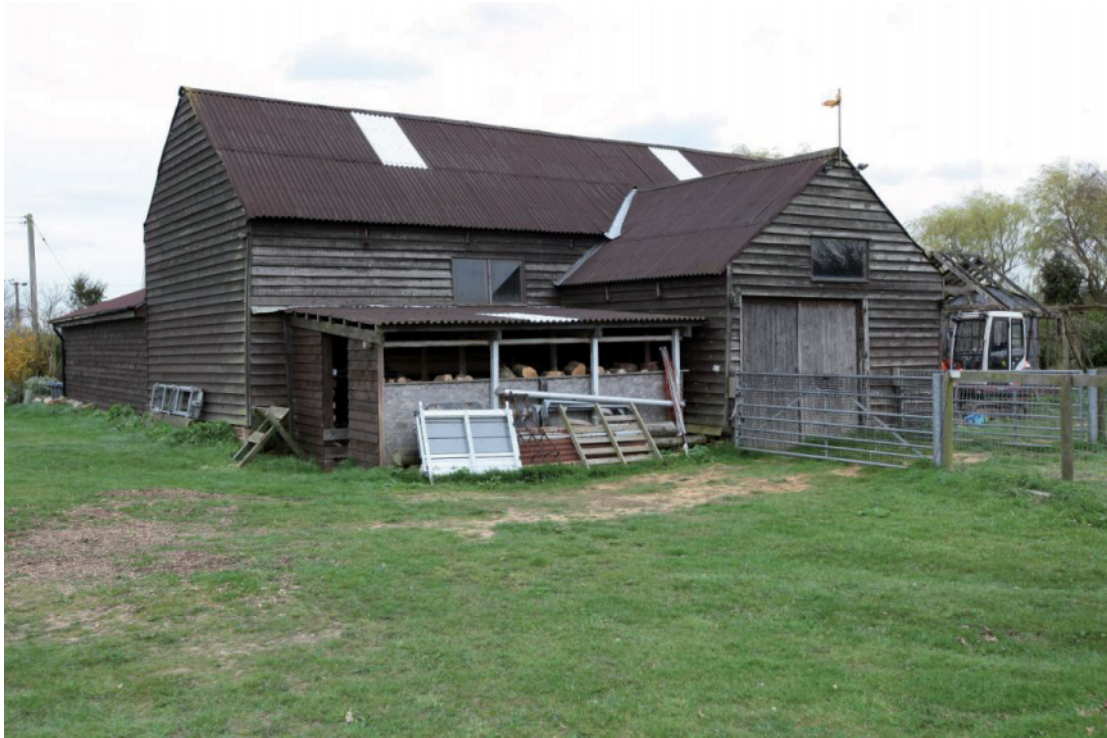
Illus. 5 Exterior of the barn (1) from the north-west showing the modern lean-to woodshed (3) to the left & the 19 th century porch (2) to the right.
