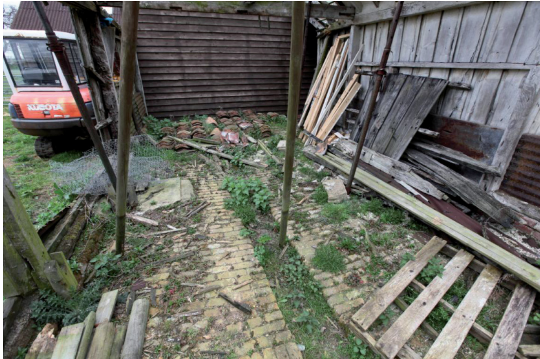
Illus. 7 The interior of the southern shed (4) from the south showing the axial drain in its original gault-brick floor.
