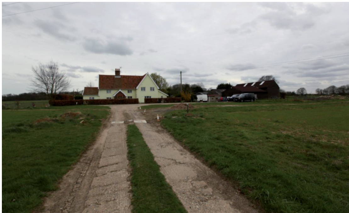
Illus. 4 General view of the site from 20th century entrance leading from the main A12 to the north showing the unlisted farmhouse with an early-17th century parlour to the left and a late-20 th century cross-wing to the right. The barn is shown to the far right. The track which passes from left to right in front of the house marks the boundary between Farnham and Benhall parishes (the photograph taken from Benhall).
