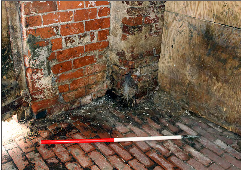
Plate 91. Building 5, interior. Ground floor west side room, south side threshing door. Showing probable recess for a board across threshing door. View looking north-northeast
