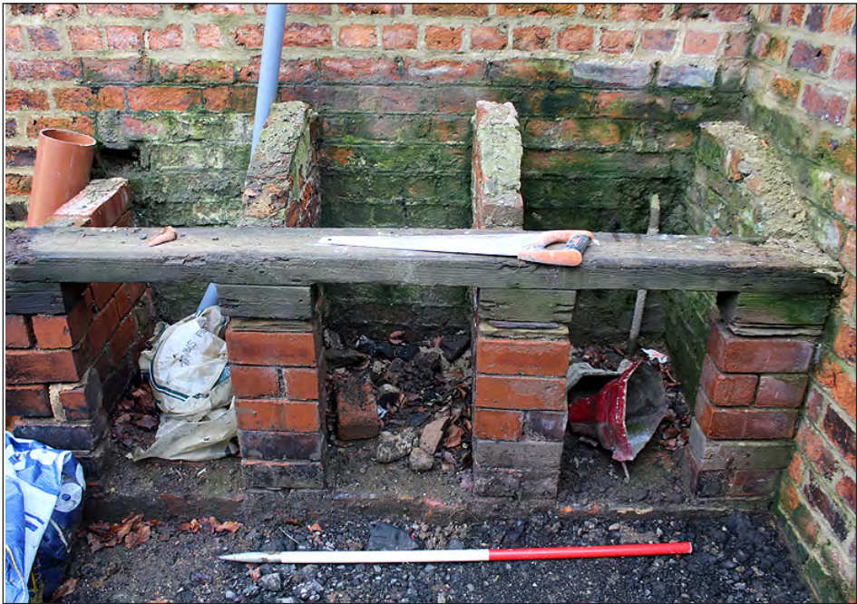
Plate 68. Structure against coal shed. View looking north-northwest
