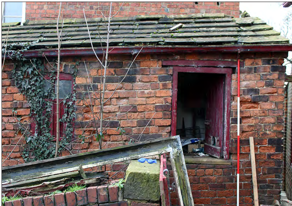
Plate 226. Building 11. North end of the east elevation. View looking west-southwest
