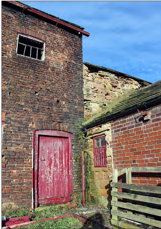
Plate 133. Building 6. West side of the south elevation. View looking north
