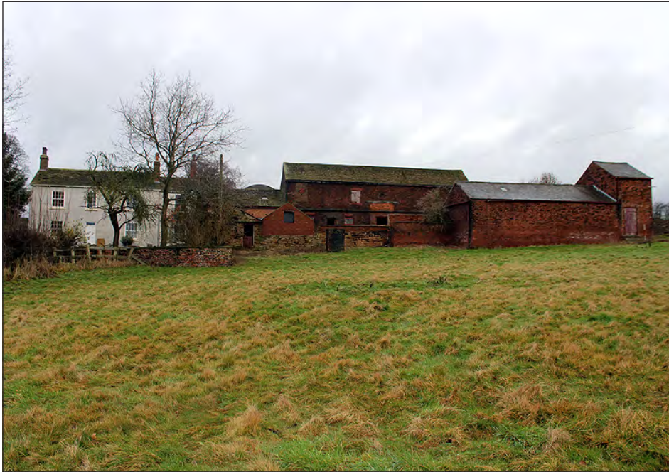
Plate 1. General view of the south side Newsam Green Farm. View looking north
