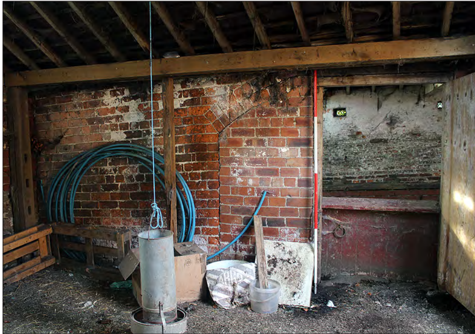
Plate 201. Building 9, interior. West elevation. View looking west-southwest
