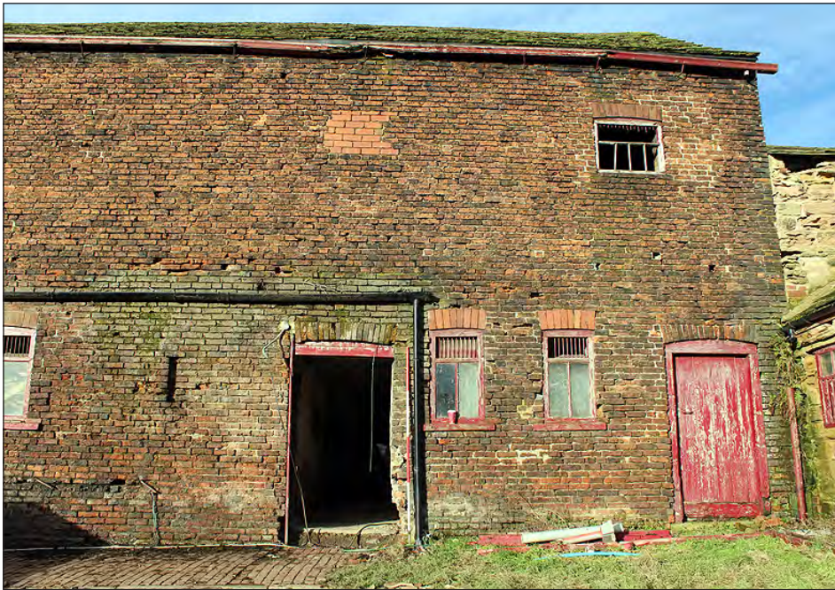
Plate 78. Building 5. East end of the south elevation. View looking north-northwest
