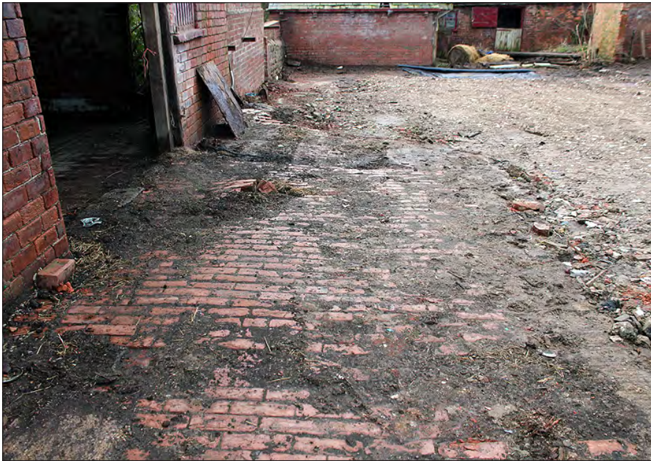
Plate 238. Yard brick surface, adjacent to Building 8. View looking west-southwest
