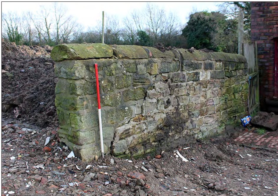
Plate 248. East wall of yard. View looking southeast
