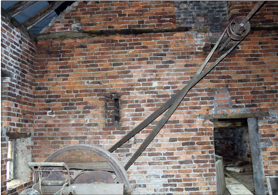
Plate 109. Building 5, interior. First floor, north side of the east elevation. View looking east-northeast
