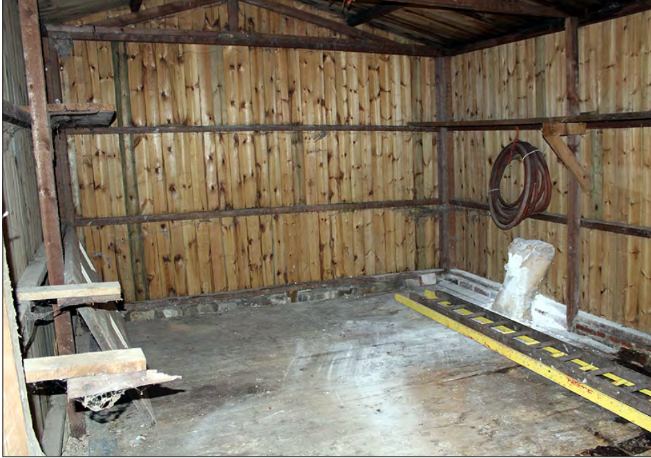
Plate 11. Building 1, interior. View looking northwest
