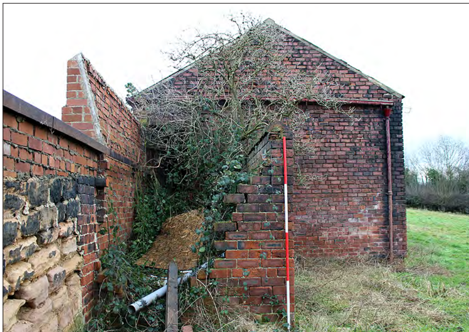
Plate 172. Building 8. West elevation. View looking east-northeast
