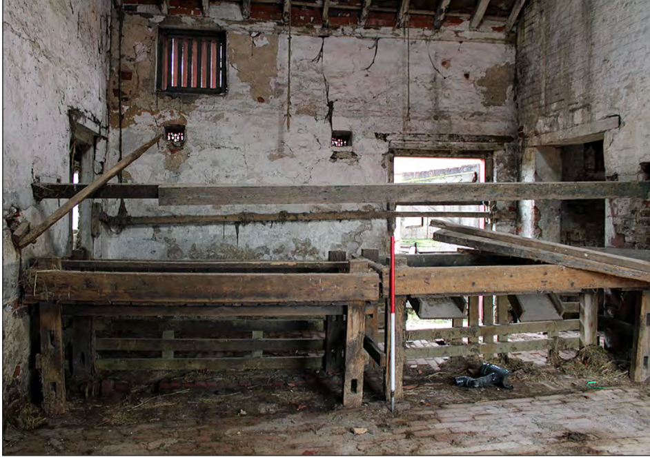
Plate 49. Building 4, interior. East side room. View looking north-northwest
