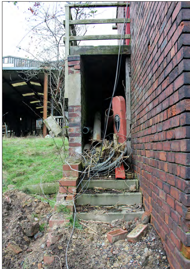
Plate 24. Building 3. West elevation, under stair area. View looking north-northwest
