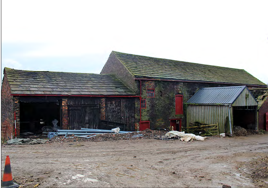
Plate 69. Buildings 5 and 6. North elevation. View looking southwest
