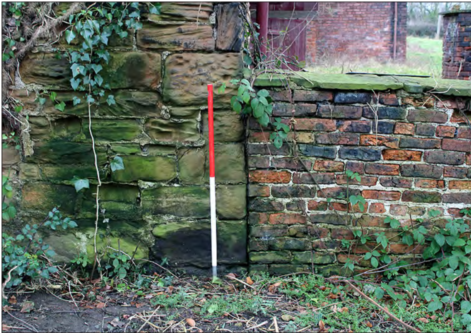
Plate 212. Building 10. Garden wall abutting Building 10. View looking east-northeast
