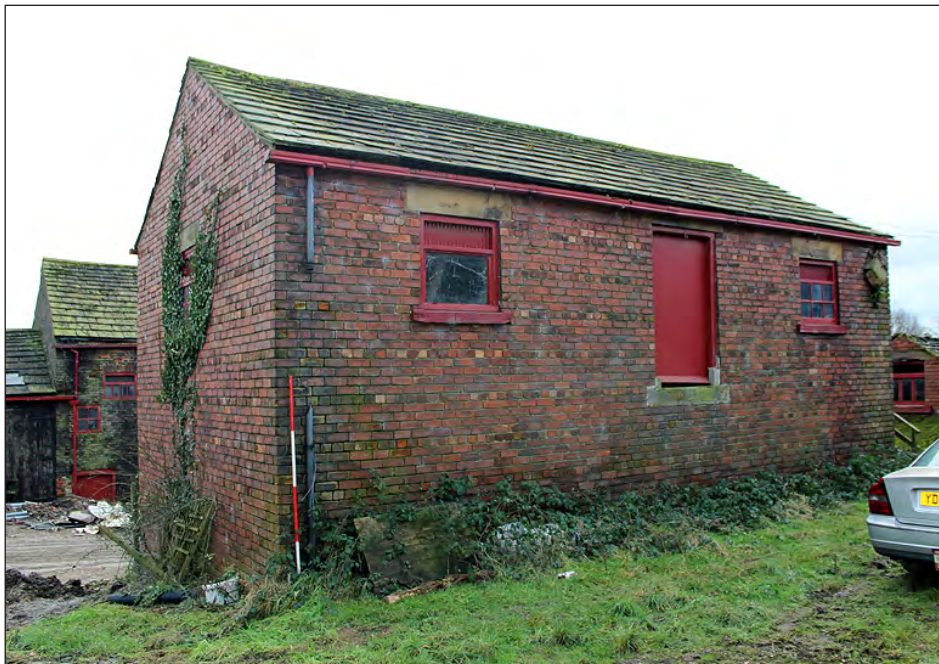
Plate 20. Building 3. North and east elevations. View looking southwest
