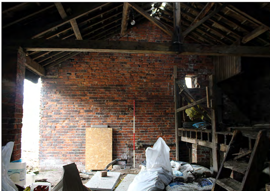
Plate 134. Building 6, interior. East elevation. View looking east-northeast
