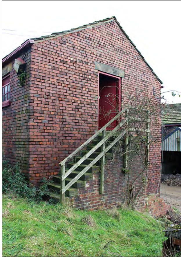
Plate 23. Building 3. West elevation. View looking southeast
