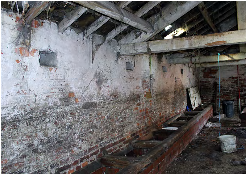
Plate 218. Building 10, interior. West elevation. View looking northwest
