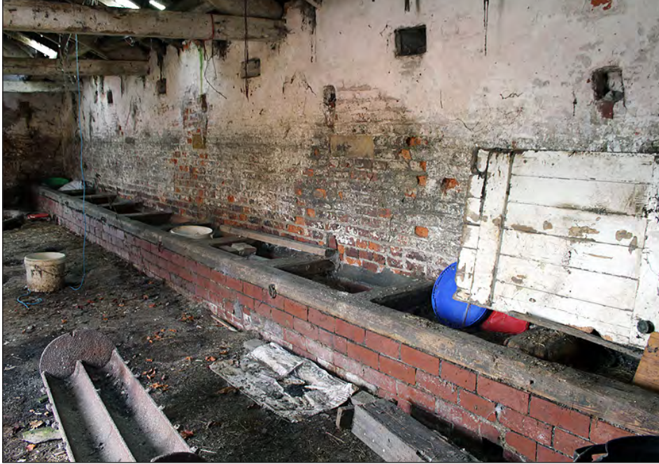
Plate 219. Building 10, interior. West elevation. View looking southwest
