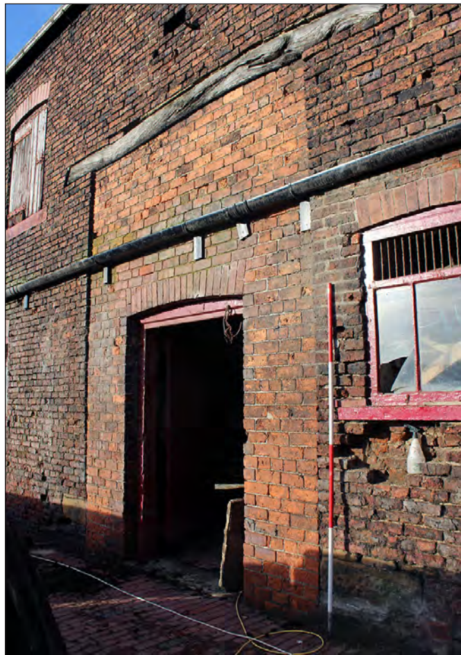
Plate 76. Building 5. South elevation, showing the threshing door. View looking northwest
