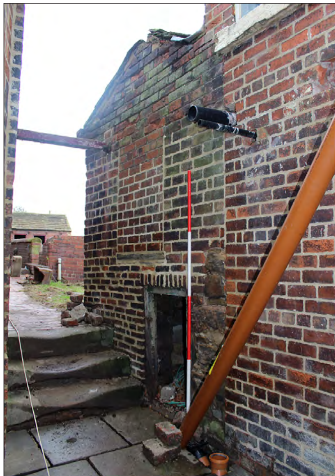
Plate 222. Building 11. North elevation. View looking southeast
