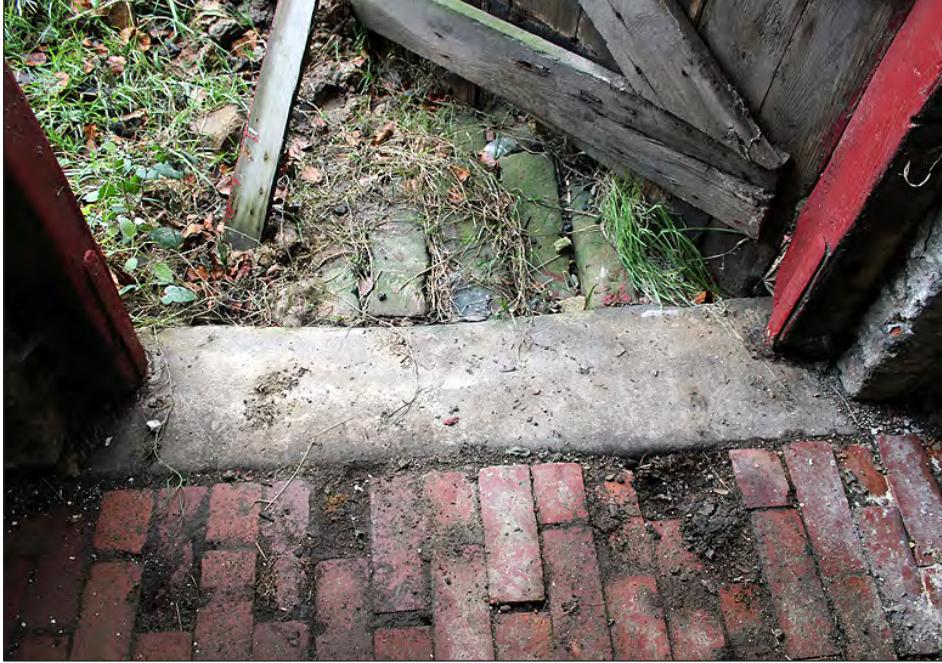
Plate 57. Building 4, interior. Threshold of the east side room. View looking north-northwest
