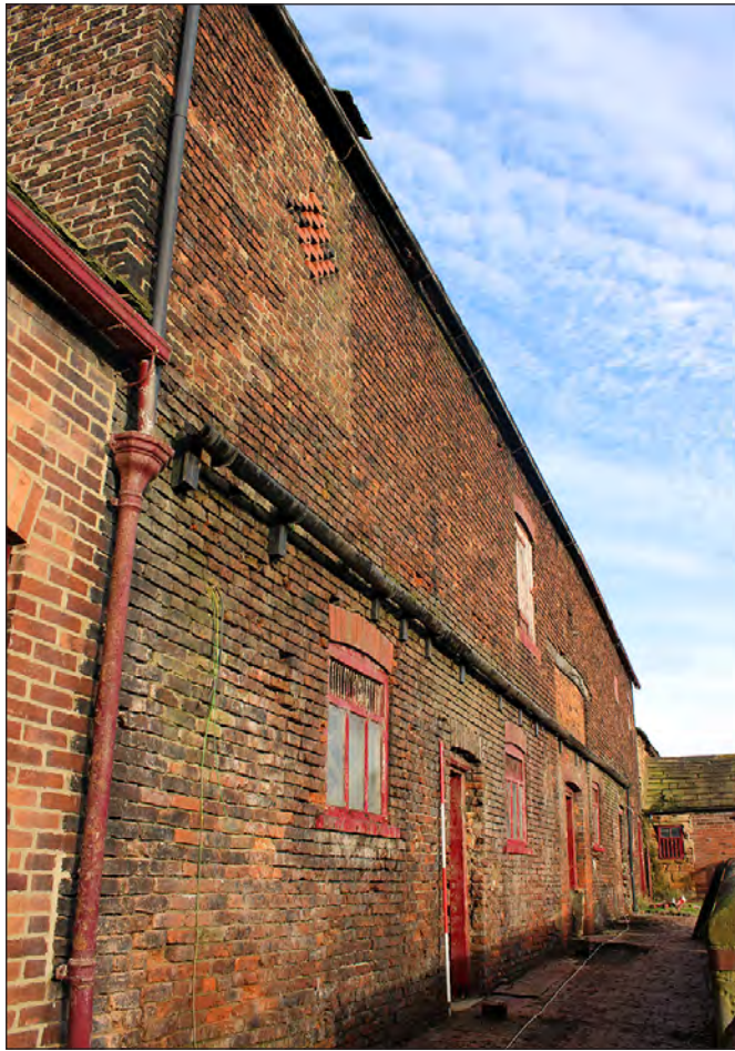
Plate 79. Building 5. View along the south elevation. View looking northeast
