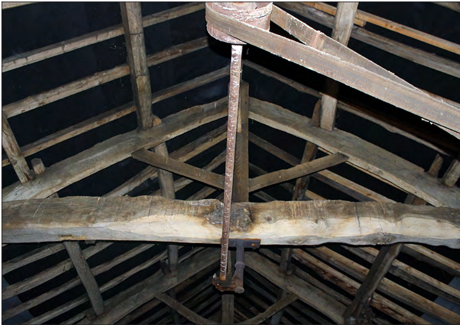
Plate 112. Building 5, interior. Roof truss. View looking east-northeast
