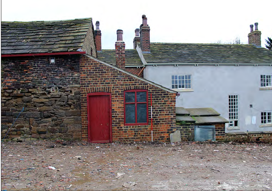
Plate 39. Building 4. West side extension. View looking south-southeast
