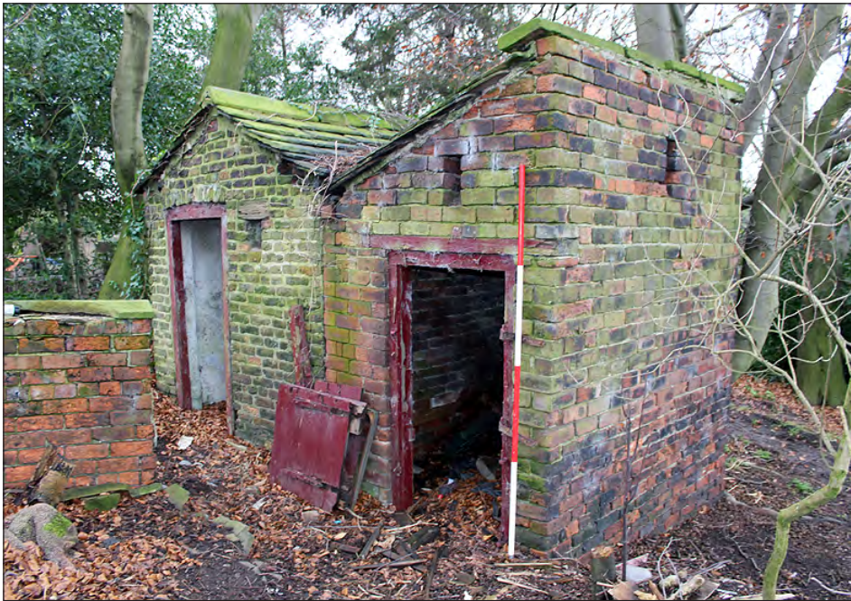
Plate 8. West side outbuildings. View looking southeast
