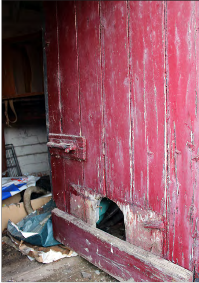
Plate 227. Building 11. Doorway to first floor. View looking southeast
