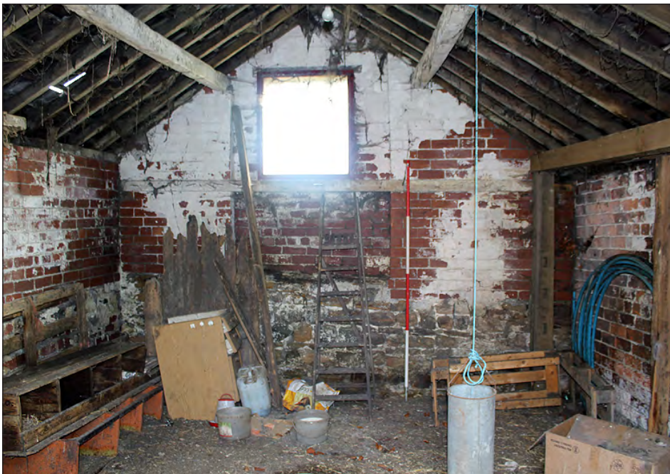
Plate 200. Building 9, interior. South elevation. View looking south-southeast
