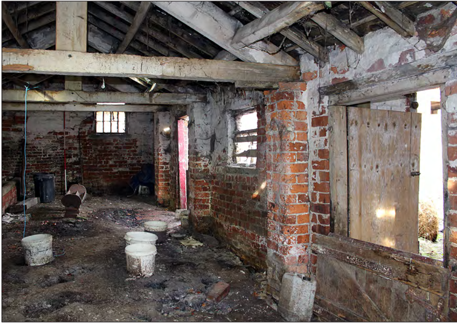
Plate 215. Building 10, interior. North and east elevation. View looking northeast
