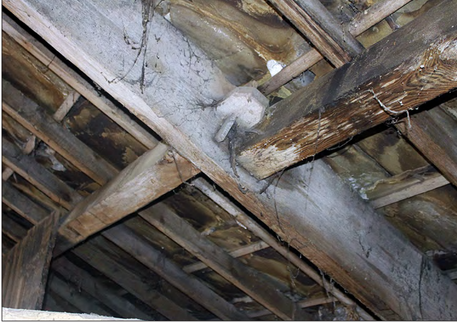
Plate 145. Building 6, interior. Pegged purlins. View looking southeast
