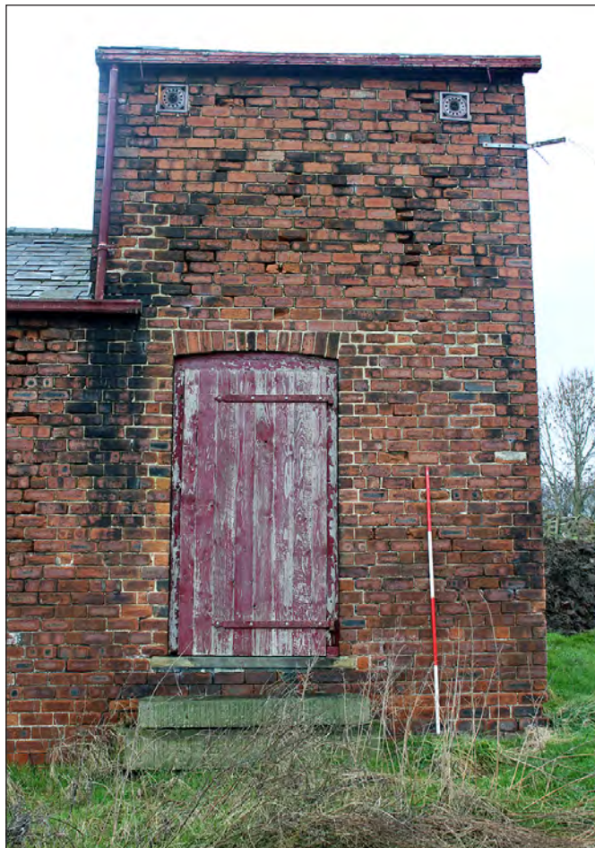
Plate 168. Building 8. East end of the south elevation. View looking north-northwest
