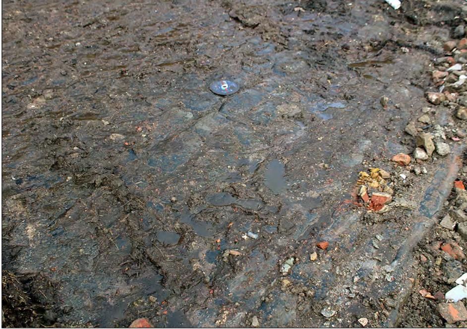
Plate 235. Yard stone sett surface. View looking northeast
