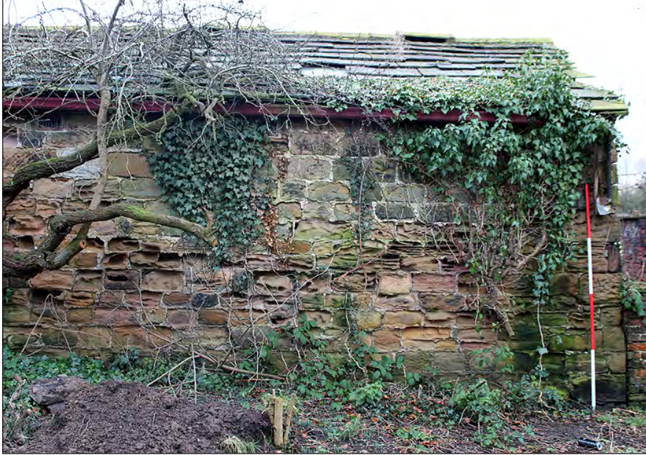
Plate 211. Building 10. South end of west elevation. View looking east-northeast
