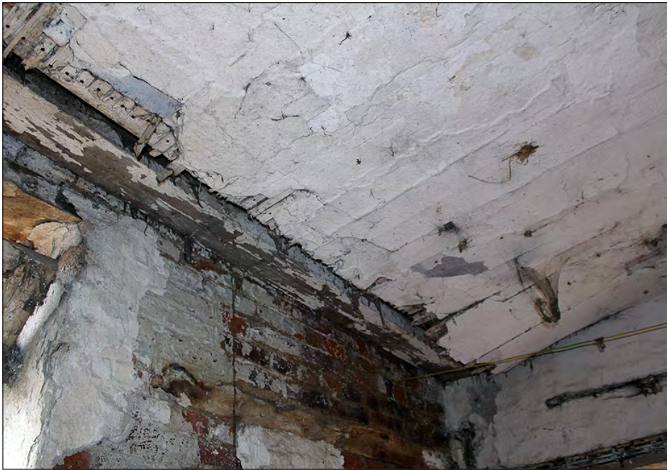
Plate 95. Building 5, interior. Ground floor west side room, ceiling. View looking southwest
