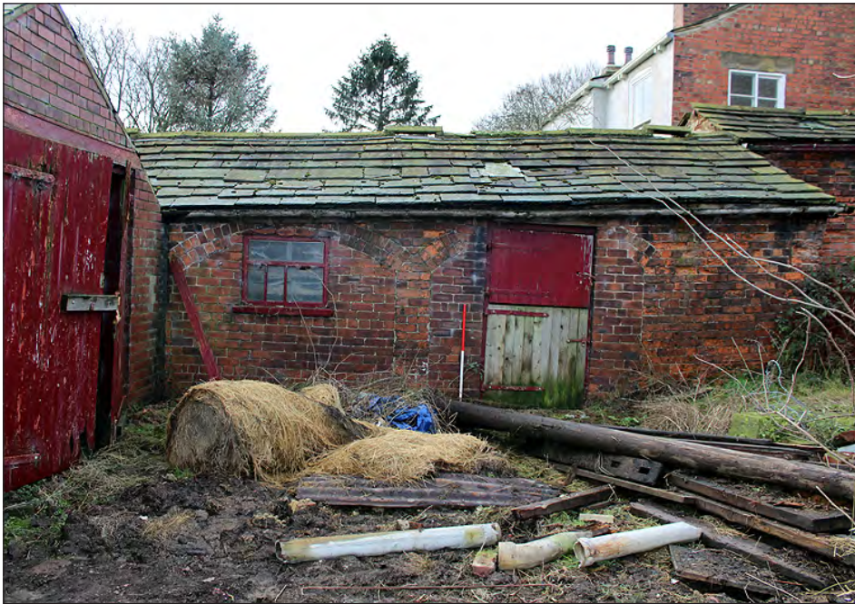
Plate 206. Building 10. East elevation. View looking west-southwest
