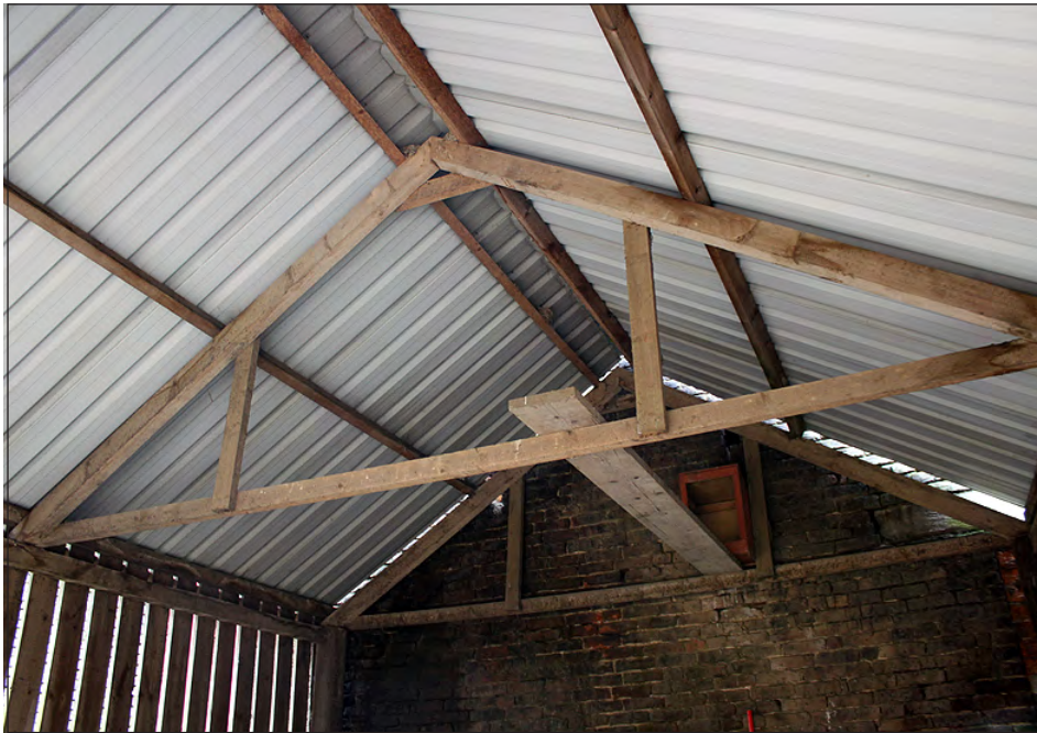
Plate 128. Timber garage extension, interior. Roof structure. View looking southeast
