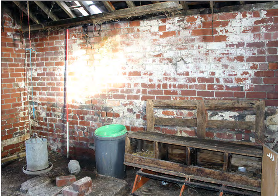
Plate 199. Building 9, interior. East elevation. View looking northeast
