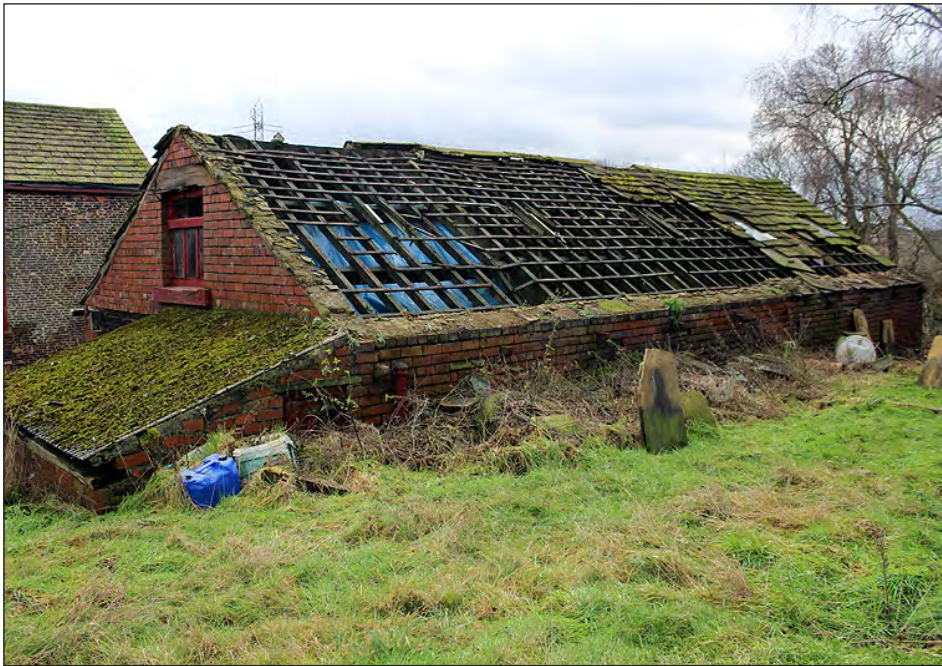
Plate 12. Building 2. North and east elevations. View looking southwest
