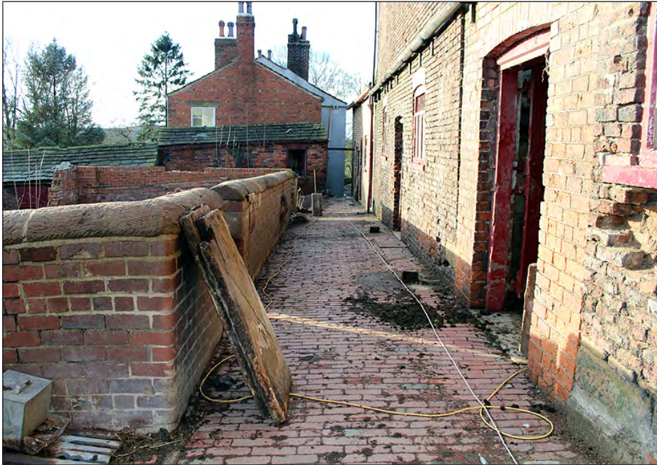
Plate 241. Causeway along south side of Buildings 4, 5 and 6. View looking west-southwest
