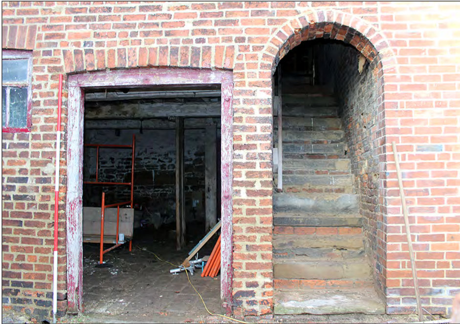
Plate 41. Building 4. South elevation doorways. View looking north-northwest
