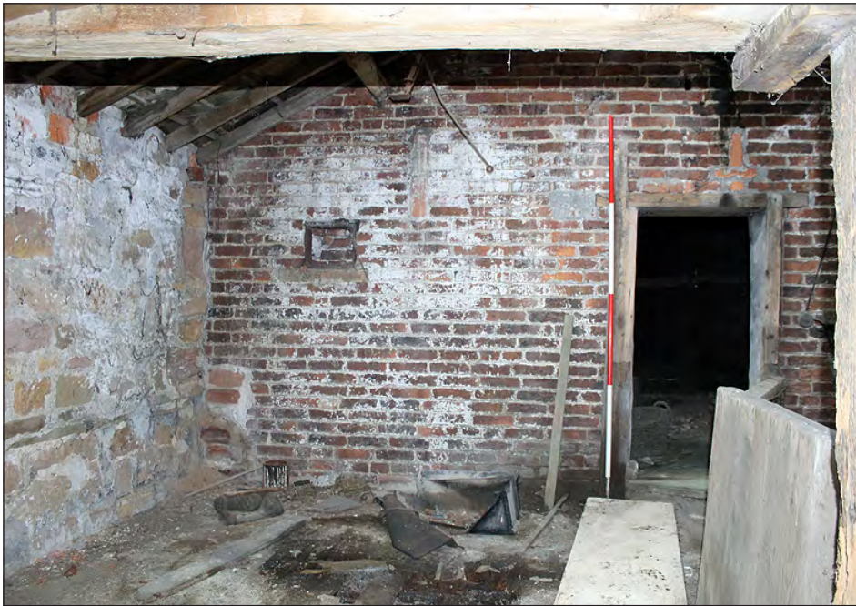
Plate 140. Building 6, interior. West elevation at mezzanine level. View looking west-southwest
