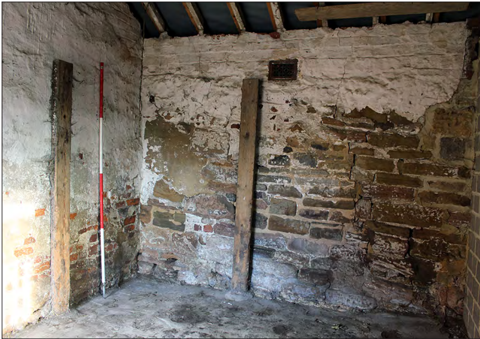
Plate 162. Building 7, interior. South side room. View looking northeast
