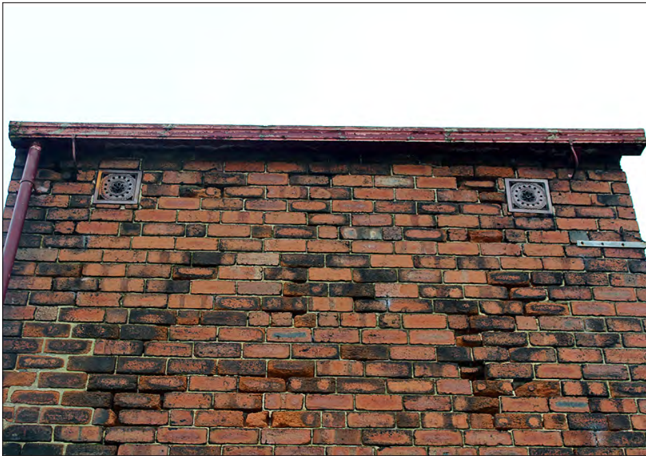
Plate 170. Building 8. South elevation, showing ceramic air brick vents. View looking north-northwest
