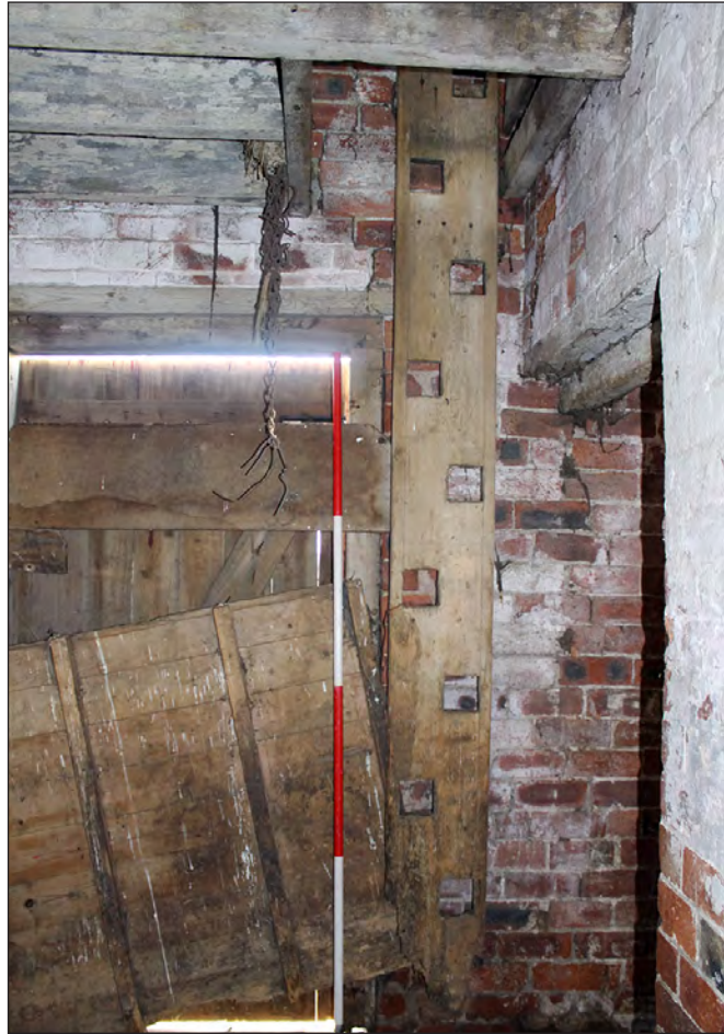
Plate 185. Building 8, interior. South elevation of the ground floor east side room, showing Jacob's ladder. View looking south-southeast
