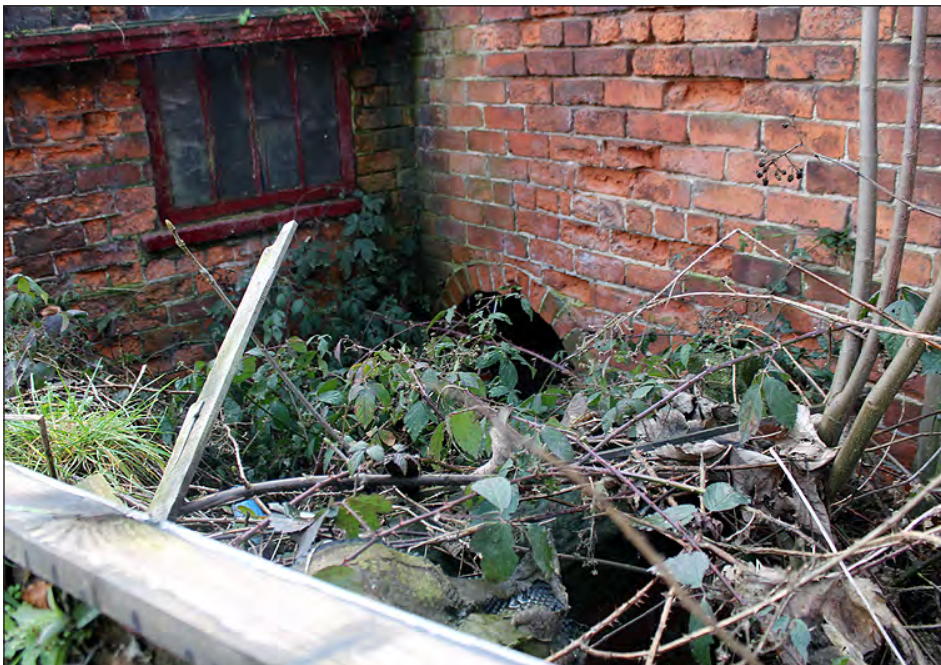
Plate 224. Building 11. View to ground floor pigsty. View looking south
