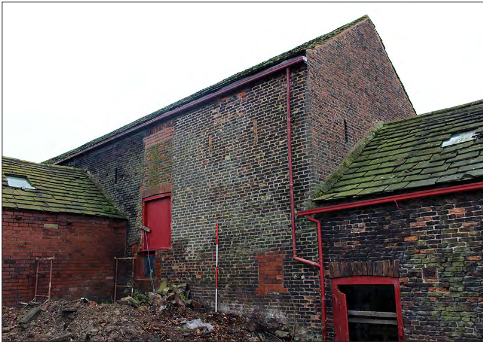
Plate 70. Building 5. West end of the north elevation. View looking southeast
