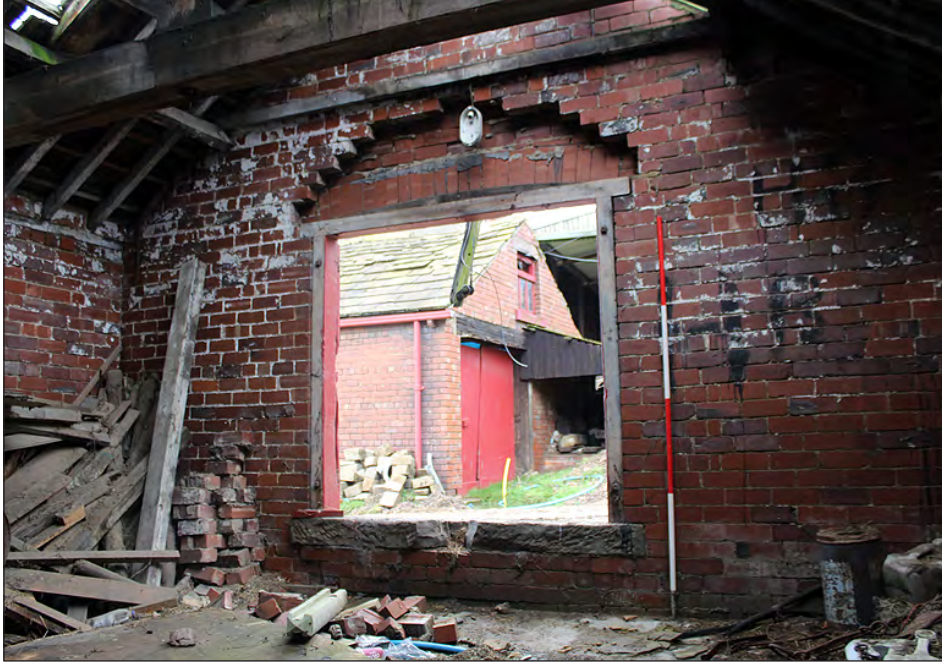
Plate 121. Brick garage extension, interior. North elevation. View looking northwest
