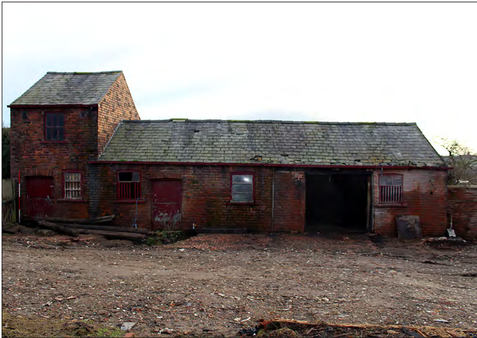
Plate 164. Building 8. North elevation. View looking south-southeast
