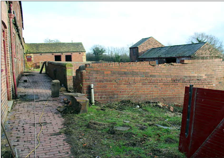
Plate 240. Causeway along south side of Buildings 4, 5 and 6. View looking east-northeast
