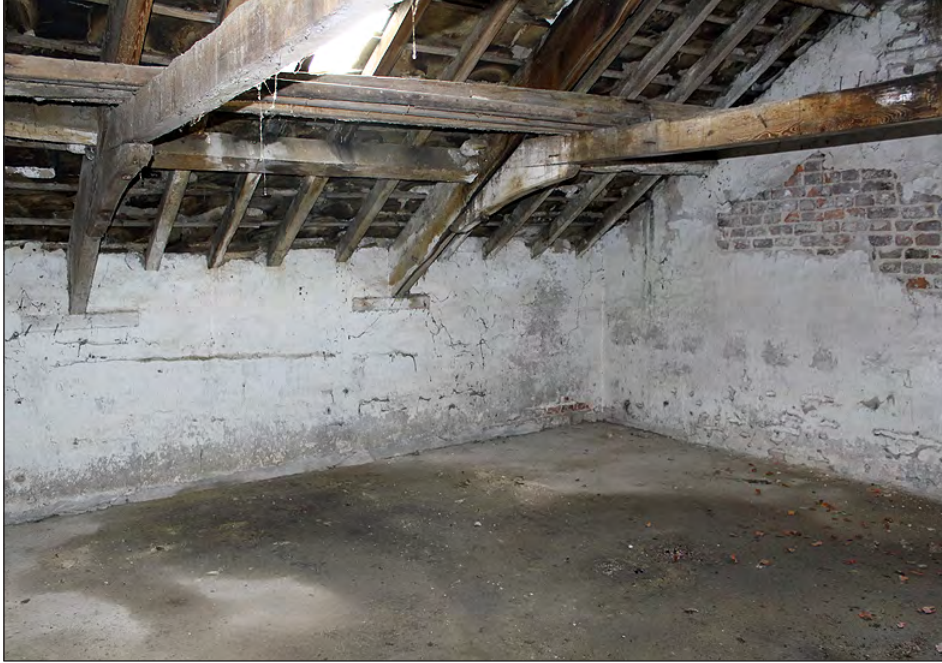
Plate 59. Building 4, interior. First floor. View looking southwest
