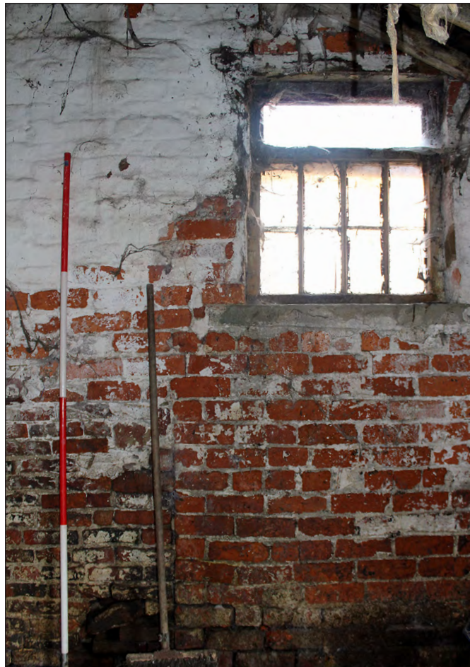
Plate 214. Building 10, interior. North elevation. View looking north-northwest
