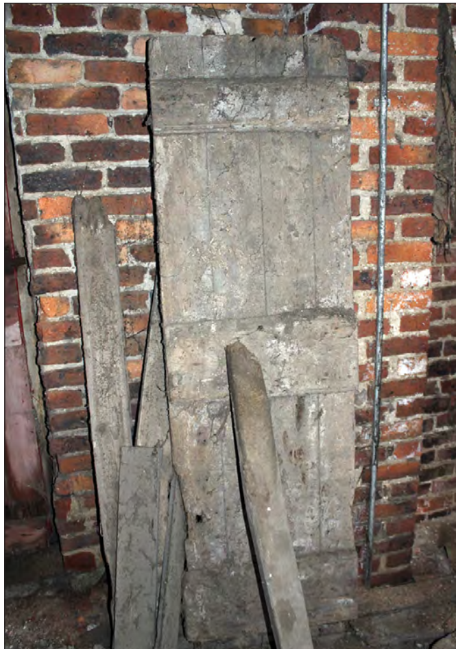
Plate 116. Building 5. Plank and batten door. View looking southeast
