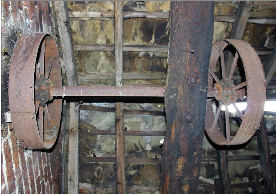
Plate 147. Building 6, interior. In situ line shaft and wheels. View looking north-northwest
