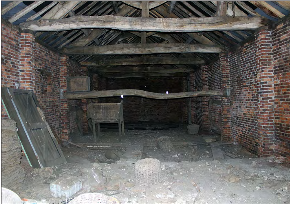
Plate 105. Building 5, interior. First floor. View looking west-southwest
