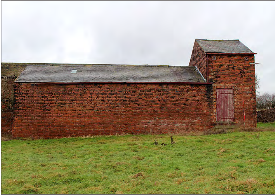
Plate 167. Building 8. South elevation. View looking north-northwest
