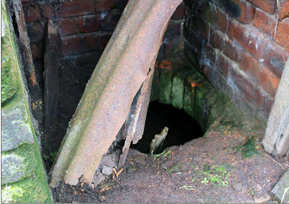
Plate 253. View within well structure. View looking northwest
