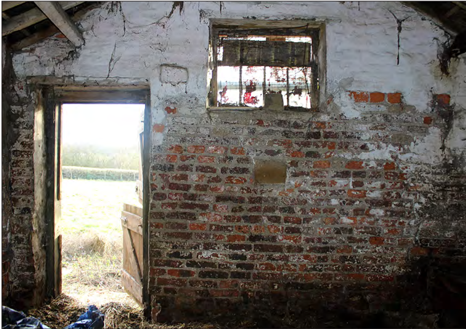
Plate 217. Building 10, interior. South elevation. View looking south-southeast
