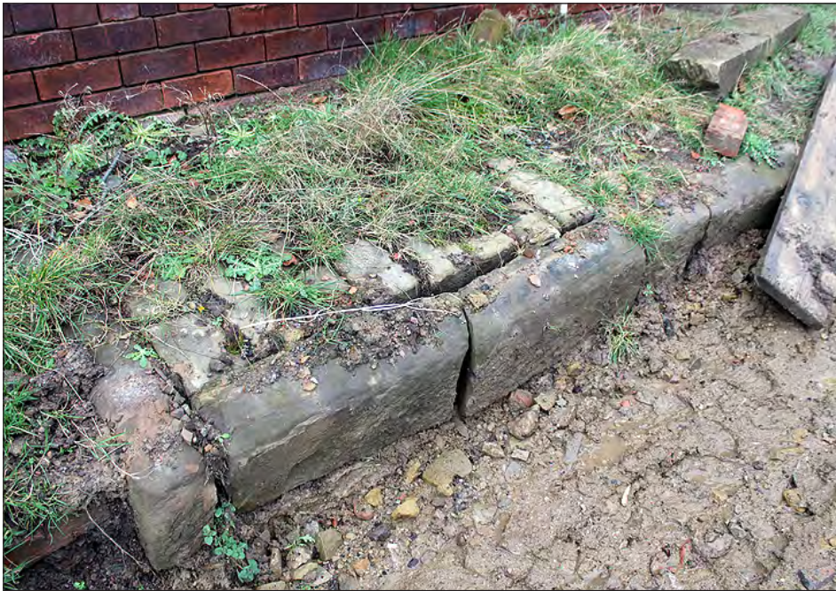
Plate 36. Raised causeway along the south side of Building 2. View looking northeast
