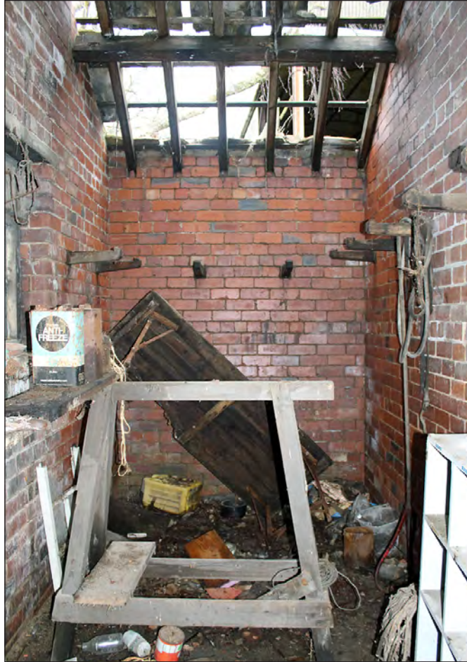
Plate 19. Building 2, interior. West side tack room. View looking north-northwest
