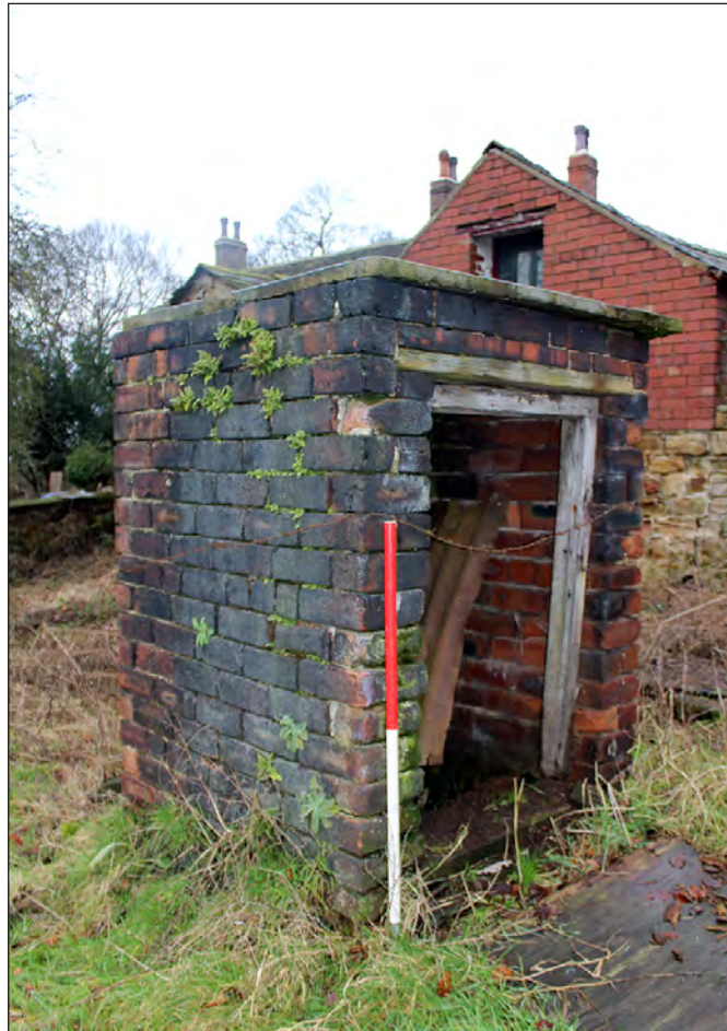
Plate 252. Well structure. View looking northwest
