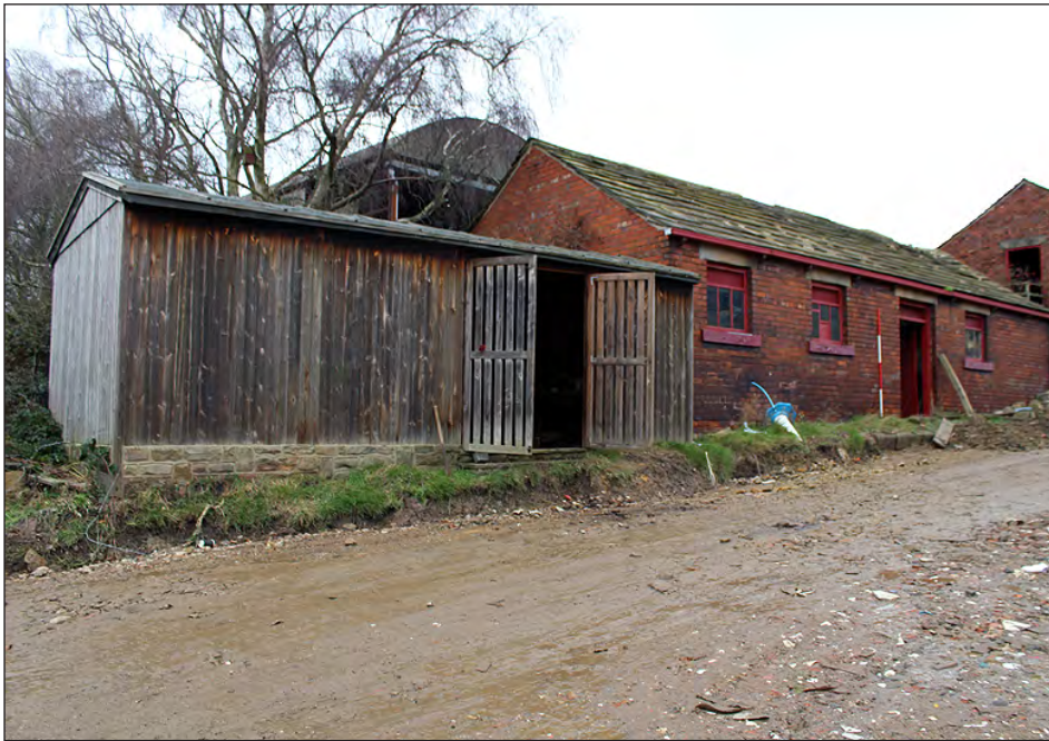
Plate 10. Building 1. View looking northeast
