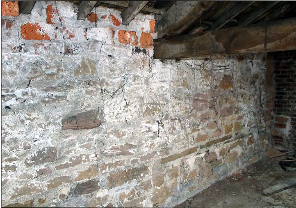
Plate 137. Building 6, interior. South elevation at mezzanine level. View looking southwest
