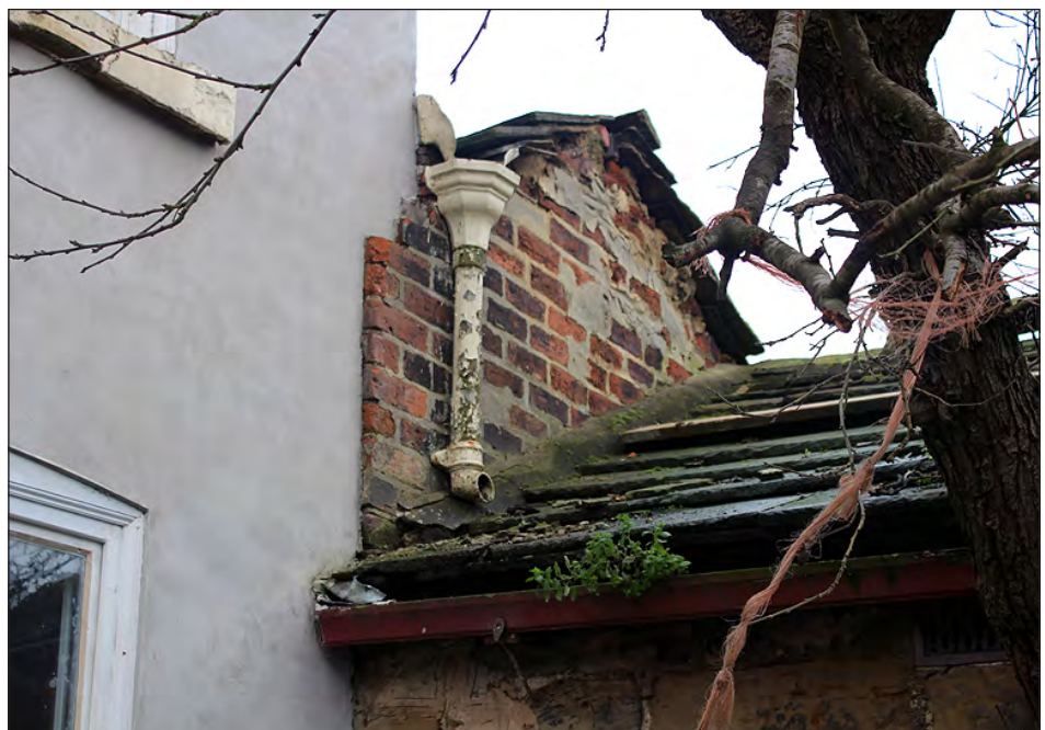
Plate 228. Building 11. South elevation. View looking north
