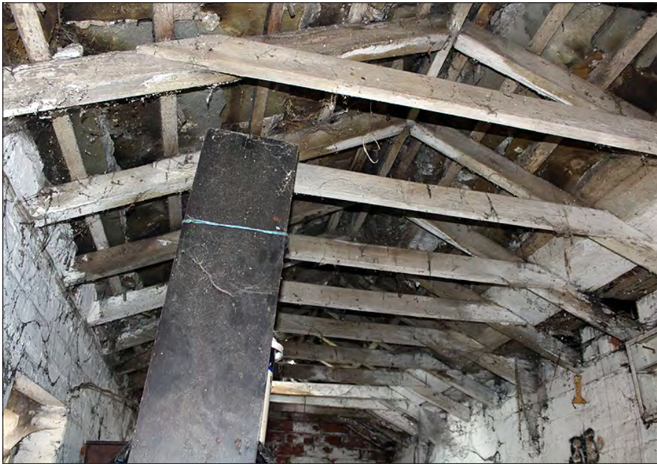
Plate 232. Building 11, interior. First floor roof structure. View looking south-southeast
