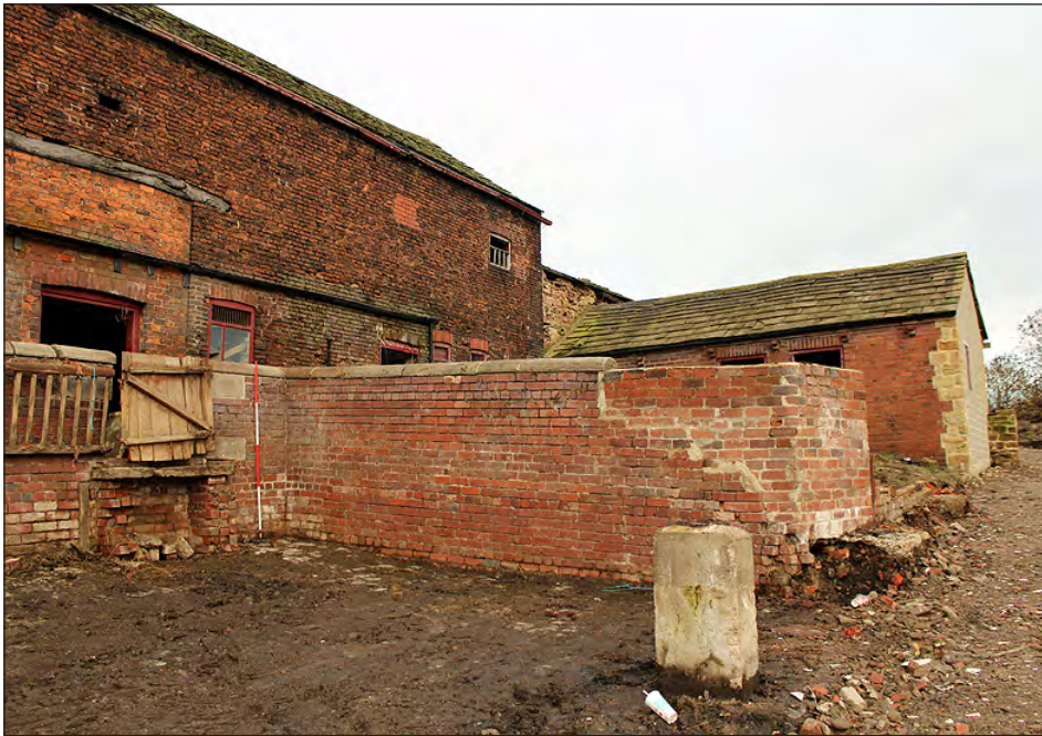
Plate 244. East wall of former shed within yard. View looking northeast
