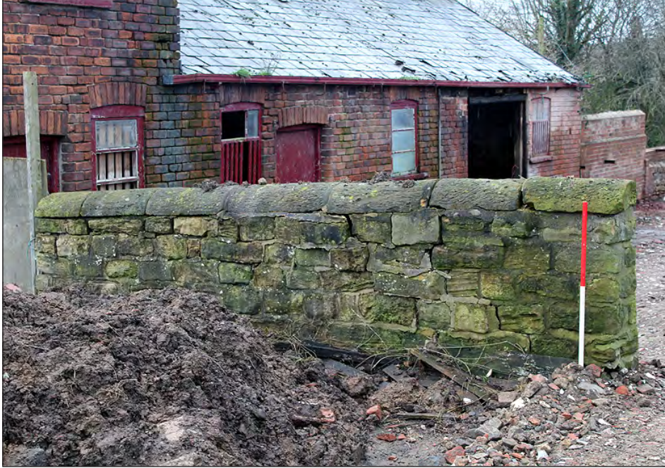
Plate 249. East wall of yard. View looking southwest
