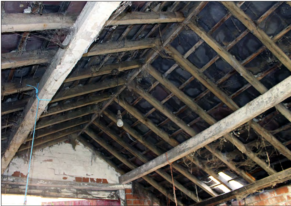
Plate 204. Building 9, interior. Roof structure. View looking northeast
