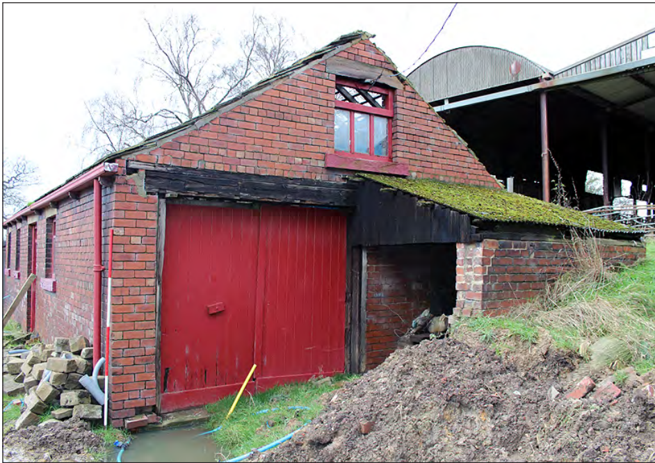
Plate 14. Building 2. East elevation. View looking northwest
