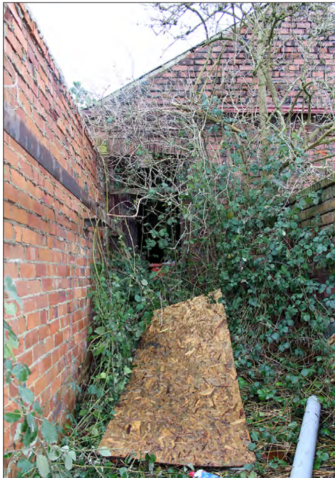
Plate 194. Building 8. West side extension. View looking east-northeast
