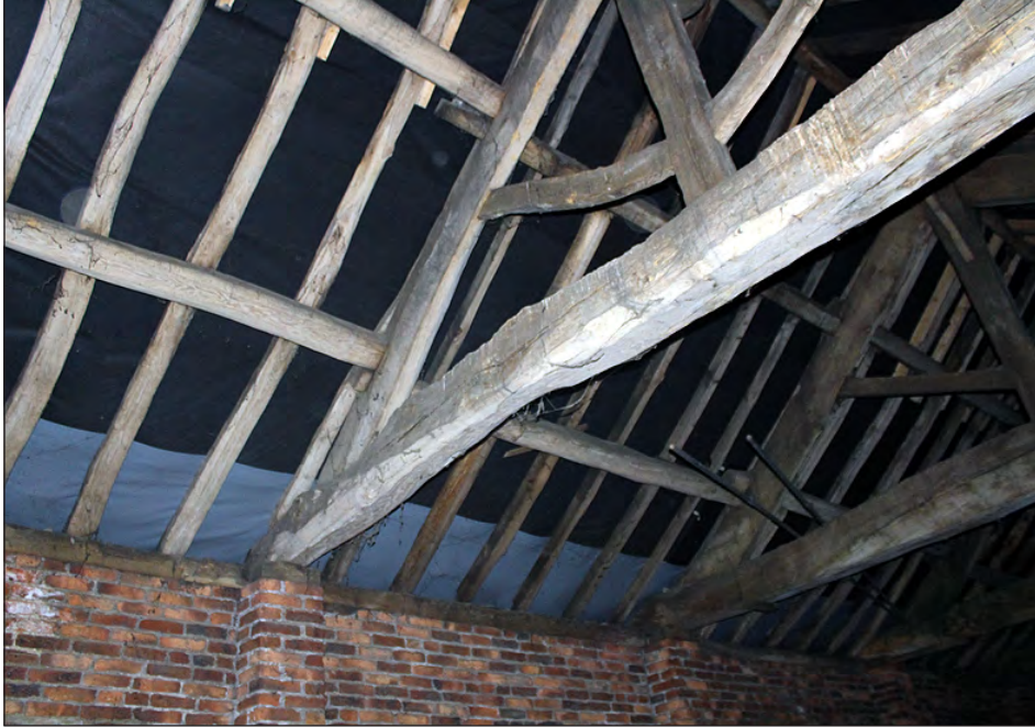
Plate 113. Building 5, interior. Roof truss. View looking southwest
