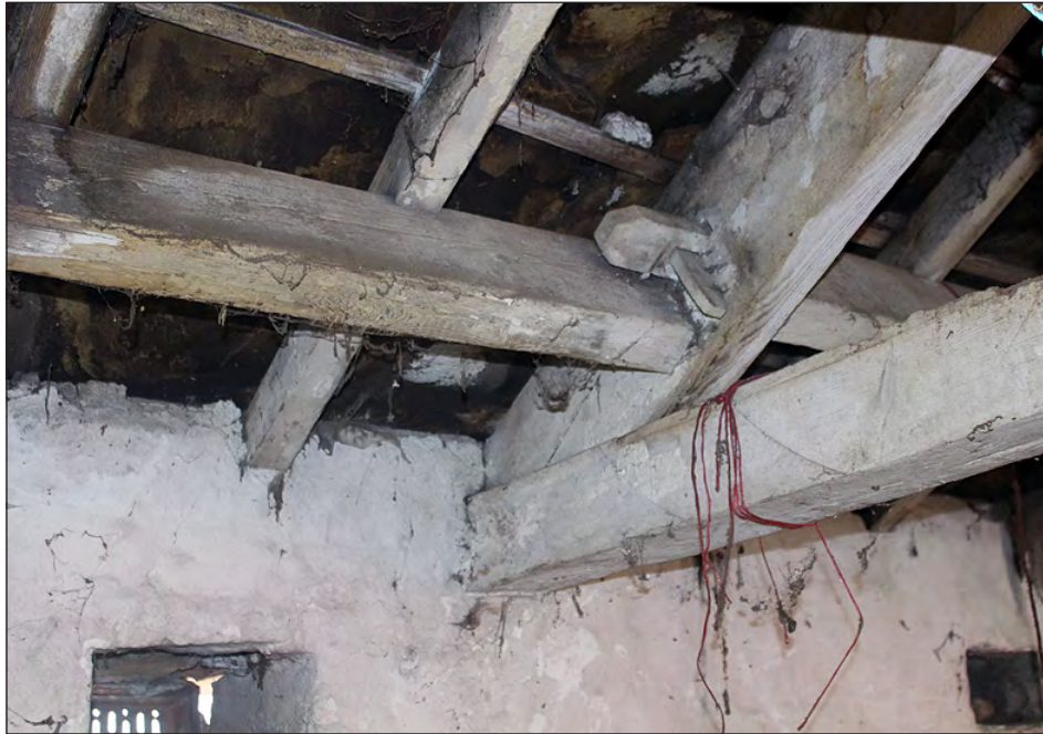
Plate 221. Building 10, interior. Roof structure. View looking northwest
