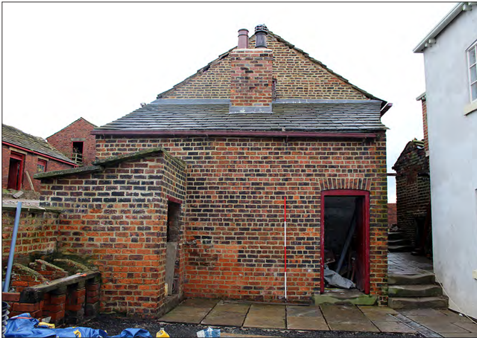
Plate 42. Building 4. West elevation. View looking east-northeast
