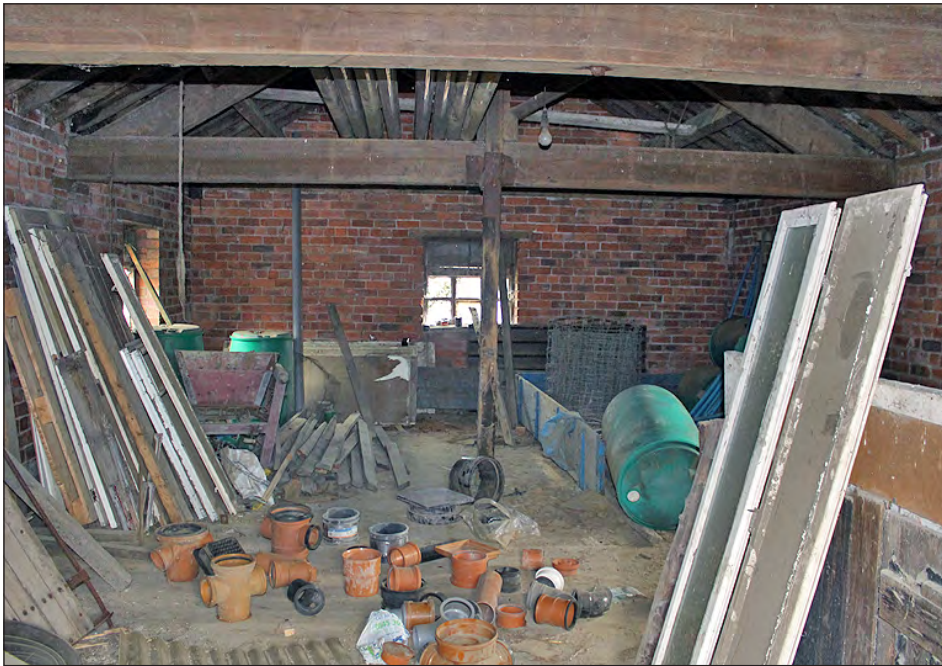
Plate 28. Building 3, interior. East side of the first floor. View looking east-northeast
