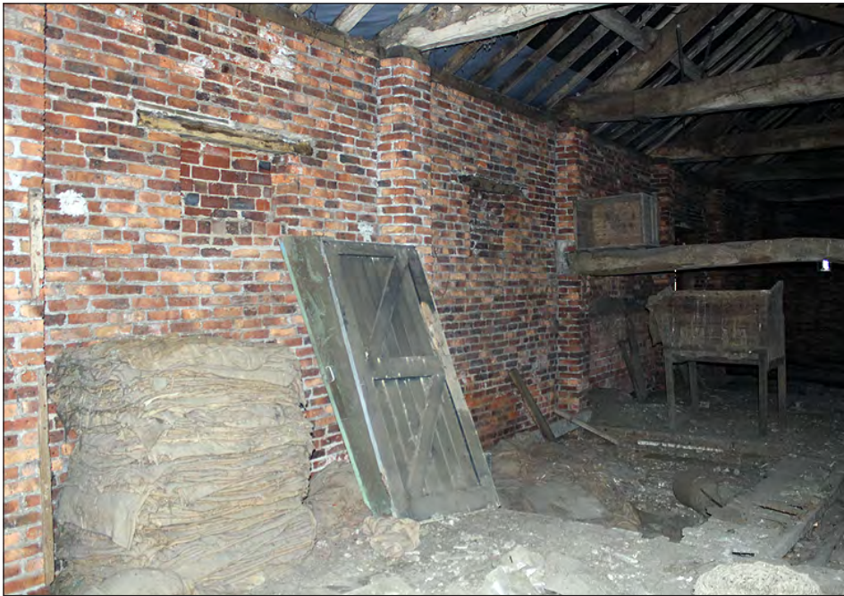
Plate 110. Building 5, interior. First floor, south elevation. View looking southwest
