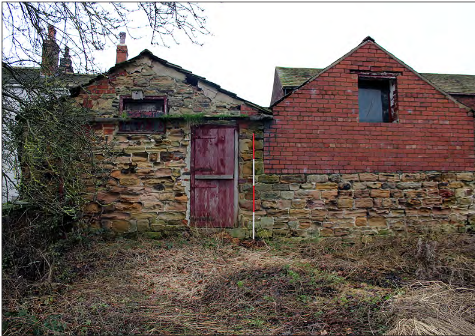
Plate 198. Buildings 9 and 10. South elevation. View looking north-northwest
