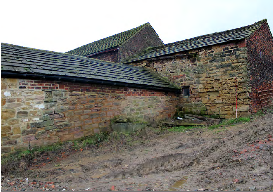
Plate 131. Building 6. South elevation. Building 7. East elevation. View looking northwest
