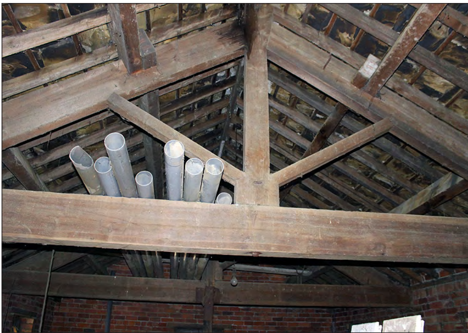
Plate 34. Building 3, interior. Roof structure. View looking east-northeast
