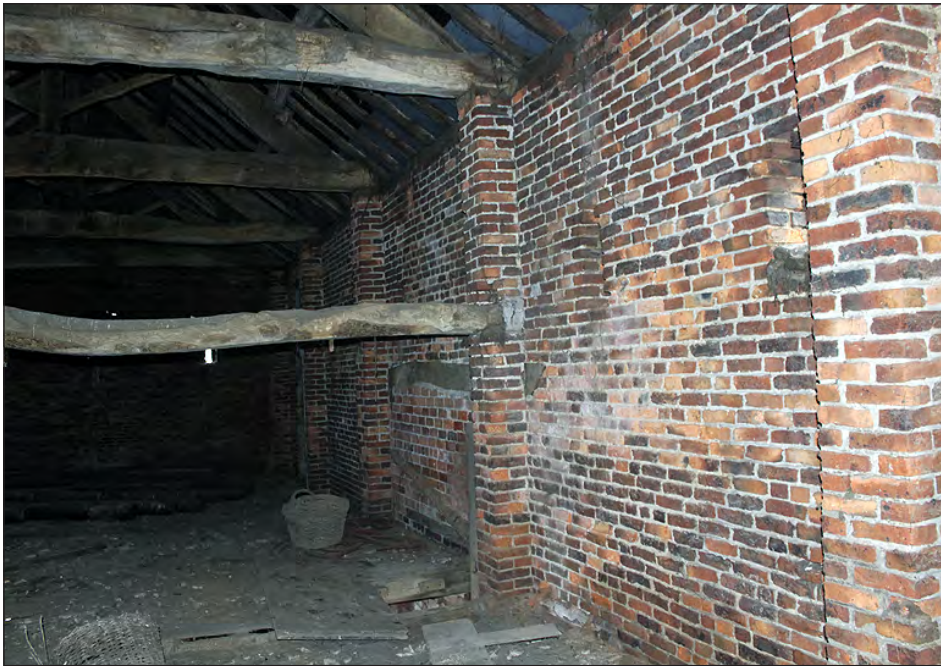
Plate 106. Building 5, interior. First floor, north elevation. View looking west
