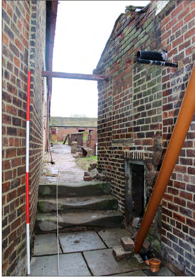
Plate 43. Passageway along the south side of Building 4. View looking east
