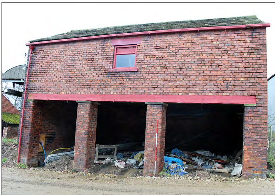
Plate 22. Building 3. South elevation. View looking north-northwest
