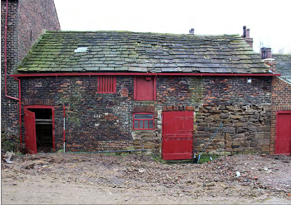
Plate 37. Building 4. North elevation. View looking south-southeast
