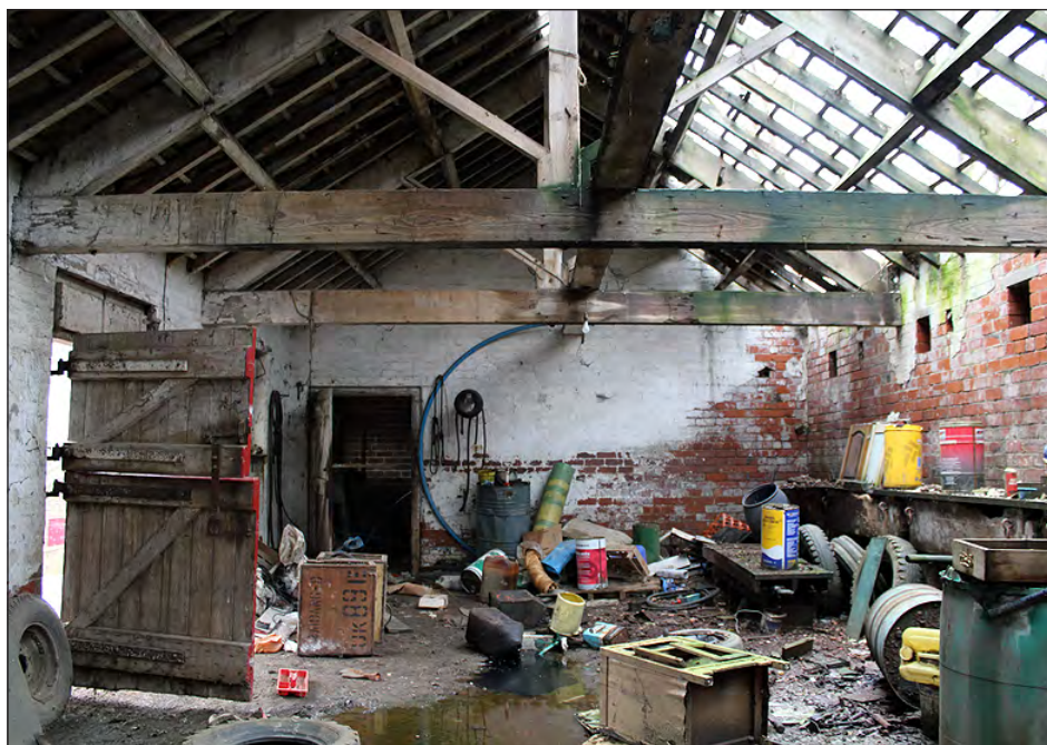
Plate 16. Building 2, interior. Stabling area. View looking west-southwest
