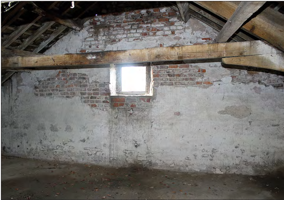
Plate 60. Building 4, interior. West elevation of the first floor. View looking west-southwest
