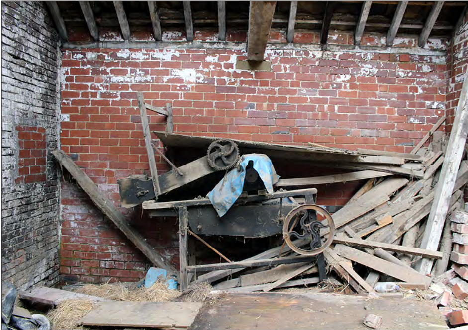
Plate 123. Brick garage extension, interior. West elevation. View looking west-southwest
