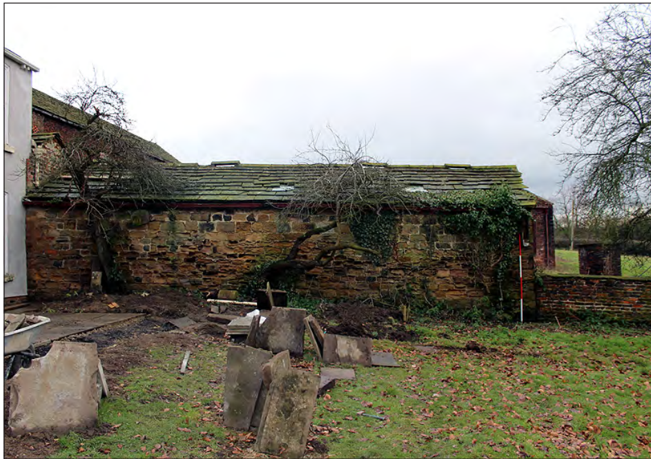
Plate 208. Building 10. West elevation. View looking east-northeast
