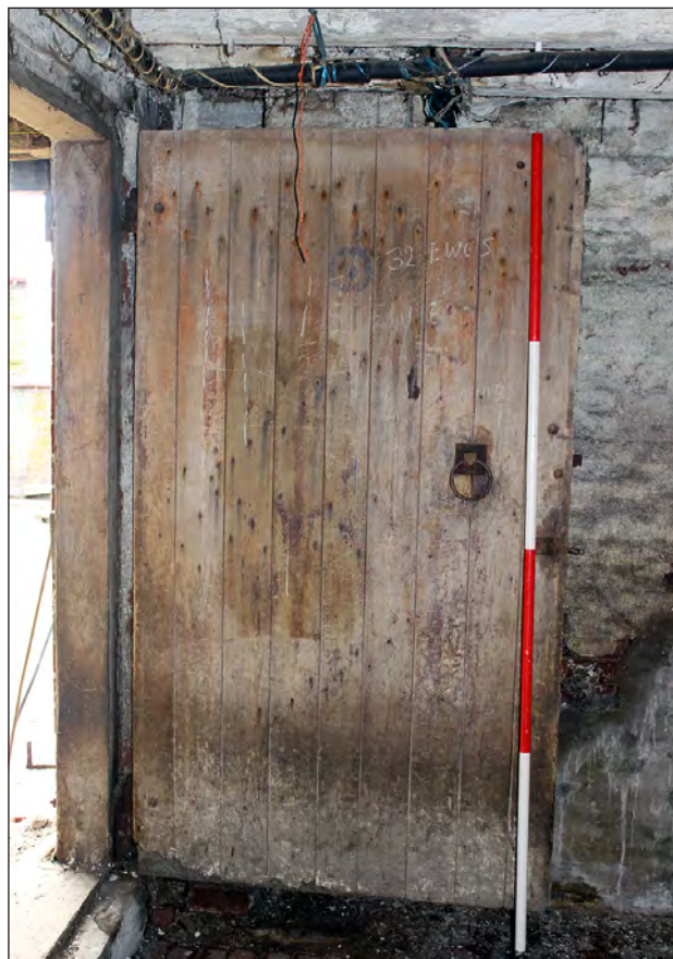
Plate 100. Building 5, interior. Ground floor cross-passage, south side door. View looking south-southeast
