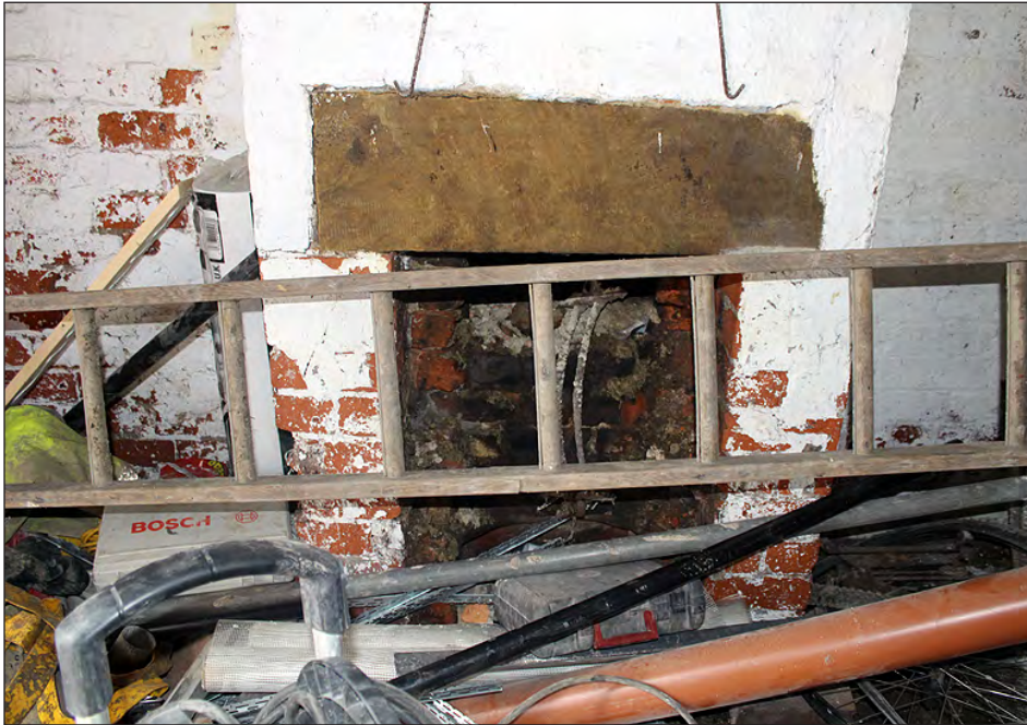
Plate 65. Building 4, interior. West side extension fireplace. View looking north-northwest
