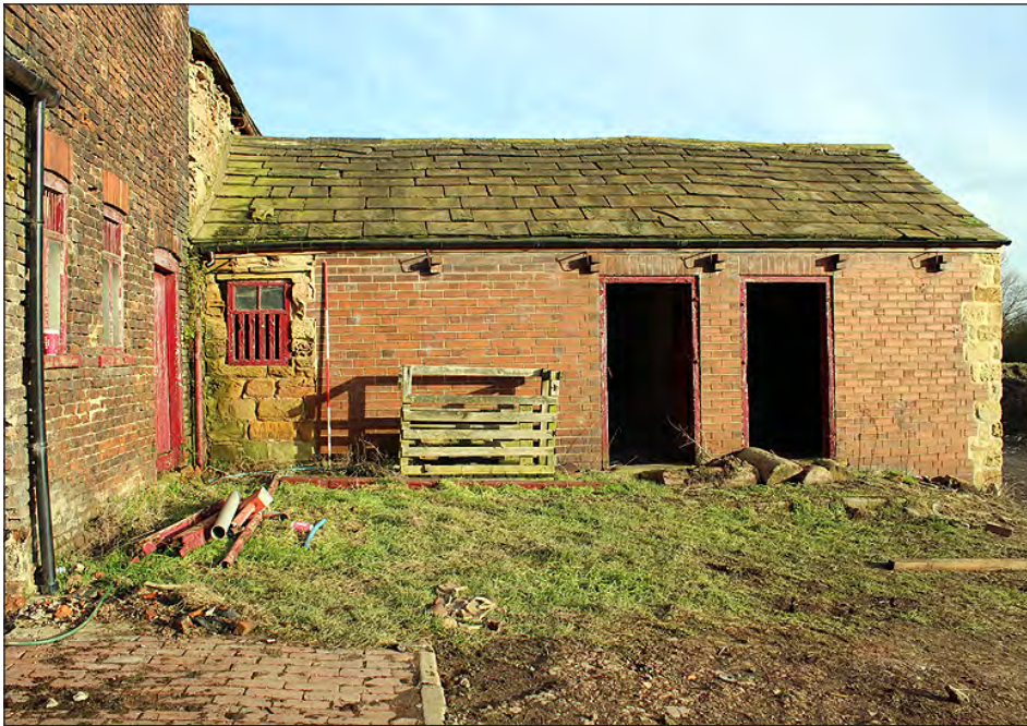
Plate 152. Building 7. West elevation. View looking east-northeast
