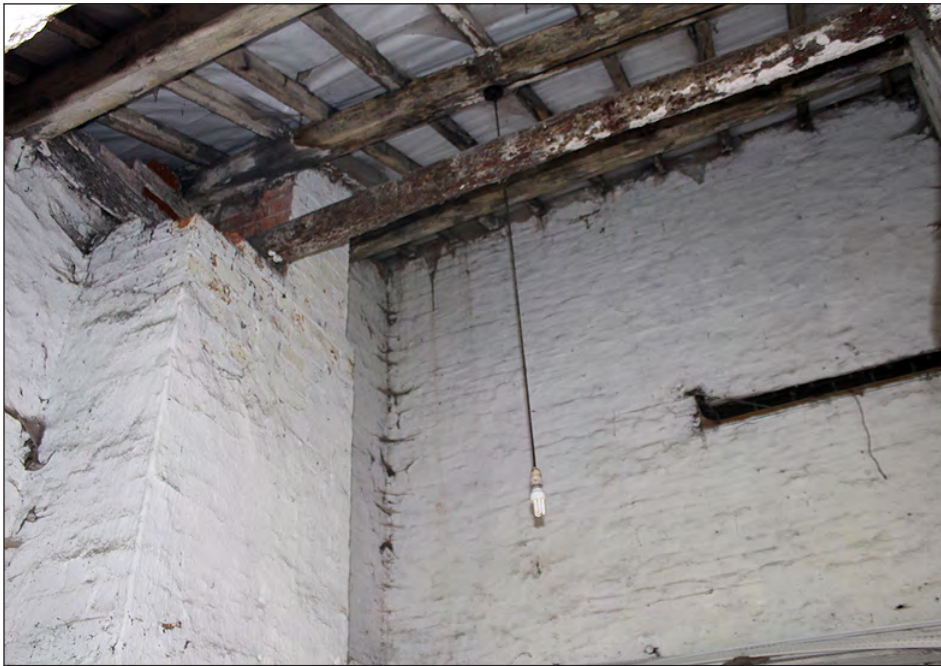
Plate 66. Building 4, interior. West side extension roof structure. View looking northeast
