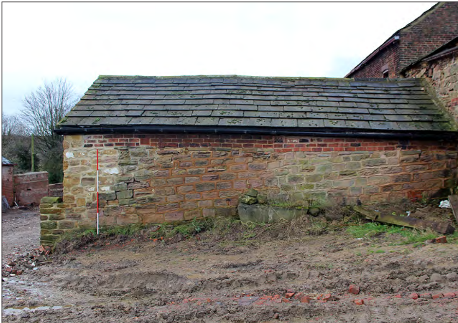
Plate 150. Building 7. East elevation. View looking west-southwest
