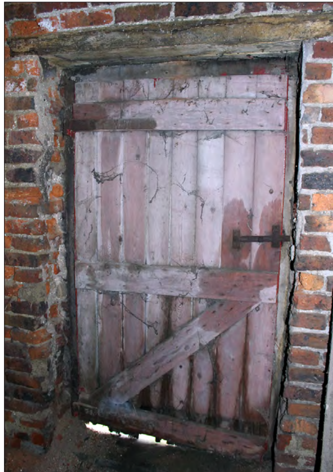
Plate 108. Building 5, interior. First floor, north elevation taking-in door. View looking north-northwest
