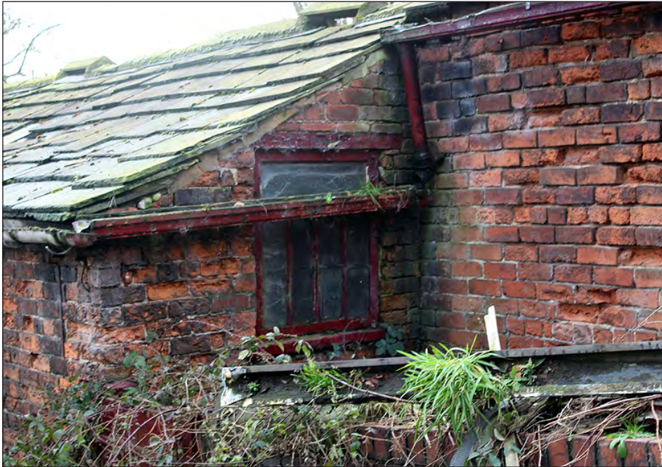
Plate 205. Building 10. North elevation. View looking southwest
