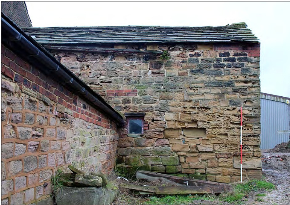
Plate 132. Building 6. East side of the south elevation. View looking north-northwest
