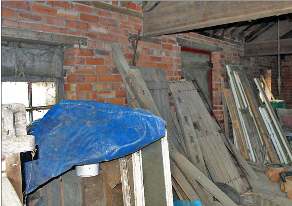
Plate 29. Building 3, interior. North elevation of the first floor. View looking northeast
