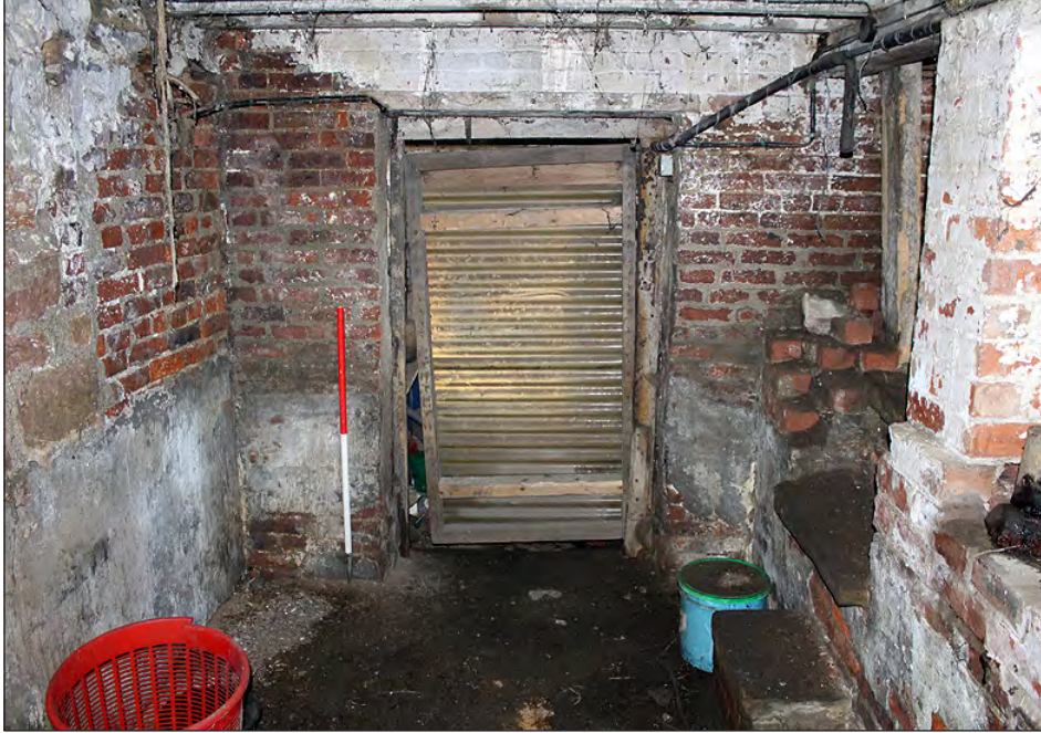
Plate 139. Building 6, interior. West elevation at passageway level. View looking west-southwest
