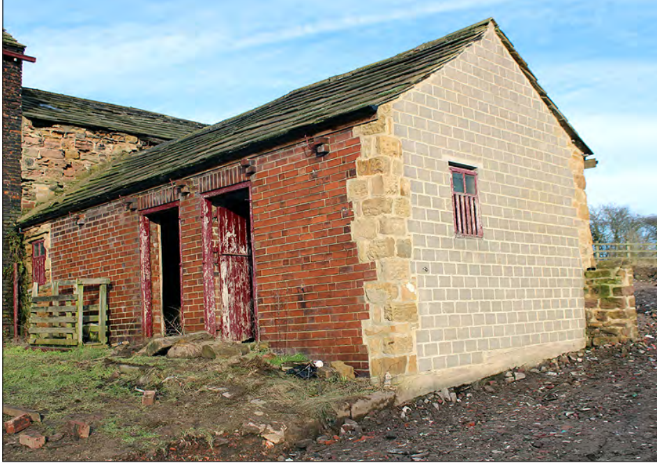
Plate 151. Building 7. South and west elevation. View looking northeast
