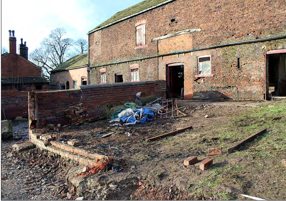
Plate 245. Area east of former shed within yard. View looking northwest
