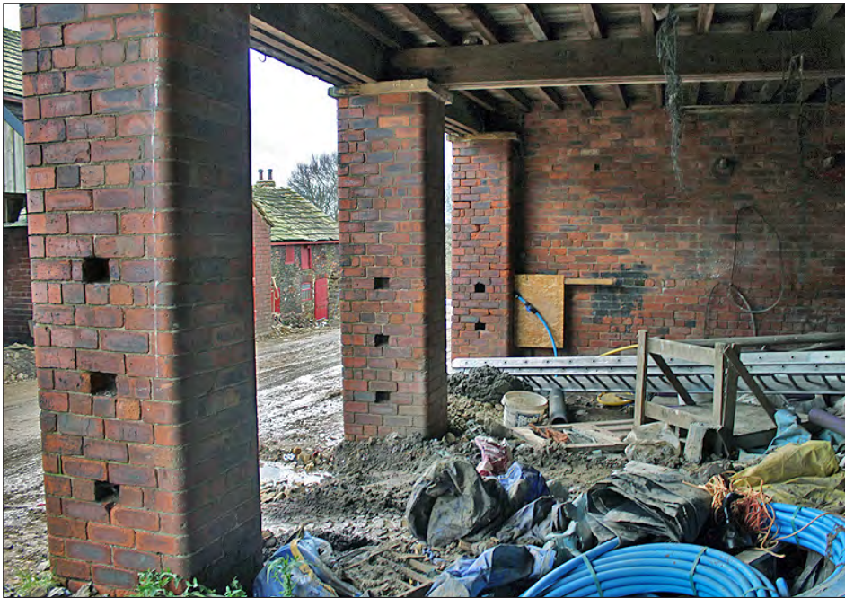
Plate 26. Building 3, interior. South side of the ground floor. View looking west-southwest
