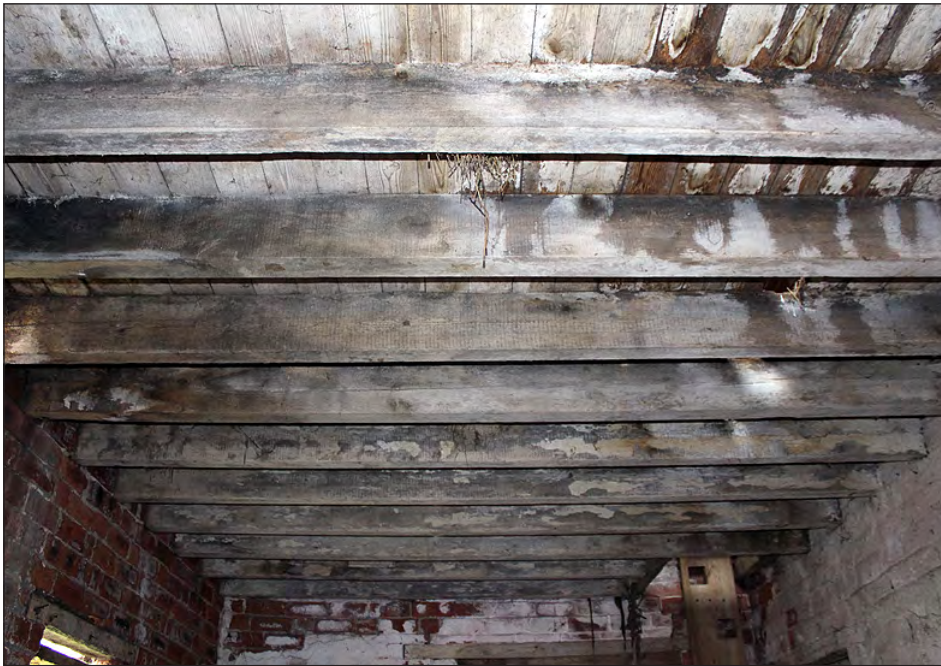
Plate 190. Building 8, interior. Ceiling of the east side room. View looking south-southeast
