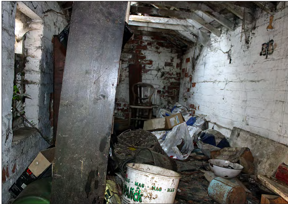
Plate 230. Building 11, interior. First floor. View looking south
