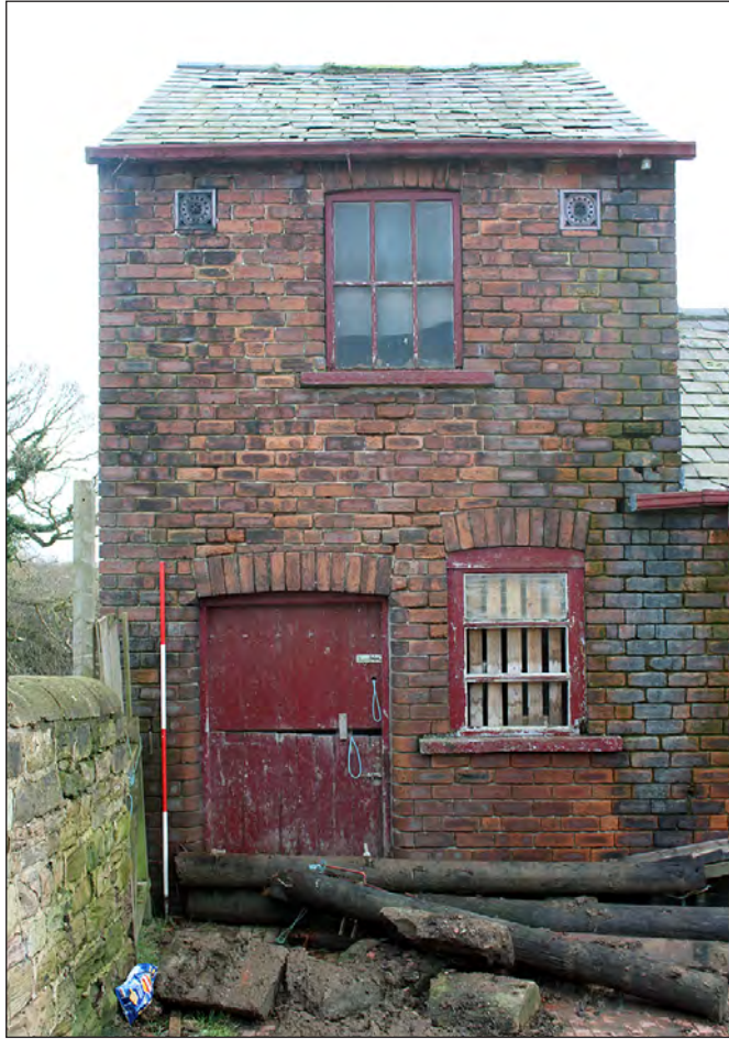
Plate 165. Building 8. East end of the north elevation. View looking south-southeast
