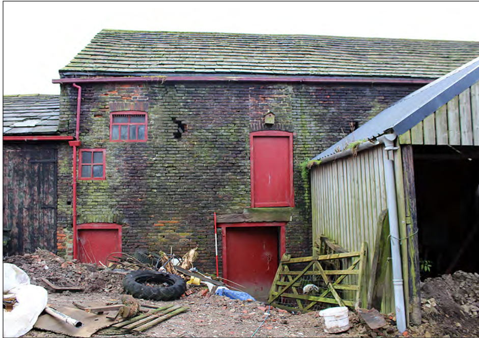
Plate 71. Building 5. East end of the north elevation. View looking south-southeast
