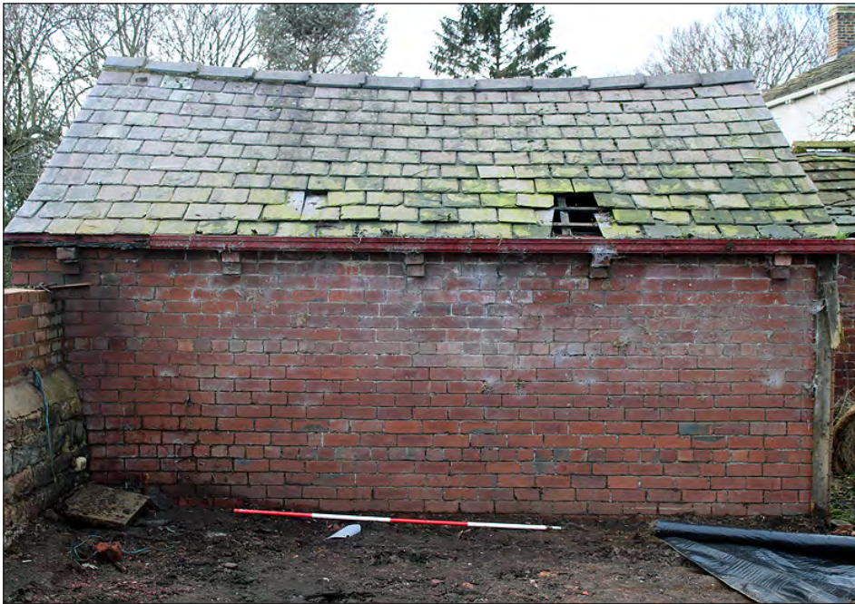
Plate 196. Building 9. East elevation. View looking west-southwest
