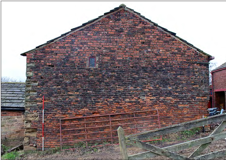
Plate 130. Building 6. East elevation. View looking west-southwest
