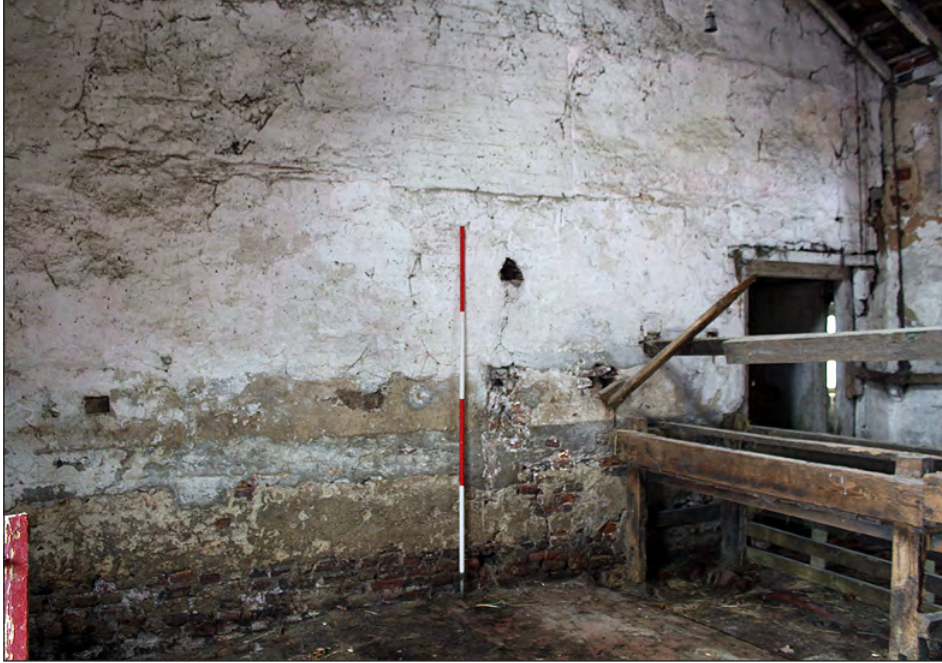
Plate 55. Building 4, interior. West elevation. View looking northwest
