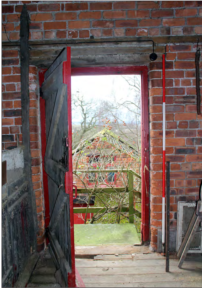
Plate 33. Building 3, interior. West elevation of the first floor. View looking west-southwest
