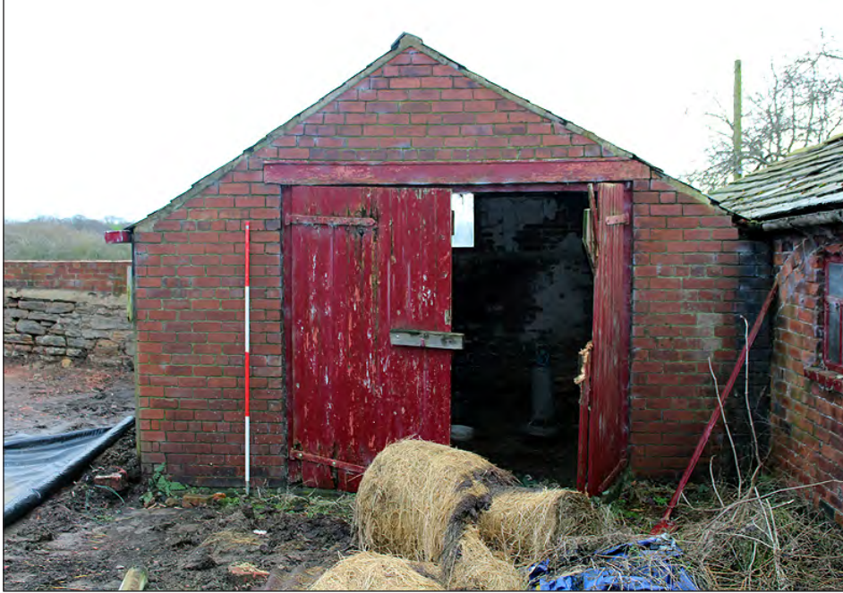
Plate 195. Building 9. North elevation. View looking south-southeast
