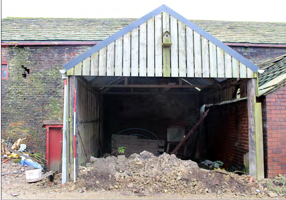
Plate 125. Timber garage extension. North elevation. View looking south-southeast
