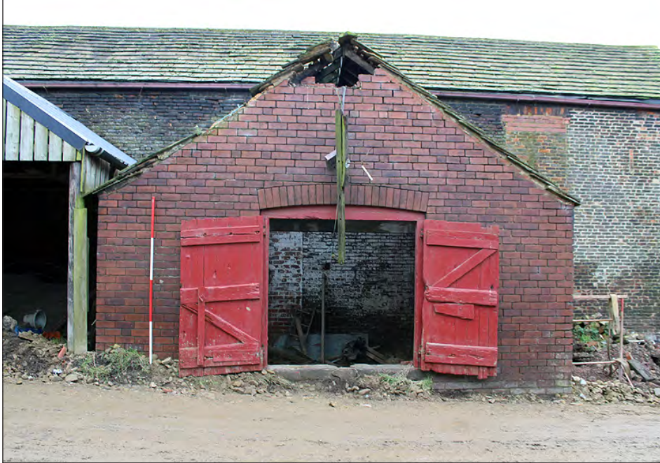
Plate 119. Brick garage extension. North elevation. View looking south-southeast
