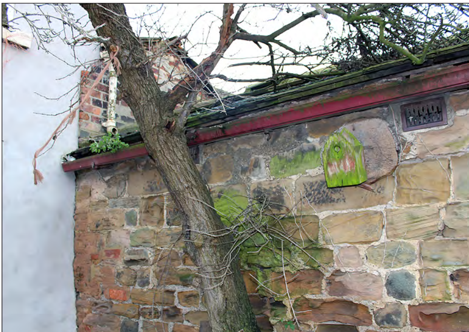
Plate 210. Building 10. North end of west elevation. View looking northeast
