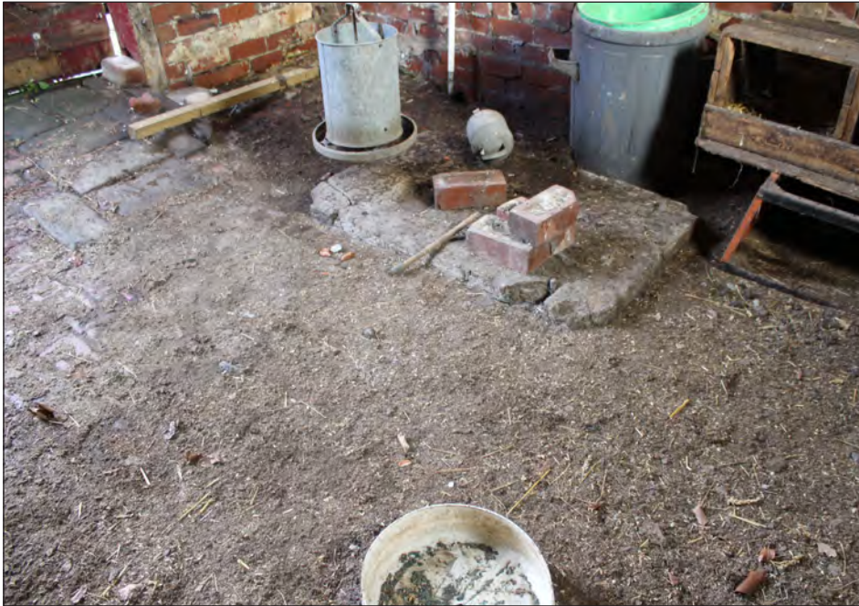
Plate 203. Building 9, interior. Floor surface. View looking northeast
