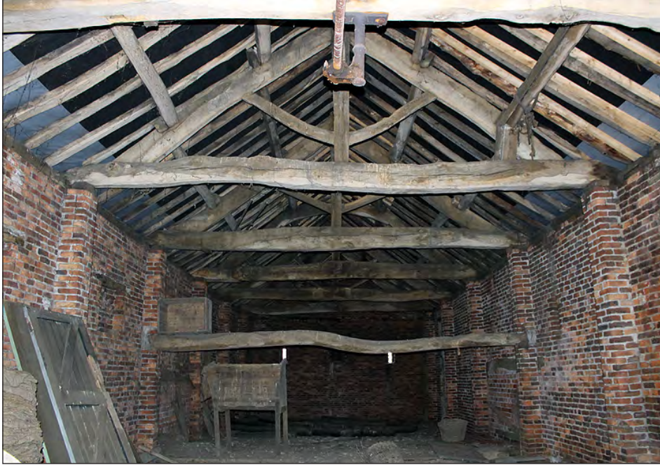
Plate 111. Building 5, interior. Roof structure. View looking west-southwest
