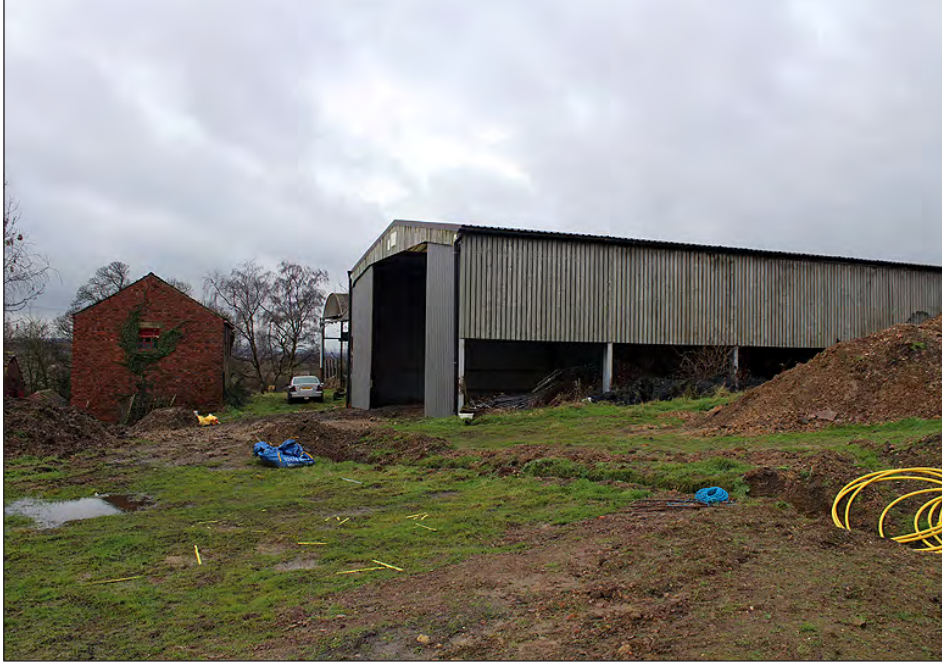
Plate 5. General view of the sheds to the north side of Newsam Green Farm. View looking northwest
