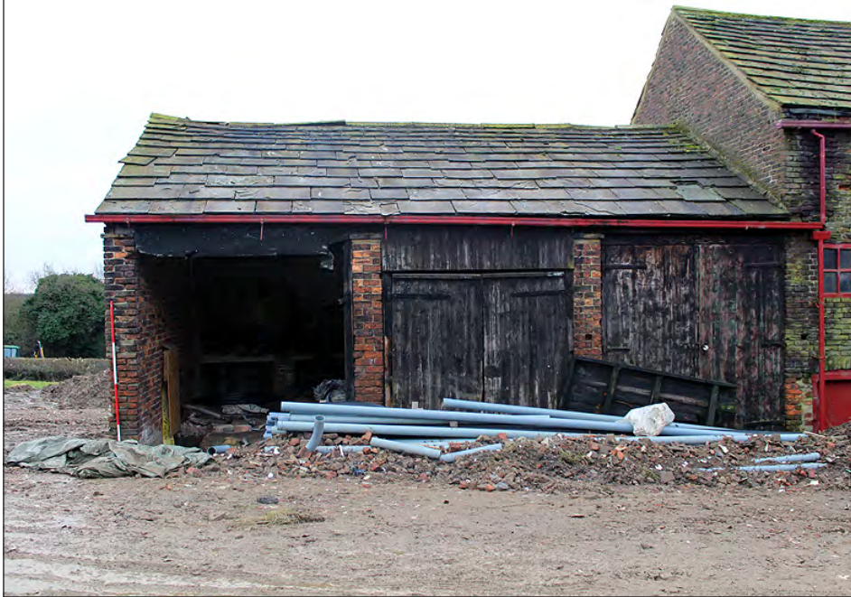
Plate 129. Building 6. North elevation. View looking south-southeast
