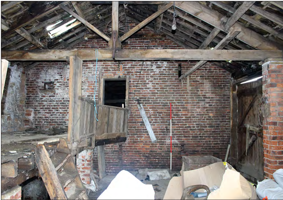
Plate 138. Building 6, interior. West elevation. View looking west-southwest
