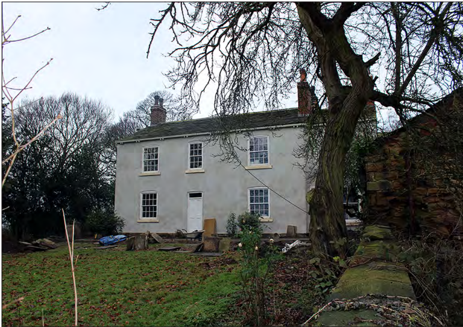
Plate 6. The farmhouse. View looking north-northwest
