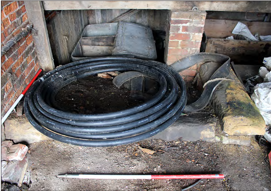
Plate 149. Building 6, interior. Engine base. View looking southeast
