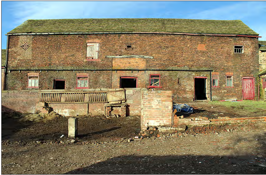
Plate 75. Building 5. South elevation. View looking north-northwest
