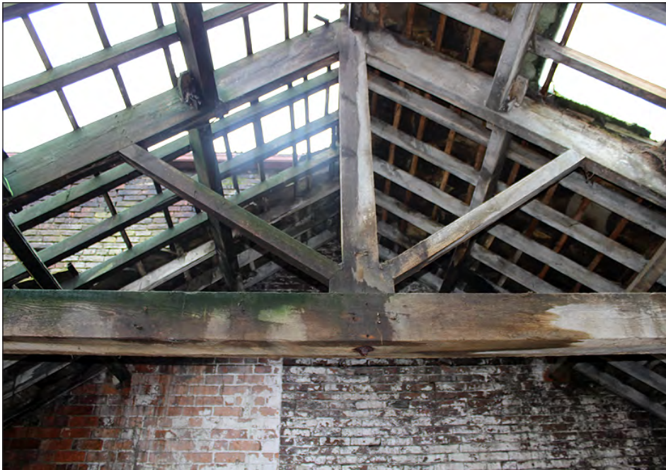
Plate 124. Brick garage extension, interior. Roof truss. View looking south-southeast
