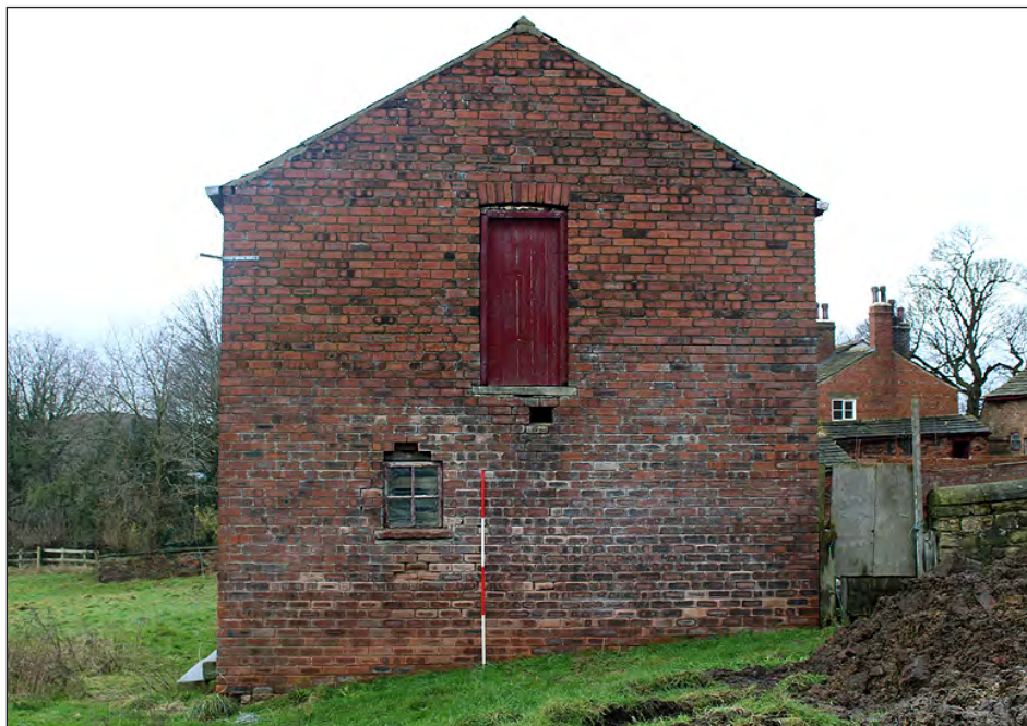
Plate 166. Building 8. East elevation. View looking west-southwest
