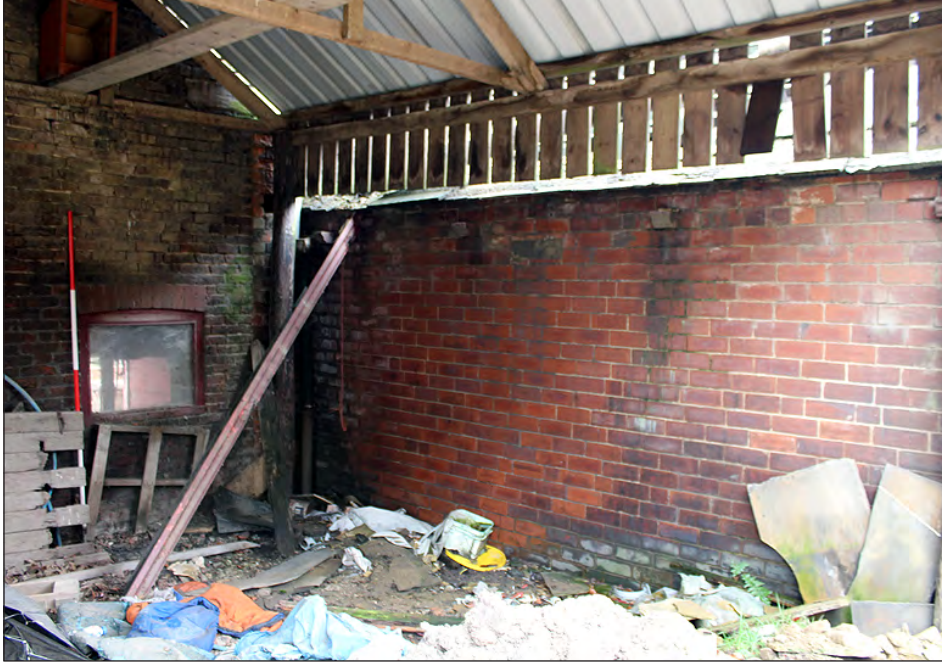
Plate 127. Timber garage extension, interior. West elevation. View looking southwest
