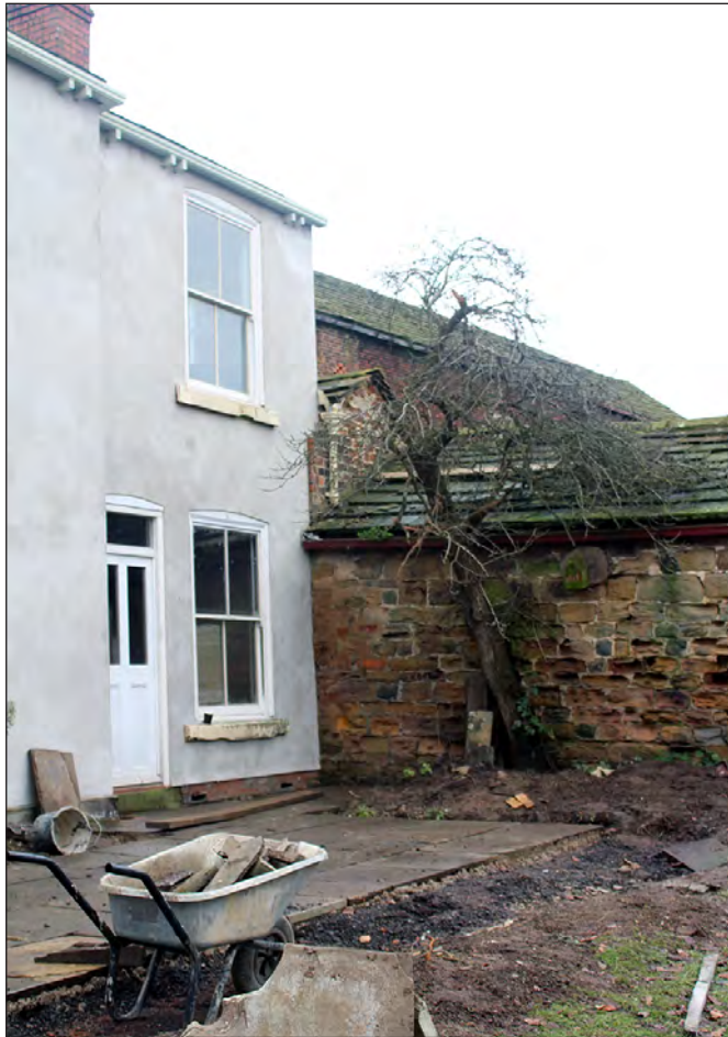
Plate 209. Building 10. North end of west elevation. View looking northeast
