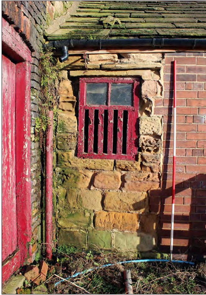
Plate 153. Building 7. North end of west elevation. View looking east-northeast
