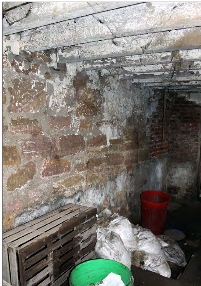
Plate 136. Building 6, interior. South elevation at passageway level. View looking southwest
