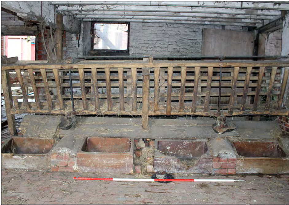
Plate 83. Building 5, interior. Ground floor west side room, feeding troughs and mangers. View looking east-northeast
