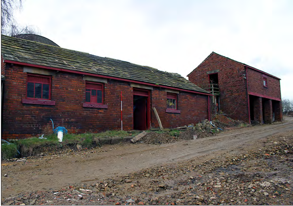
Plate 13. Building 2. South elevation. View looking northeast
