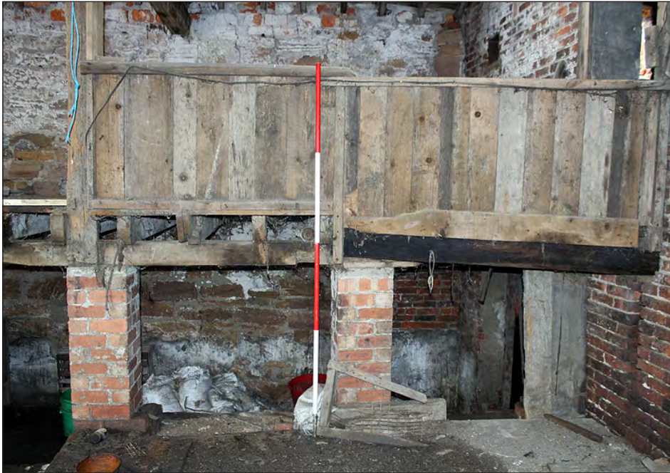
Plate 143. Building 6, interior. Mezzanine. View looking south-southeast
