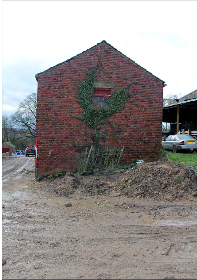
Plate 21. Building 3. East elevation. View looking west-southwest
