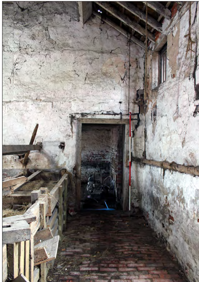
Plate 50. Building 4, interior. View along the north wall of the east side room. View looking west-southwest
