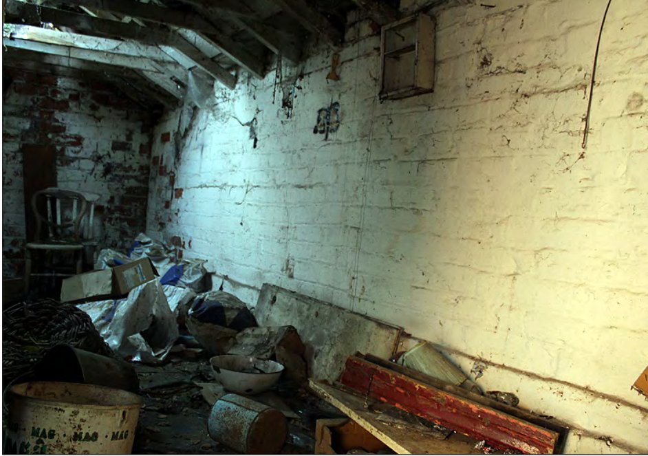
Plate 231. Building 11, interior. First floor. View looking south
