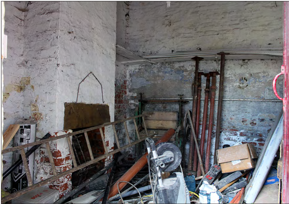
Plate 64. Building 4, interior. West side extension. View looking northeast
