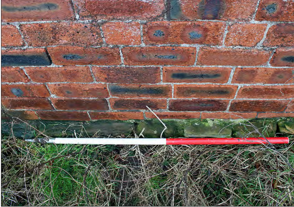
Plate 169. Building 8. South elevation, showing stone plinth. View looking north-northwest
