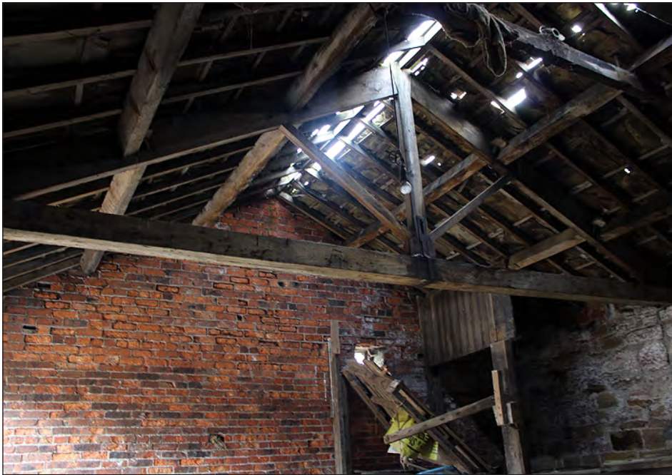
Plate 144. Building 6, interior. Roof structure. View looking southeast
