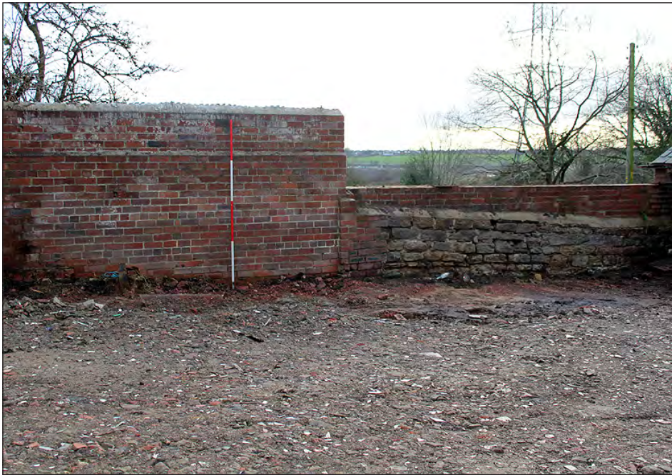
Plate 250. South wall of yard. View looking south-southeast
