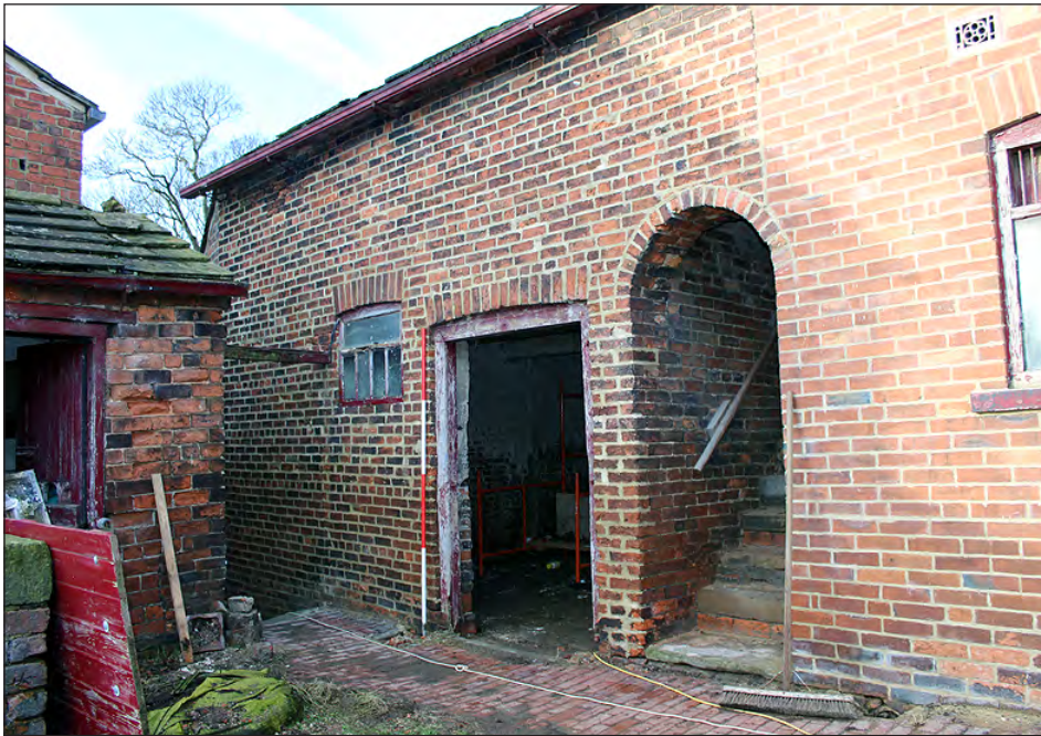
Plate 40. Building 4. South elevation. View looking northwest
