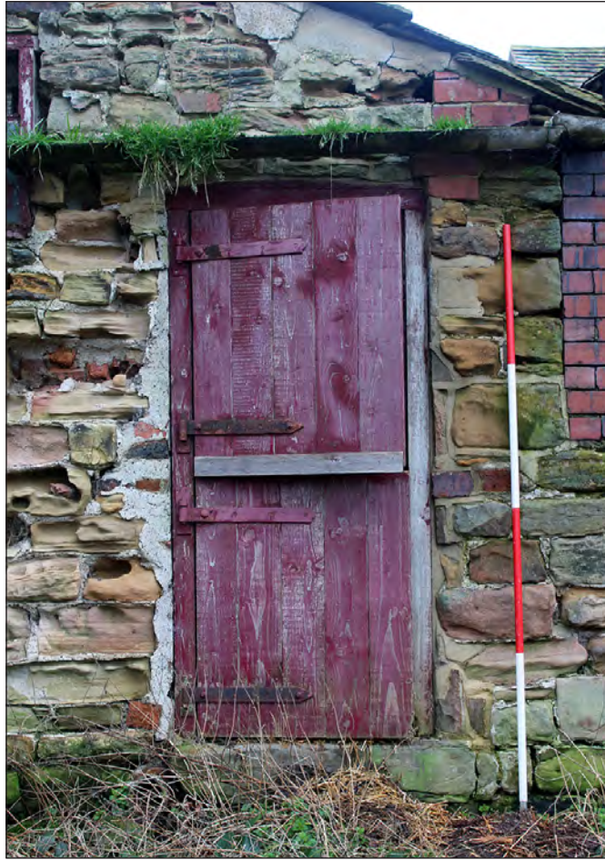
Plate 207. Building 10. South elevation doorway. View looking north-northwest
