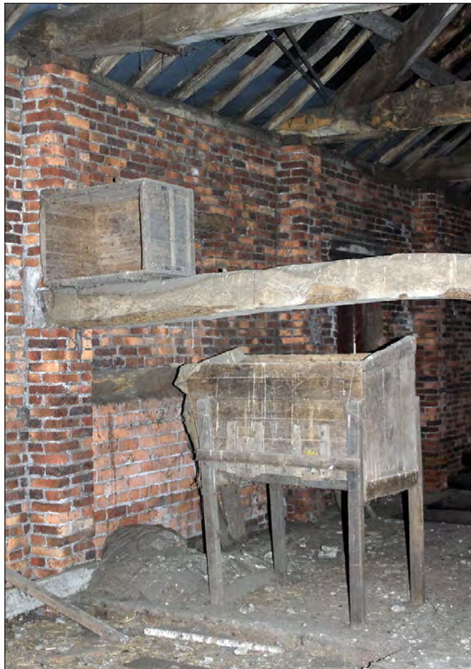
Plate 118. Building 5. Possible quail house or adapted hutch. View looking southwest
