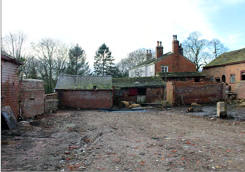
Plate 233. General view of the yard. View looking west-southwest
