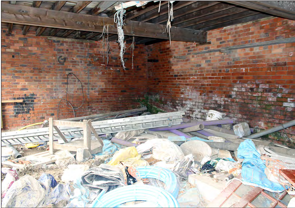
Plate 25. Building 3, interior. Ground floor. View looking northwest
