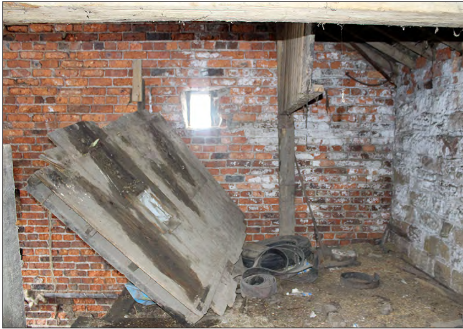
Plate 135. Building 6, interior. East elevation at mezzanine level. View looking east-northeast
