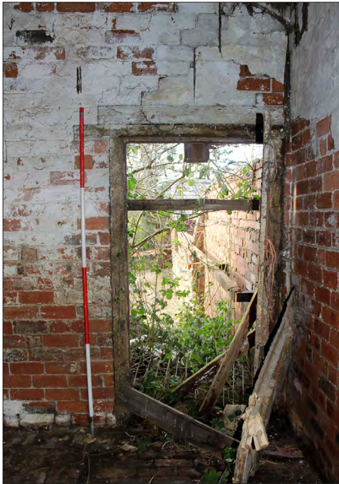
Plate 179. Building 8, interior. West elevation of the west side room, showing doorway. View looking west-southwest
