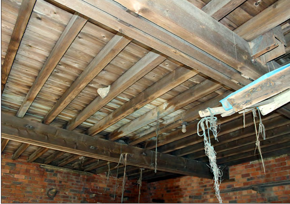
Plate 27. Building 3, interior. Ground floor ceiling. View looking northwest
